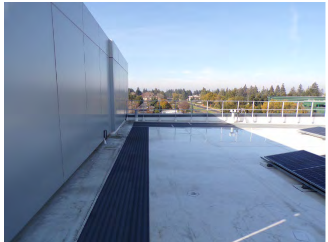
28. HVAC equipment screens are installed on the roof. They consist of aluminum composite panels on galvanized steel stud framing (at left).
