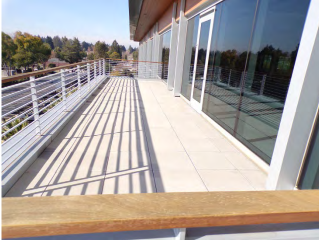
49. The balconies have a pedestal flooring system.
