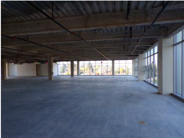
45. Third floor: Interior finishes in undeveloped shell of tenant lease area.
