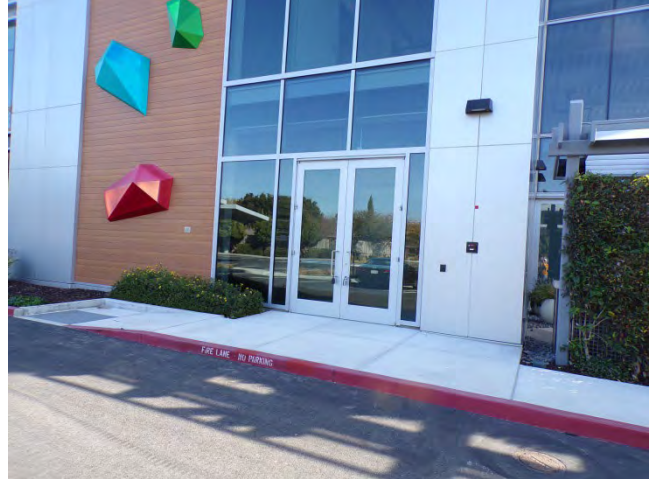
26. A secondary entrance is located along the west elevation.
