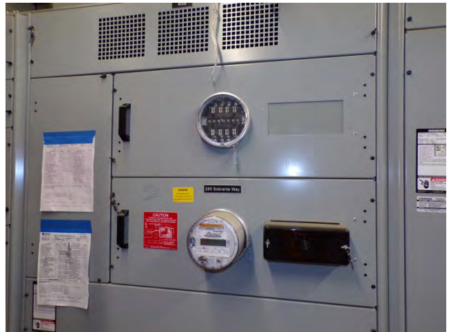
76. A Seimens 4,000 amp main service entrance panel is installed.
