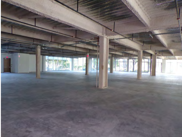
37. First floor: Interior finishes in undeveloped shell of tenant lease area.
