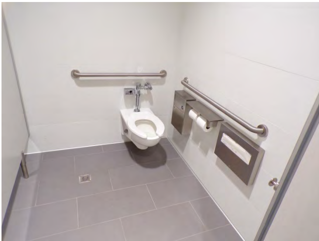
51. Interior finishes and fixtures in restrooms.
