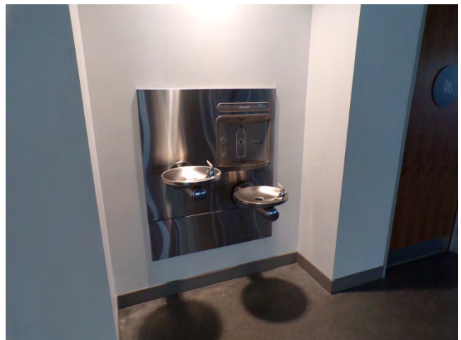
54. An Accessible high-low drinking fountain combination with bottle fill is provided on the first floor only.
