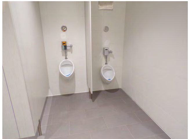
52. Interior finishes and fixtures in restrooms.
