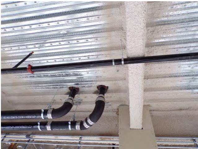
47. Fourth floor: Interior finishes in undeveloped shell of tenant lease area.
