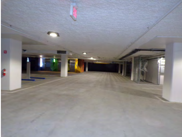
55. Basement: Interior finishes and fixtures.
