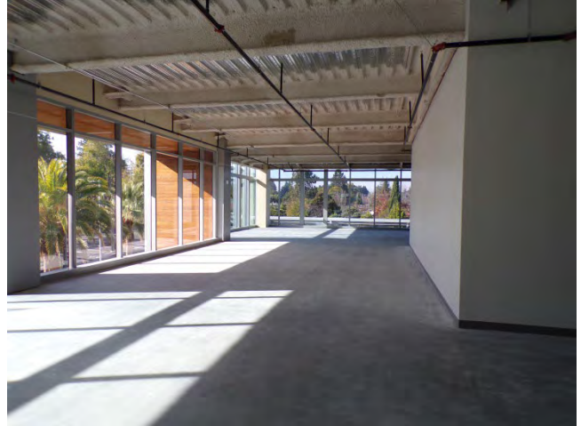
44. Second floor: Interior finishes in undeveloped shell of tenant lease area.
