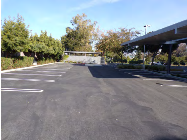
19. The asphalt-paved parking lot appeared in "Excellent" condition.
