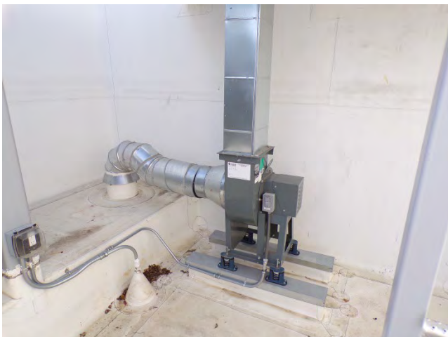
71. A Greenheck exhaust fan serves the electrical service room.
