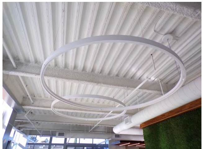
42. First floor: Interior finishes and fixtures in reception/seating area.
