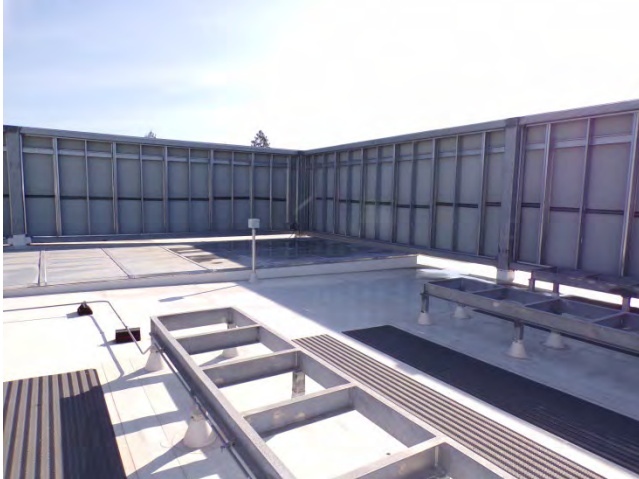
31. The roofing system appeared in "Good" condition.
