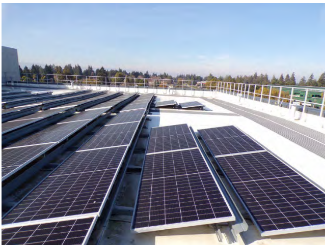
29. The solar panels cover much of the roof area.
