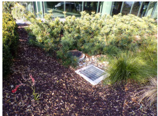
18. Numerous drain inlets are found in landscaped areas and in the parking lot.
