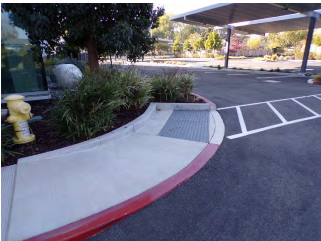
11. Truncated domes are installed in required locations.
