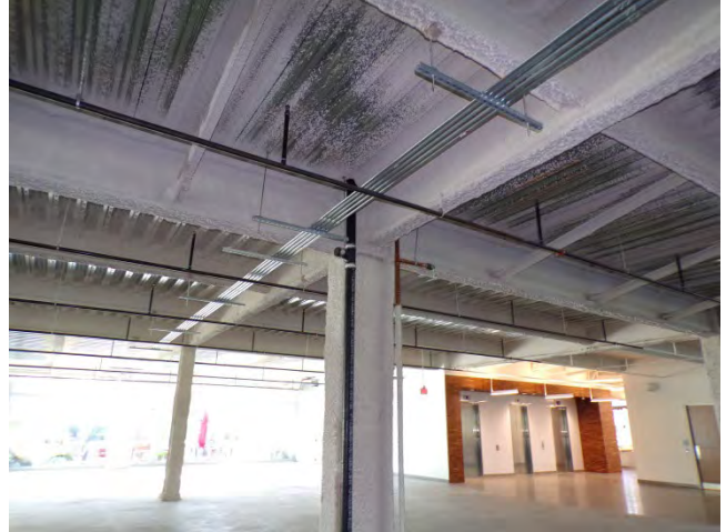
38. First floor: Interior finishes in undeveloped shell of tenant lease area. Elevator bank in background at right.
