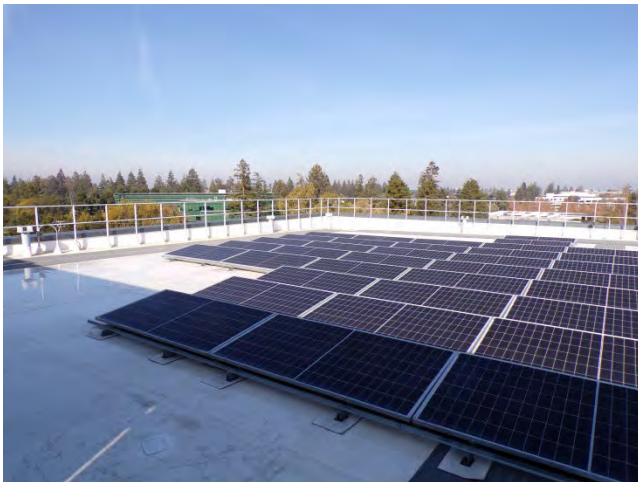
27. The TPO roofing system has a 60 mil membrane manufactured by Johns-Manville .
