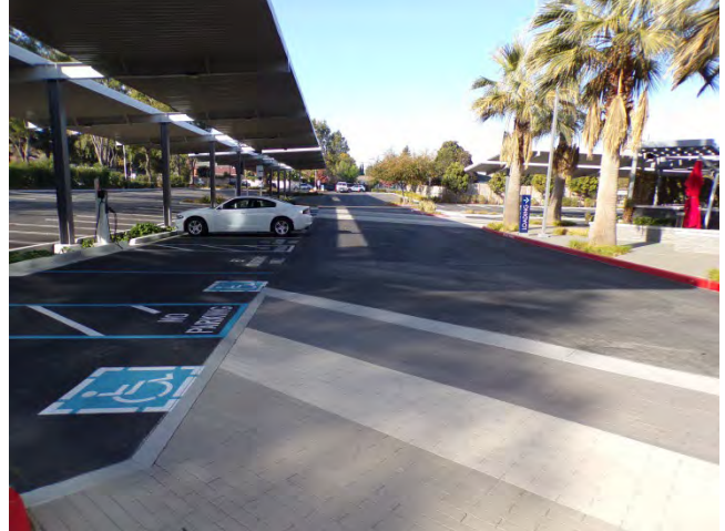
20. Concrete pavers resembling bricks in size can be seen in the foreground.
