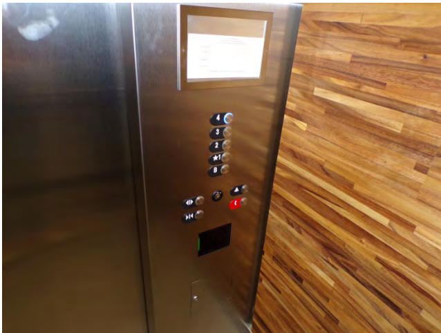
63. Interior finishes and control panel in elevator cars.
