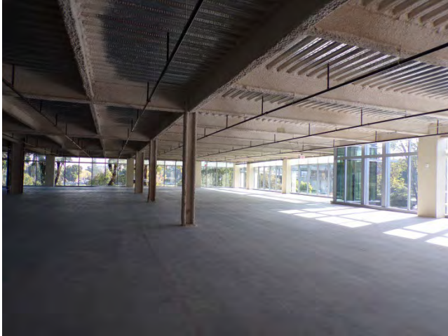
43. Second floor: Interior finishes in undeveloped shell of tenant lease area.
