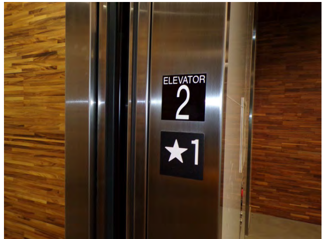
64. The elevators are evaluated in "Excellent" condition for Accessibility conformance.
