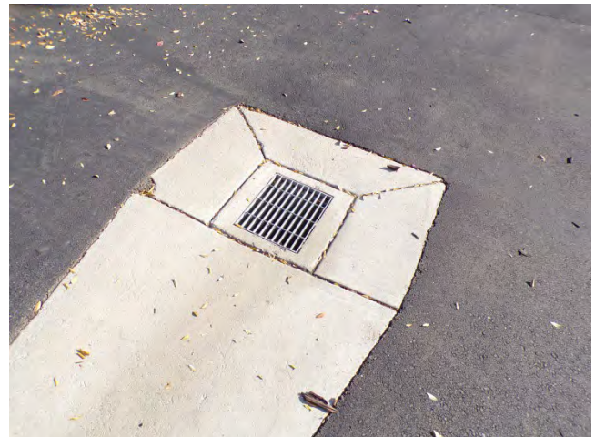
84. Drain inlets are located in several locations in the parking lot.
