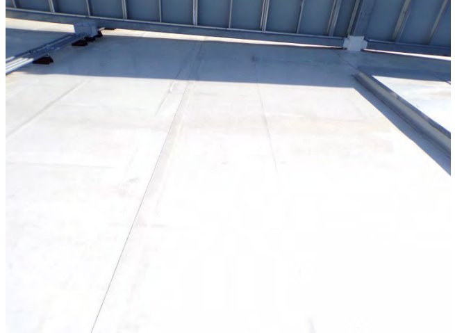
32. The roofing system has a 20-year NDL warranty.
