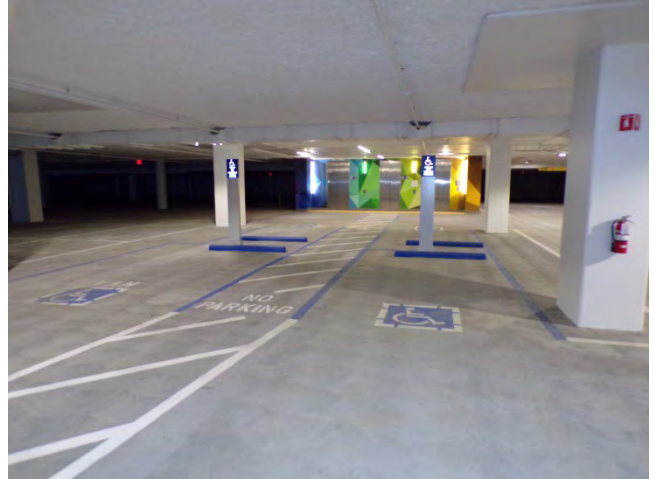
56. Basement: Interior finishes and fixtures. Four Accessible parking stalls are located in the basement.
