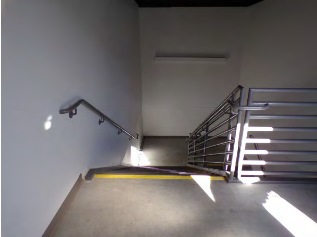
67. The fire stairs are steel-framed with cast-in-place concrete treads.
