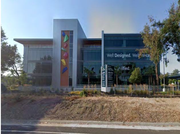
1. North elevation along Central Expressway.
