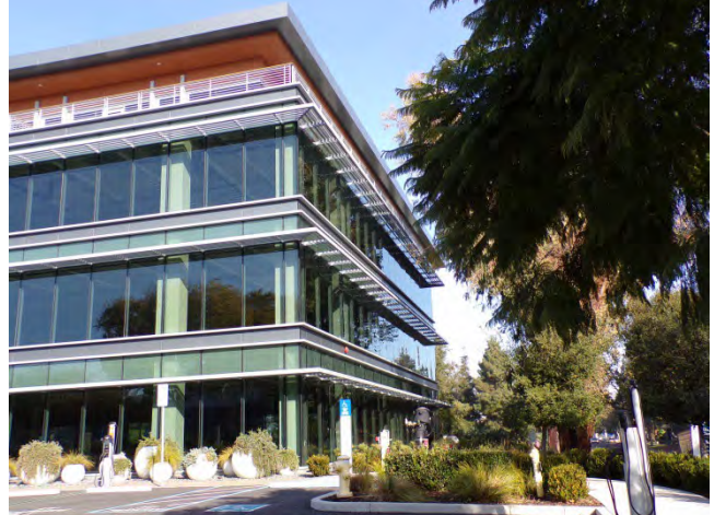
2. East elevation at right—portion of south elevation at left.
