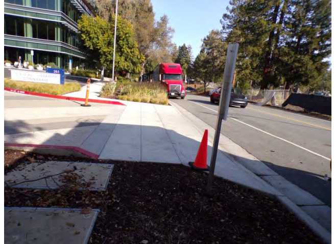
8. Sobrante Way curb cut, looking north.
