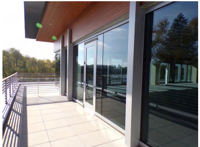
48. Balconies are installed on the fourth floor.
