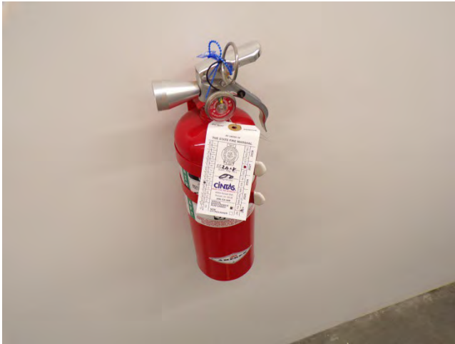
81. All observed fire extinguisher inspection tags were current.
