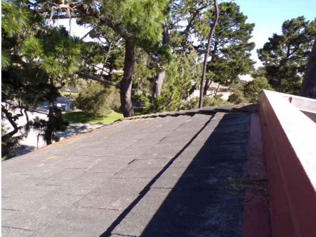
37. The concrete tile roof likely dates to original construction.
