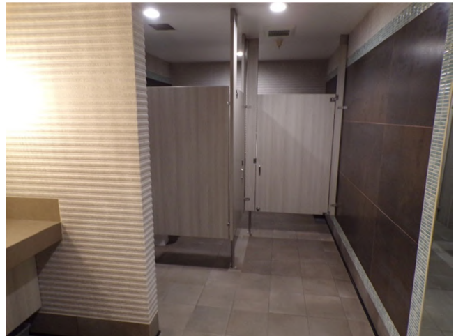
58. Interior finishes and fixtures in restrooms.
