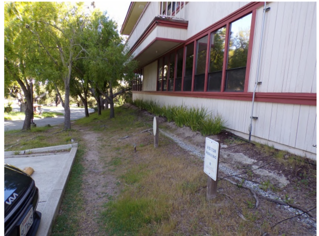
22. Purposefully planted vegetation immediately adjacent to the building is minimal.
