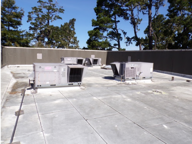
31. West wing: A BUR roofing system is installed.
