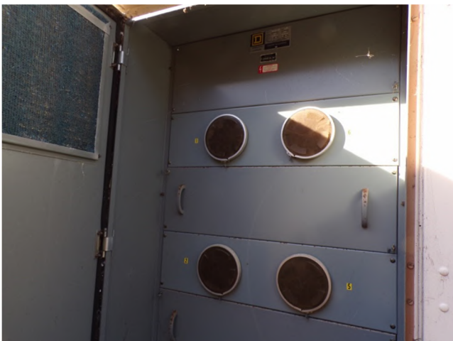
71. Four meter blanks are provided.
