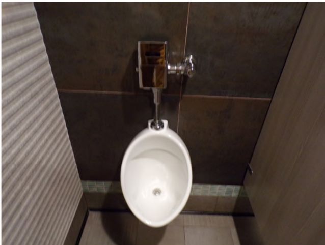
57. Interior finishes and fixtures in restrooms.
