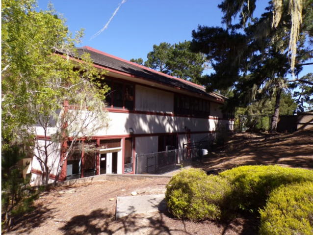
7. South elevation of east wing.
