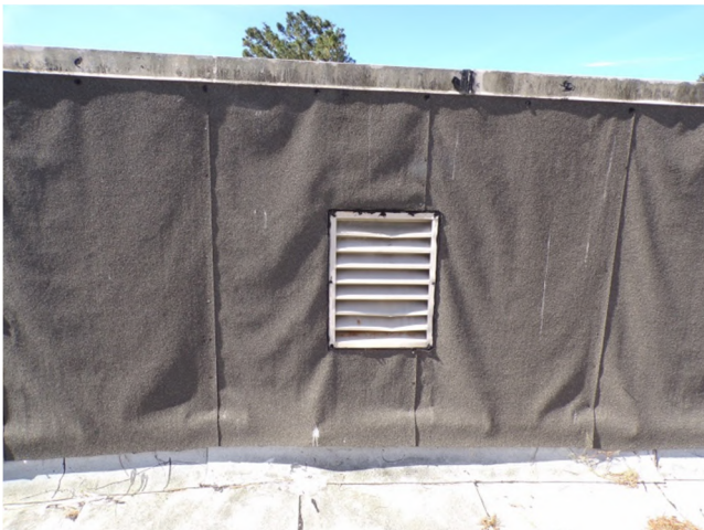
29. Both wings: A gray mineral granule cap sheet is applied to the inside face of the parapets. East wing shown.
