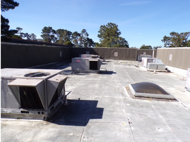
25. East wing: A BUR roofing system is installed.
