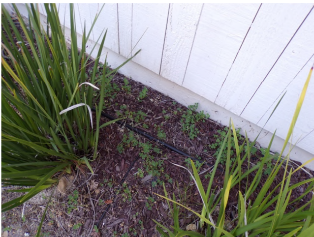
23. The irrigation system is only installed in proximity to the building perimeter. The grassy areas are typically unserved by the irrigation system.
