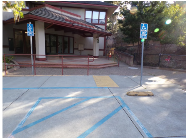
100. Truncated domes are located in only one required location near the Accessible parking stalls.
