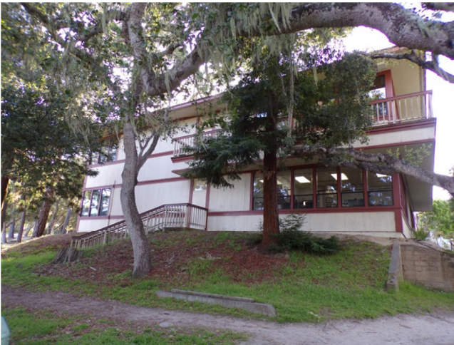
3. North elevation of west wing.
