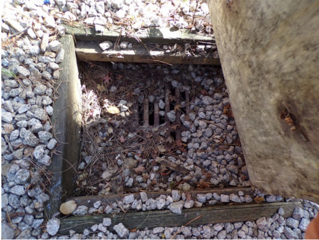
103. An area drain near the main building entrance is be fitted with a temprary plwood cover.
