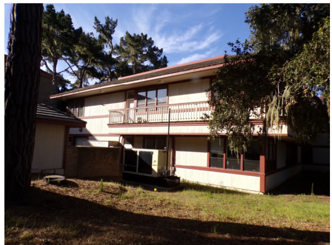
6. East elevation of east wing.
