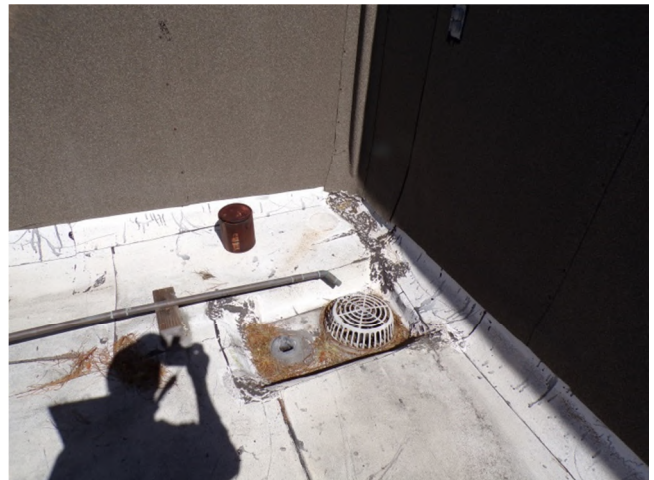
30. Both wings: The roof and overflow drains are located in shallow sumps. West wing shown.
