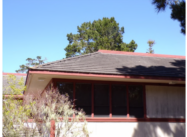
38. Most of our observations of the concrete tile roof were conducted from grade.
