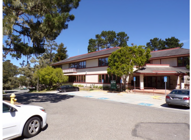
2. West elevation of west wing. This is the primary elevation facing the parking lot.
