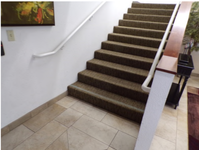
53. Interior finishes at stairs near main lobby.
