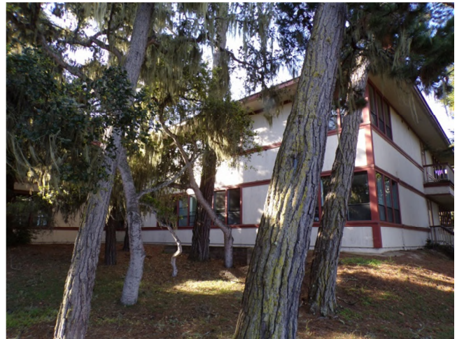
4. East elevation of west wing.
