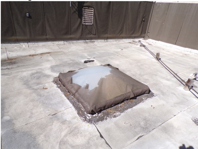
35. Four skylights are installed; two on each wing. East wing shown.
