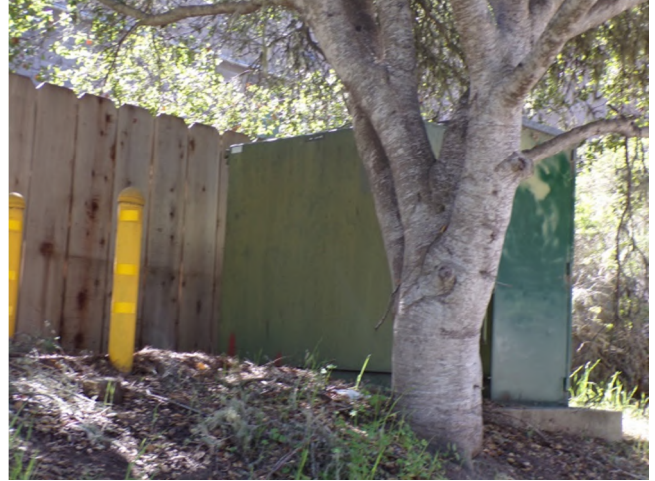
104. Electrical service is likely supplied from the adjacent parcel to the south.
