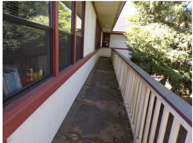
94. Two L-shaped balconies are provided.
