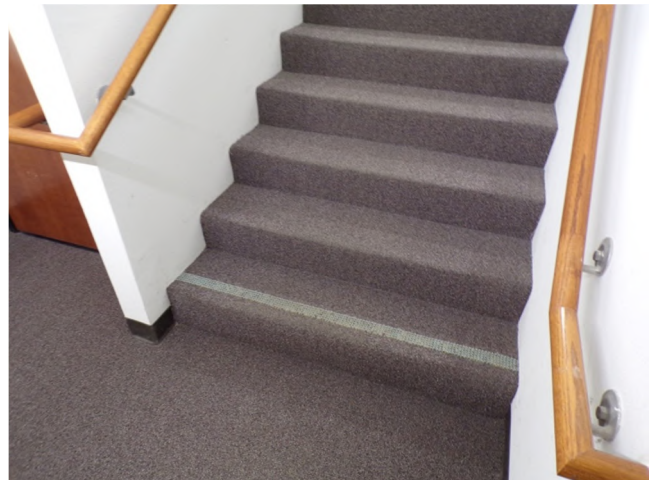
54. Interior finishes at secondary stairs.
