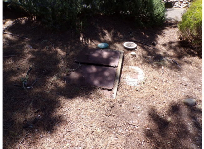
74. Water utility service is likely supplied from the adjacent parcel to the south.
