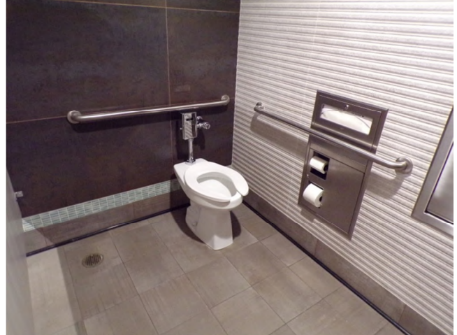
56. Interior finishes and fixtures in restrooms.
