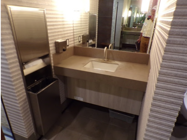
55. Interior finishes and fixtures in restrooms. The same finishes and fixtures are used in all four restrooms.
