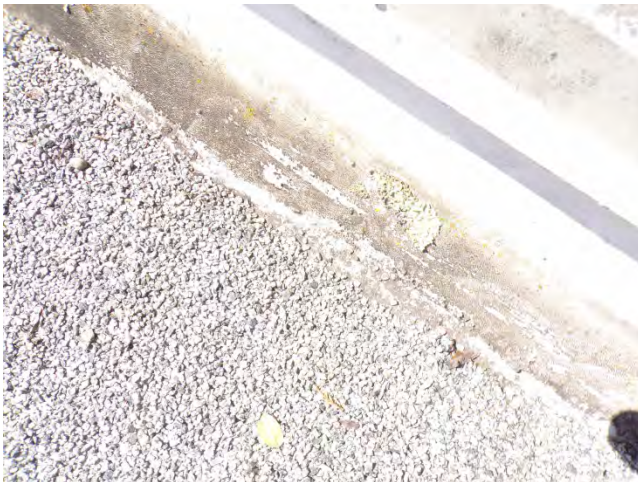
21. The roofing system appears to be a single-ply TPO membrane topped with ballast.
