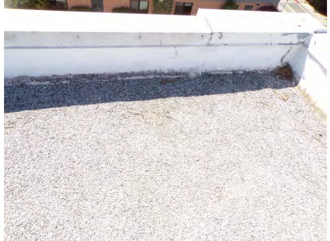
20. Granite pea ballast is broadcast over the underlying roofing membrane.
