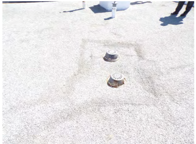
22. In the ballasted areas, roof and overflow drain combinations are installed within shallow sumps.
