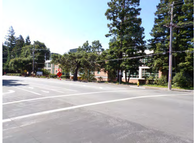
2. North elevation along Middlefield Road.
