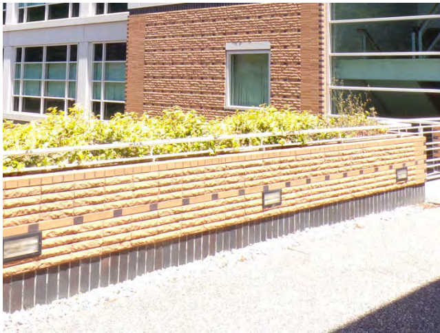
15. Landscaping at second floor level along walkway leading to main office/lab area entrance.
