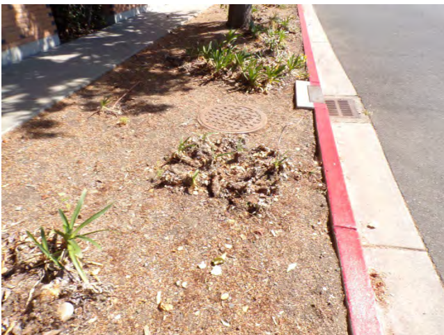
11. Plants in a degraded condition were observed in several locations.
