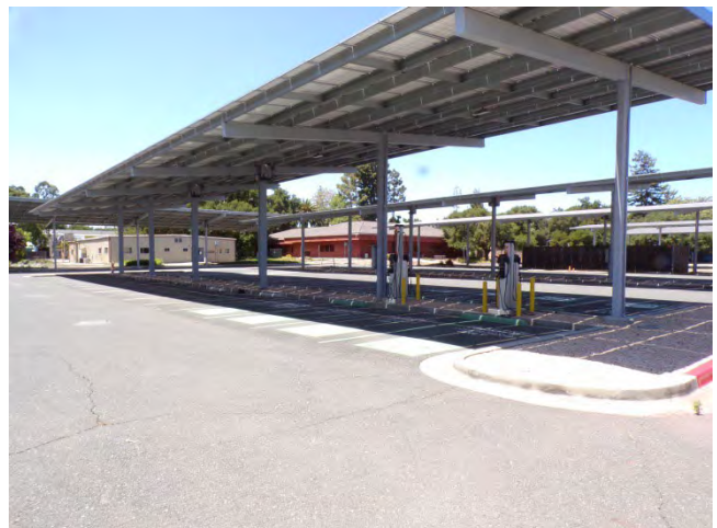
30. Canopies topped with solar arrays are installed in the main parking lot. The canopies/solar arrays are outside the scope of work for this project.
