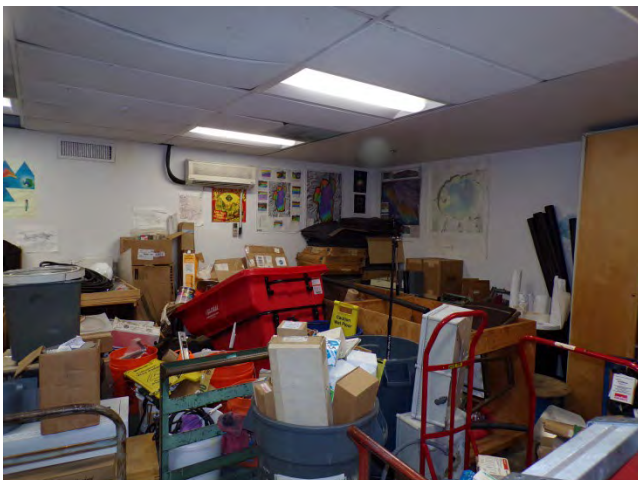
41. Interior finishes and fixtures in storeroom.
