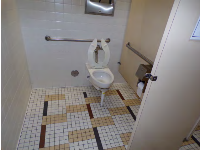
43. Interior finishes and fixtures in restrooms.
