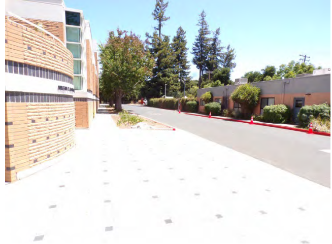
8. Survey Lane sidewalk, looking east-northeast.
