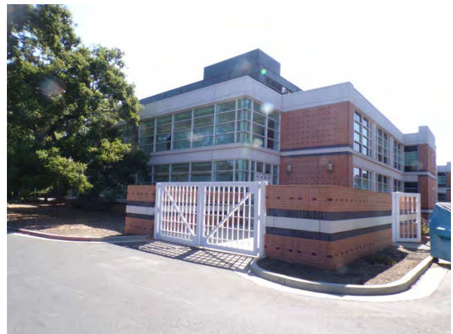
18. The loading dock area is located at the southwest corner of the building.
