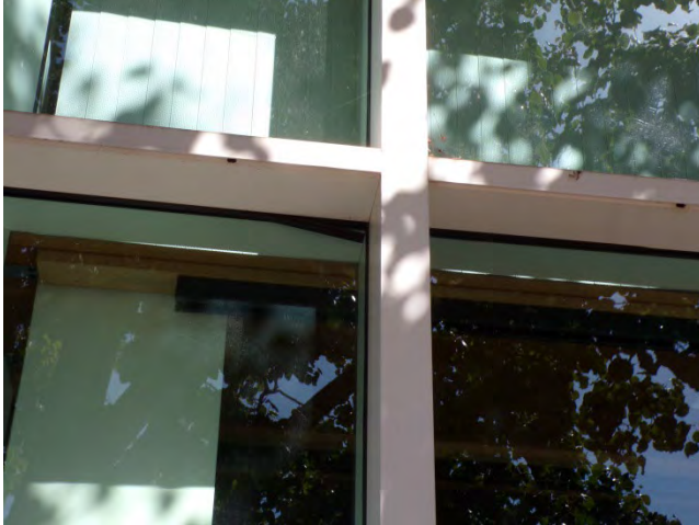
49. Drooping rubber window seal.
