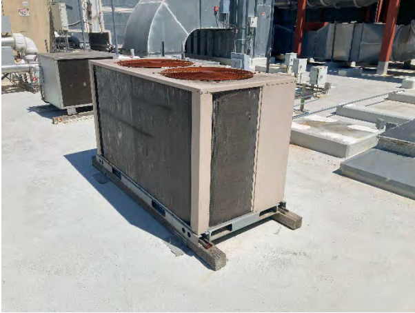
M-7. Supplemental packaged air conditioner.
