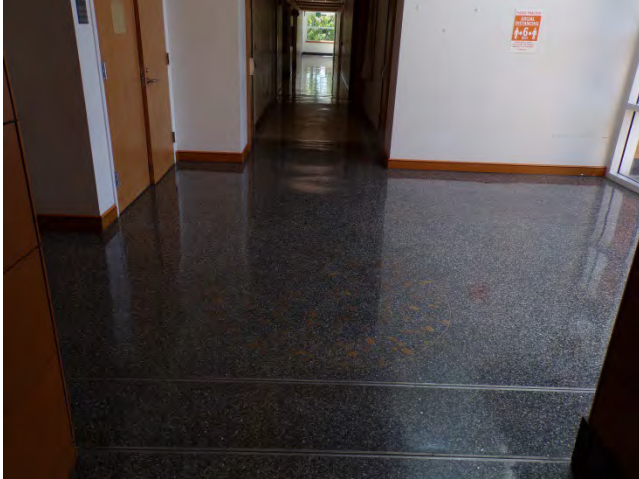
31. Interior finishes in lobbies and some corridor areas.
