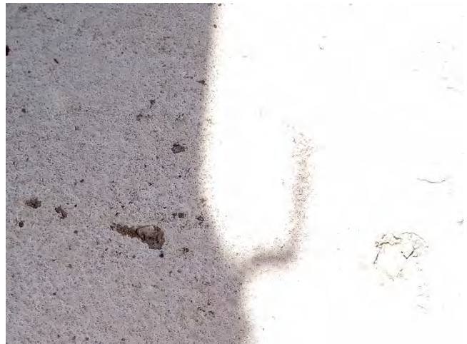
28. A coating has been applied on the roofing membrane within the screened areas.
