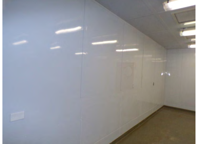
38. Interior finishes and fixtures in lab areas.
