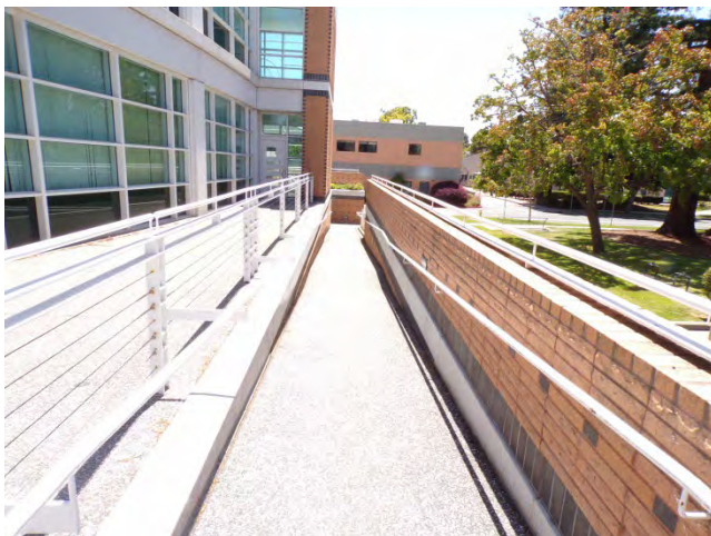
17. Concrete ramp along south elevation.
