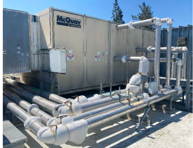
M-2. Four-pipe air handling unit.
