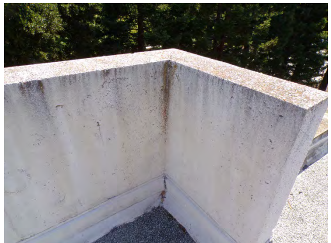
24. The precast concrete panels are also used for the parapets.
