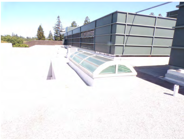
23. Seven skylights are installed.
