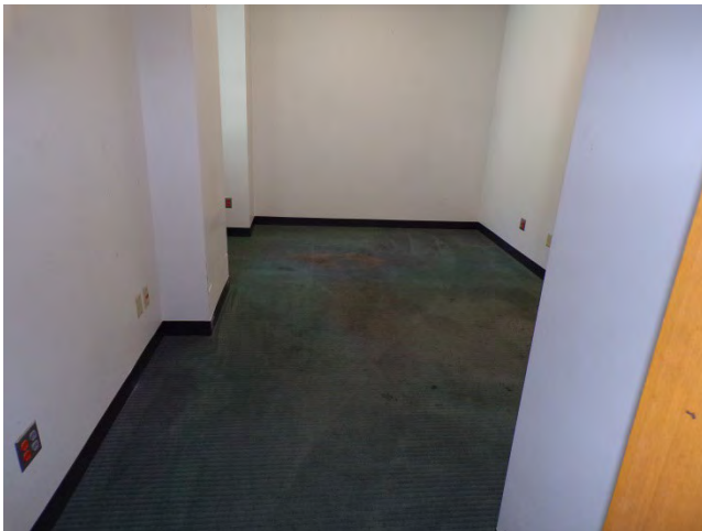
39. Interior finishes in office areas.
