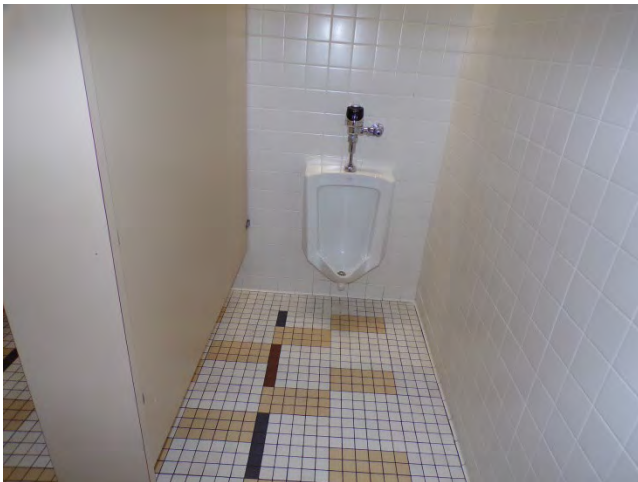
45. Interior finishes and fixtures in restrooms.
