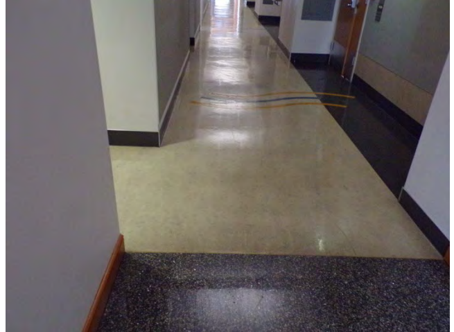
32. Interior finishes in corridor areas.
