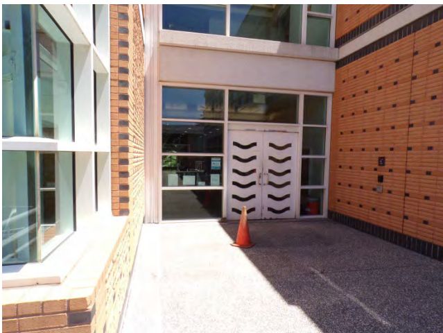
5. Main entrance on second floor level to offices and labs.
