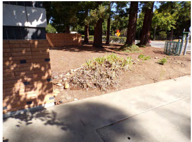
10. Plants in a degraded condition were observed in several locations.
