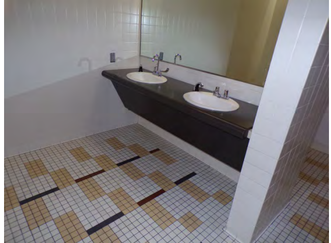
44. Interior finishes and fixtures in restrooms.
