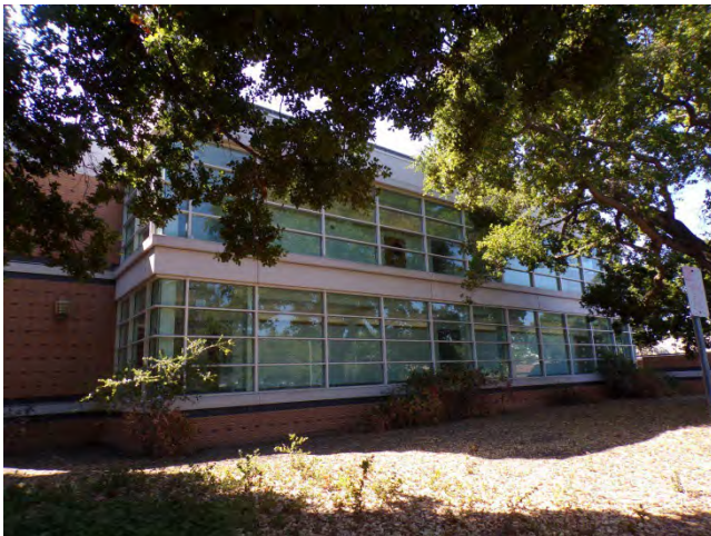
3. Portion of west elevation.
