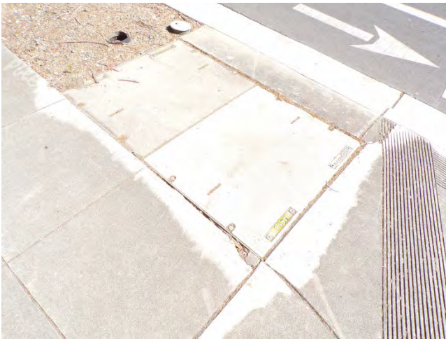
9. Evidence of past concrete grinding was observed.
