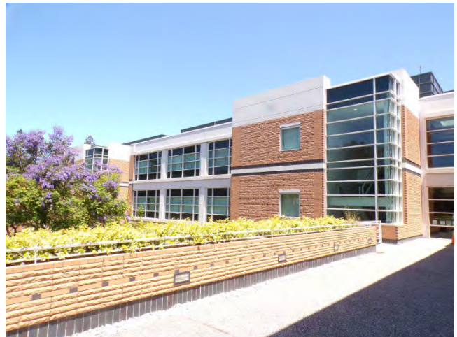
4. Portion of south elevation.
