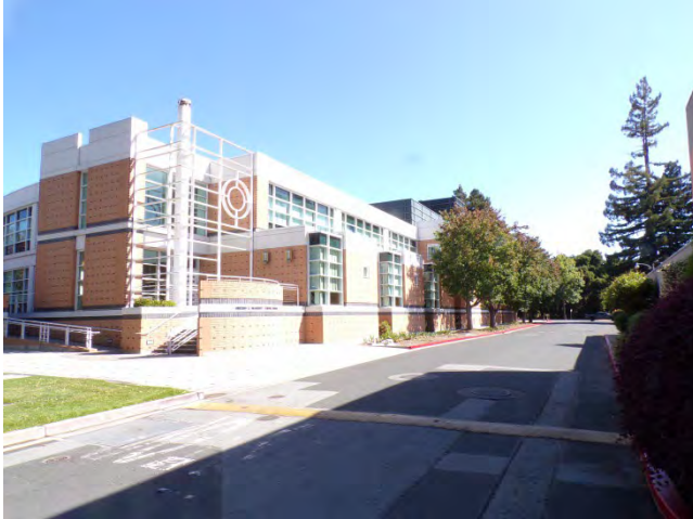
1. Southeast corner of Bldg 15 with east elevation at center. Survey Lane shown to the right of the building.
