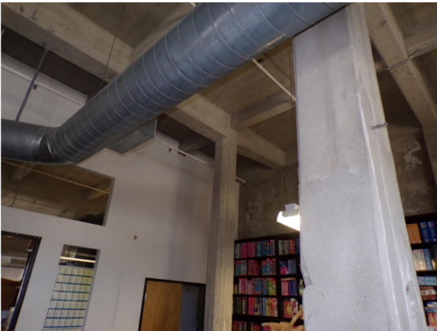
81. Fourth floor: Interior finishes and fixtures in private office.
