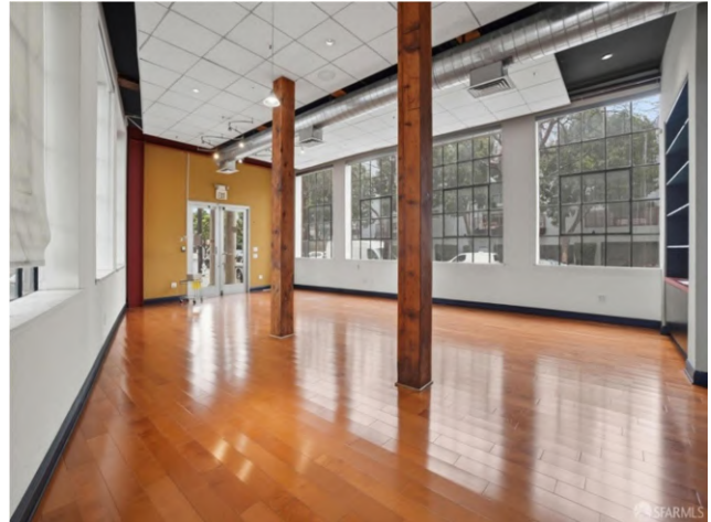
68. First floor: Interior finishes and fixtures in large foyer at main entrance.
