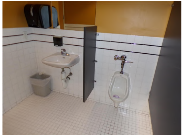
88. Interior finishes and fixtures in restrooms.
