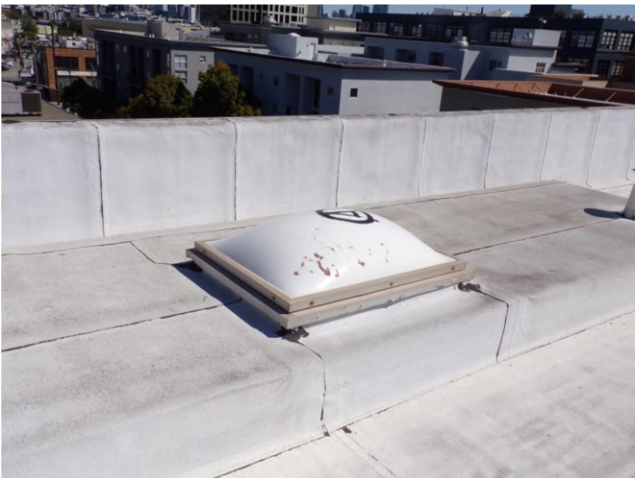
29. Fourth floor roof: Only one skylight is installed on this building.
