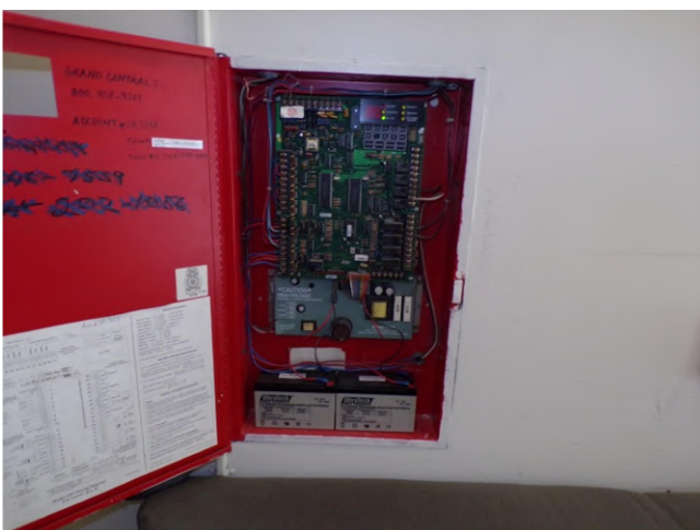
53. The FACP is a Silent Knight model 5207; it is out of production and obsolete.
