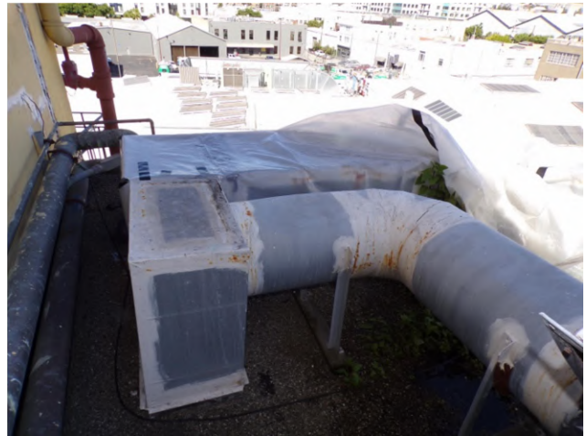
40. The age of the ventilation fan complex is unknown. Replacement is recommended.
