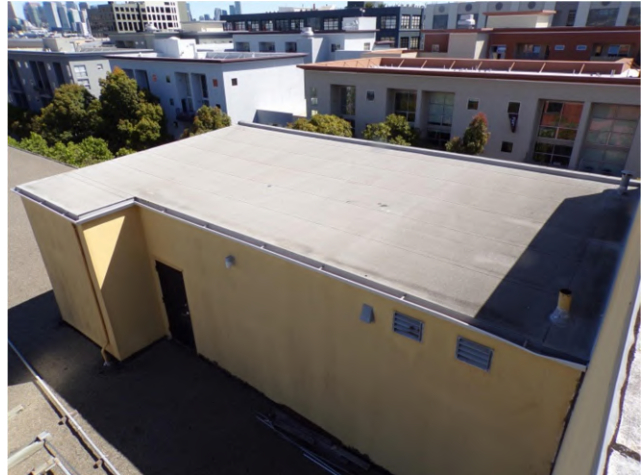
32. Penthouse: The BUR system on this roof level does not have gravel ballast.
