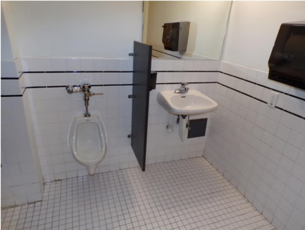
85. Interior finishes and fixtures in restrooms.
