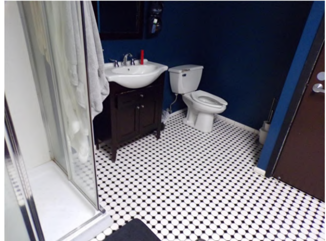
92. Interior finishes and fixtures in restrooms.
