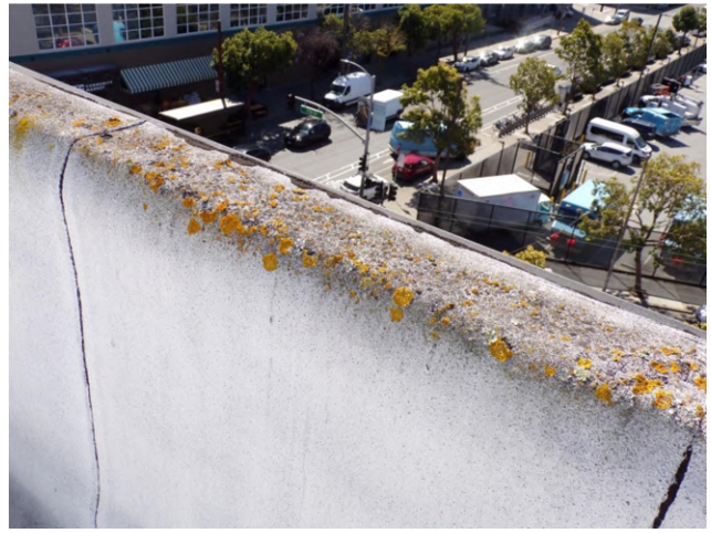
28. Fourth floor roof: The age of the roofing system is unknown; replacement is recommended.
