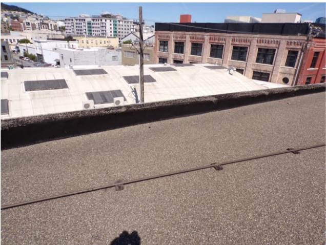
23. Main roof: Low parapets are provided.
