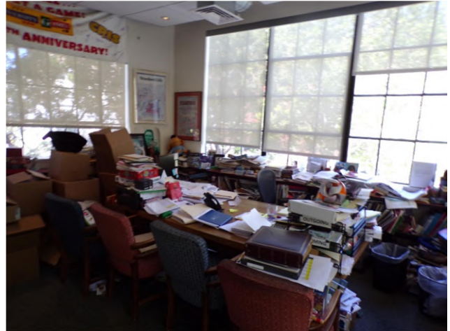
74. Second floor: Interior finishes and fixtures in private office.
