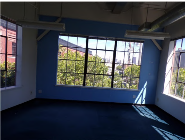
77. Third floor: Interior finishes and fixtures in private office.
