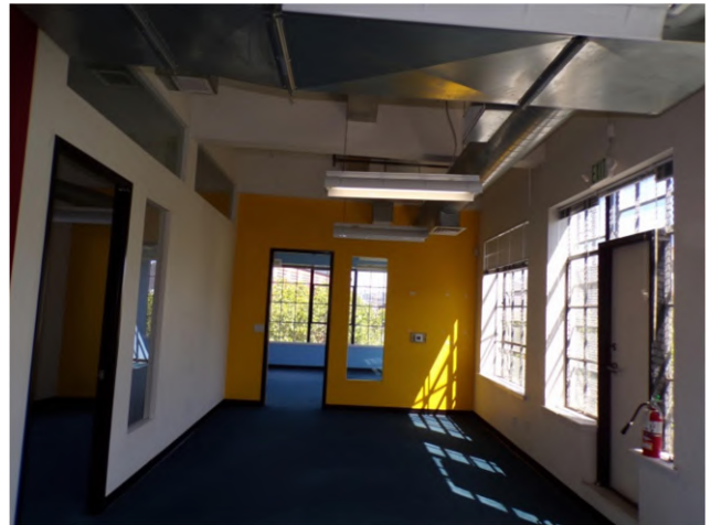
76. Third floor: Interior finishes and fixtures in private office.
