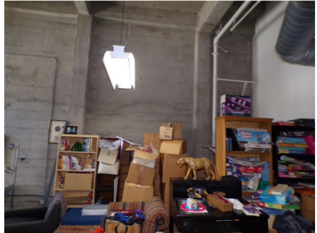
80. Fourth floor: Interior finishes and fixtures in private office.
