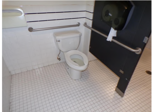
86. Interior finishes and fixtures in restrooms.
