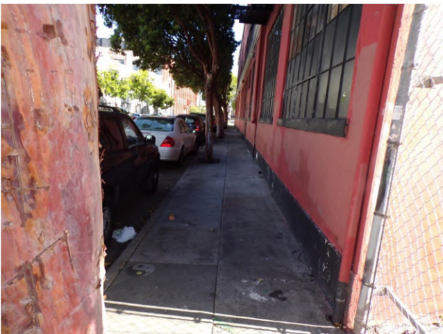
17. Public sidewalk along west elevation.
