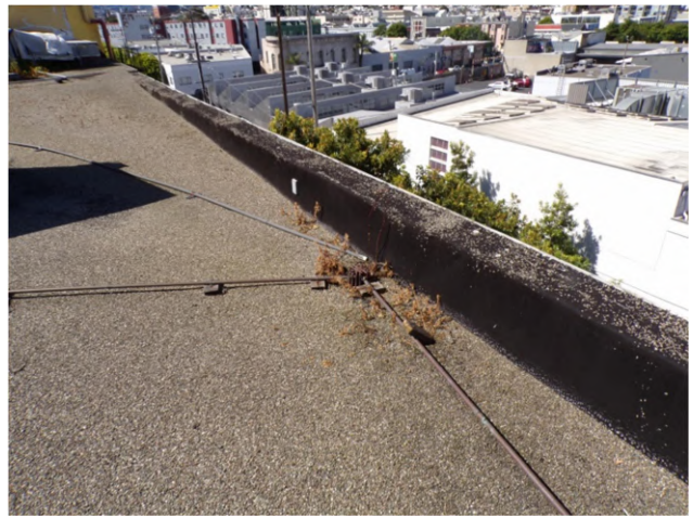
24. Main roof: Only one roof drain serves this level of the roof.
