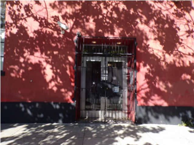
13. The secondary pedestrian entrance on the east elevation serves as an Accessible entrance. ISA signage is not provided at this entrance.
