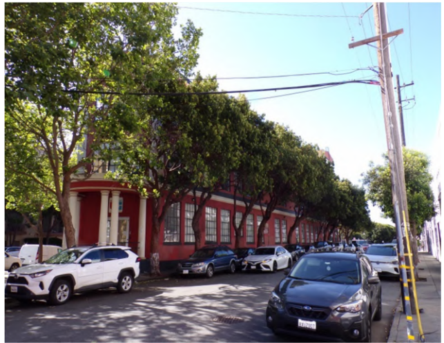
4. West elevation along Treat Avenue.
