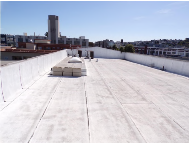
27. Fourth floor roof: The BUR system on this roof level does not have gravel ballast.
