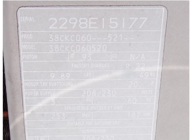
44. Both Carrier split systems were manufactured in 1998.
