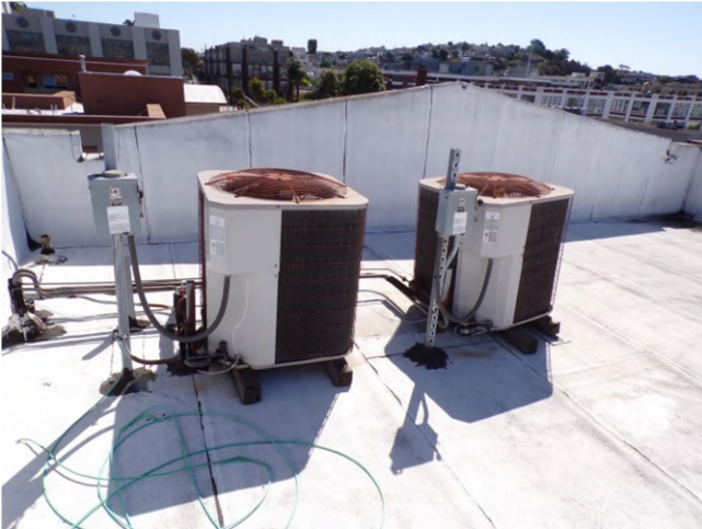
43. Two five ton Carrier splits systems are installed on the fourth floor roof.
