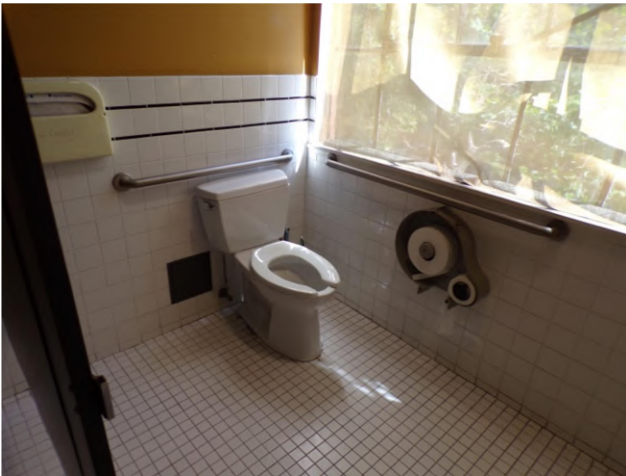
87. Interior finishes and fixtures in restrooms.
