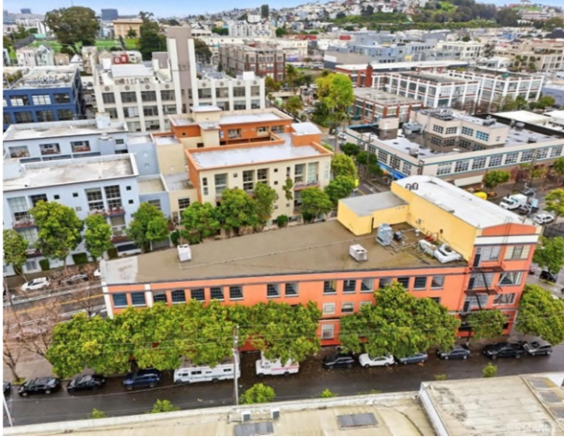
1. The building was constructed in 1907.
