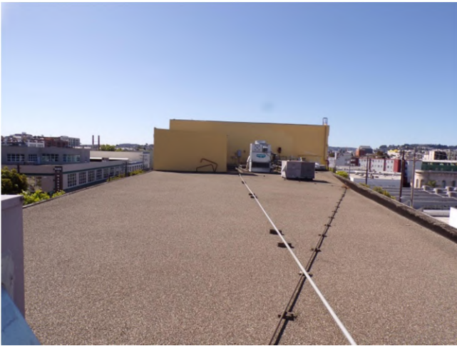
21. Main roof: The BUR system has pea gravel ballast.
