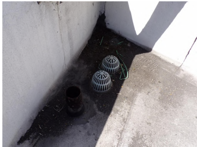
30. Fourth floor roof: A roof and overflow drain combination is provided.
