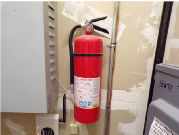
59. All observed fire extinguishers had expired tags or the tags were absent, as shown.
