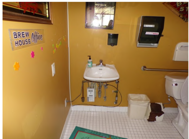
90. Interior finishes and fixtures in restrooms.
