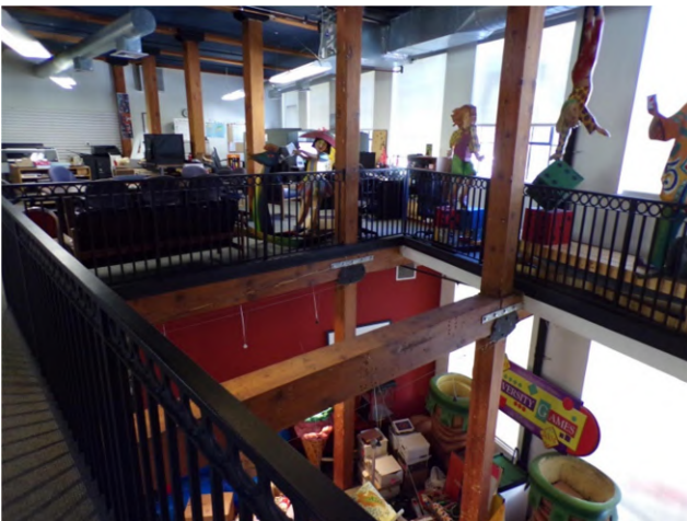
71. Second floor: Interior finishes and fixtures in open office area.
