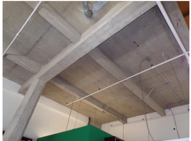
82. Fourth floor: Interior finishes in private office.
