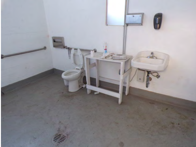
121. Bldg 5601E: Interior finishes and fixtures in restrooms. Unlike other restrooms, this one does not appear to have been upgraded for Accessibility compliance.
