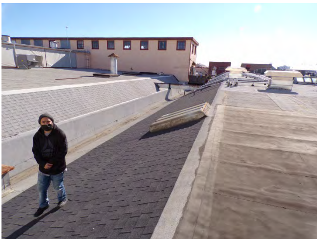
77. Bldg 5733W: Composite asphalt shingles are typically installed on the pitched roofs.
