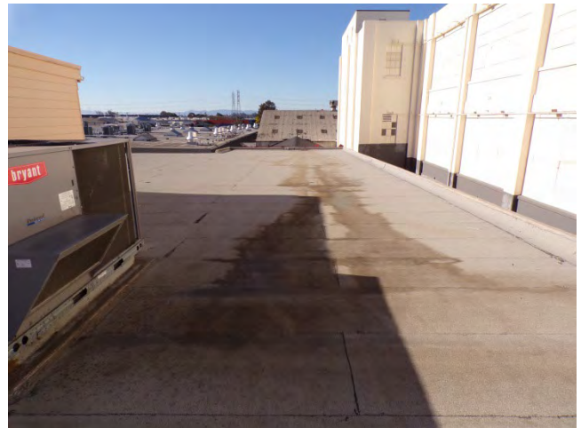
64. Bldg 5733E: The BUR roofing system on the north side of the building, looking west.
