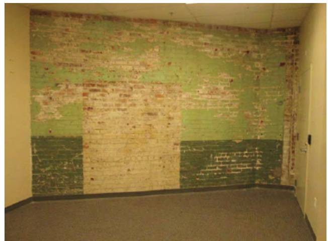
114. Bldg 5733W: Interior finishes in office areas. (Photo from 2017 PCA.)
