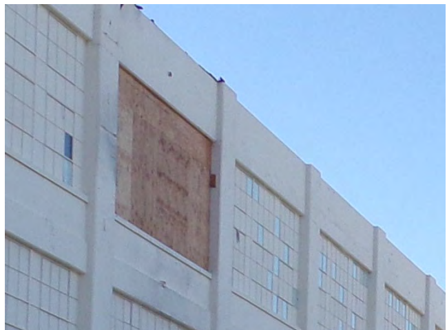
132. Bldg 5601E: One window bay on the third floor of the north elevation has been infilled with plywood.
