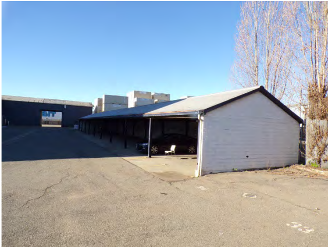
15. Bldg 5601E: Carport along north property line.
