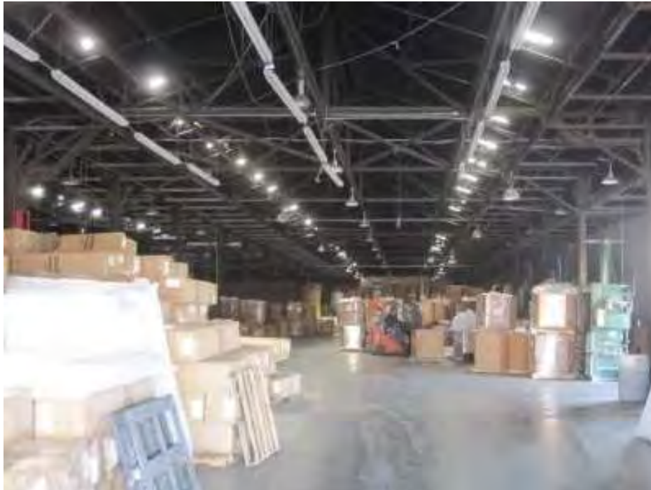
7. The warehouse open-web steel trusses and supporting columns.
