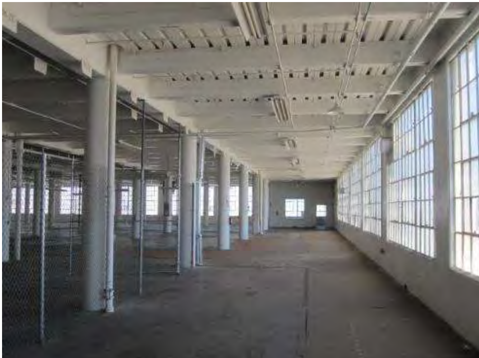
6. The corrugated metal decking, concrete slabs, joists, beams, columns and supporting exterior bearing walls in the main portion of the building.
