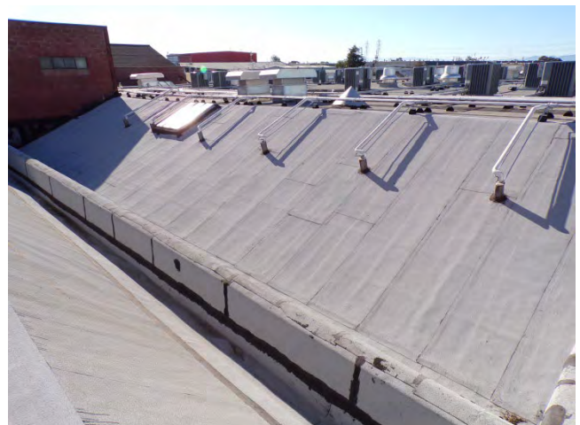
78. Bldg 5733W: BUR systems are also installed on some pitched roofs.
