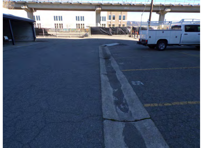
38. Bldg 5601E: Asphalt parking area on north side of building; concrete swale at center of photo.
