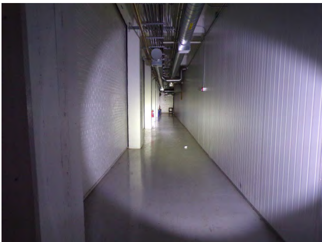
89. Bldg 5601E: Interior finishes and fixtures in circulation area of plant cultivation rooms.
