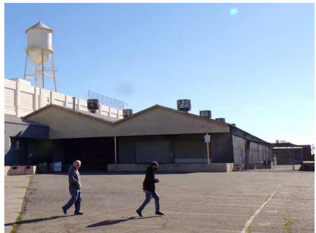
6. Bldg 5601W: North elevation at center of photo; west elevation at right.
