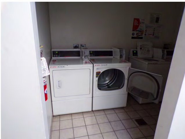
137. 5733E: Laundry room in apartment portion of building.
