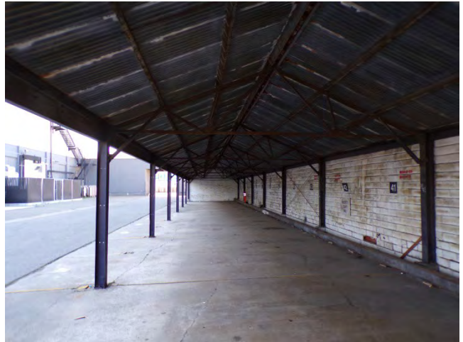
16. Bldg 5601E: Carport along north property line. Paint finishes in carport should be repainted during the reserve term.
