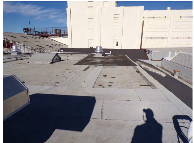
76. Bldg 5733W: The BUR roofing system on the east side of the building, looking north.
