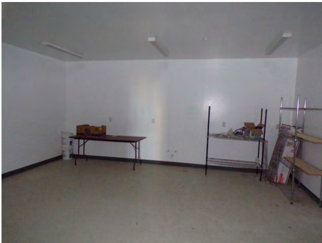
93. Bldg 5601W: Interior finishes and fixtures in office area.
