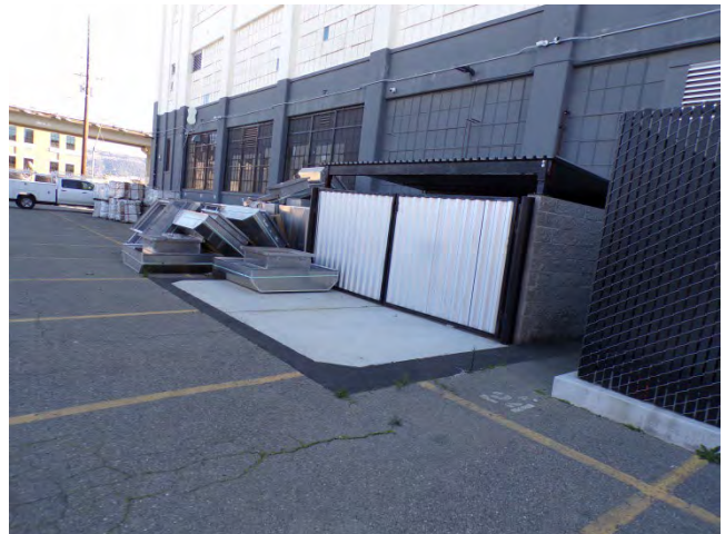
18. Bldg 5601E: A CMU trash enclosure was recently constructed.
