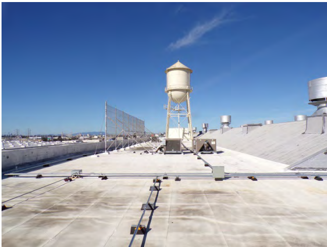
57. Bldg 5601E: The water tower is no longer in service.
