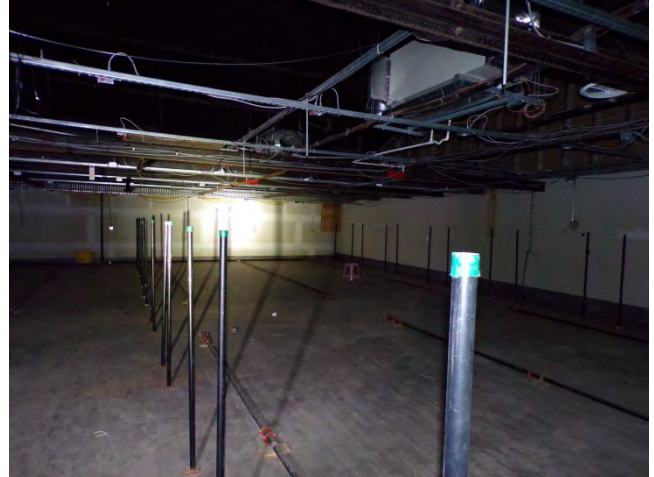
98. Bldg 5601W: Interior finishes, fixtures and equipment in attic room.
