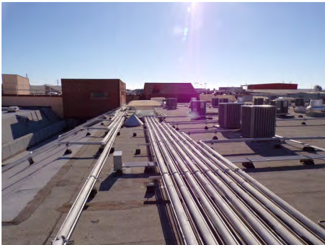
75. Bldg 5733W: The BUR roofing system on the east side of the building, looking south.
