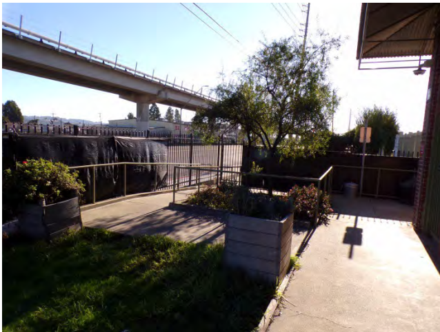
33. Bldg 5733E: Landscaping at the property is minimal.
