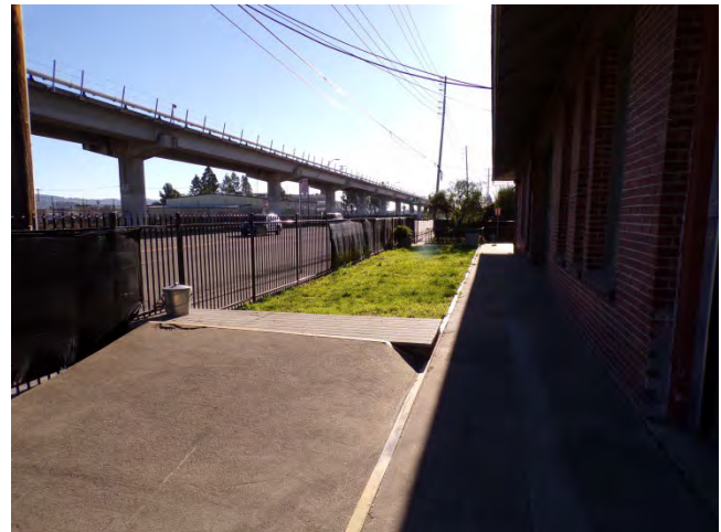
34. Bldg 5733E: Landscaping at the property is minimal.
