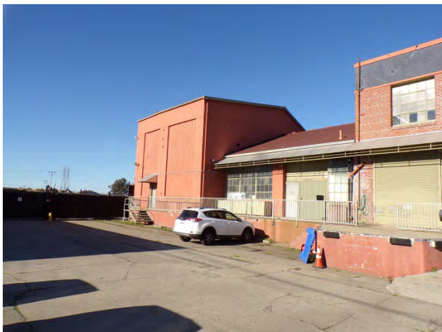
23. Bldg 5733E: South elevation, west portion.
