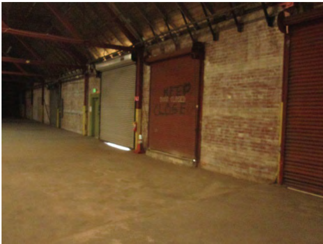
111. Bldg 5733E: Interior finishes in warehouse areas. (Photo from 2017 PCA.)
