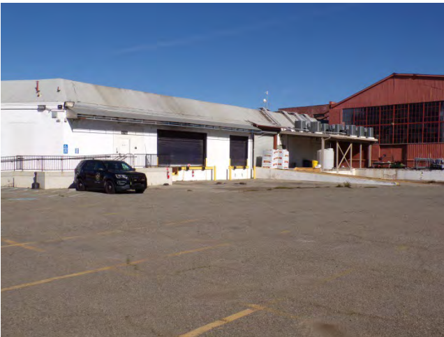
27. Bldg 5733W: South elevation.
