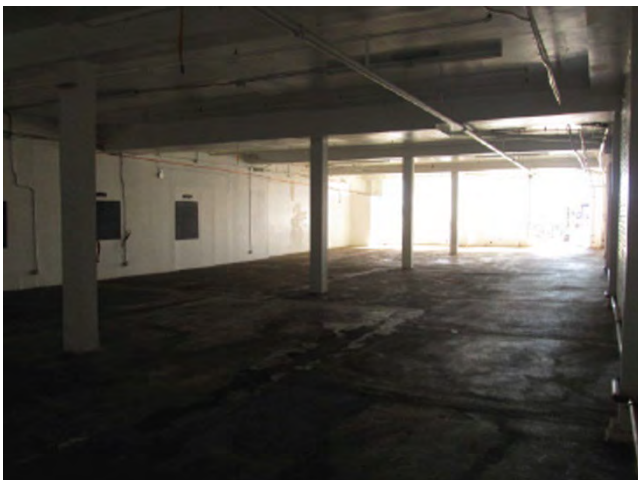
113. Bldg 5733W: Interior finishes and fixtures in warehouse areas. (Photo from 2017 PCA.)
