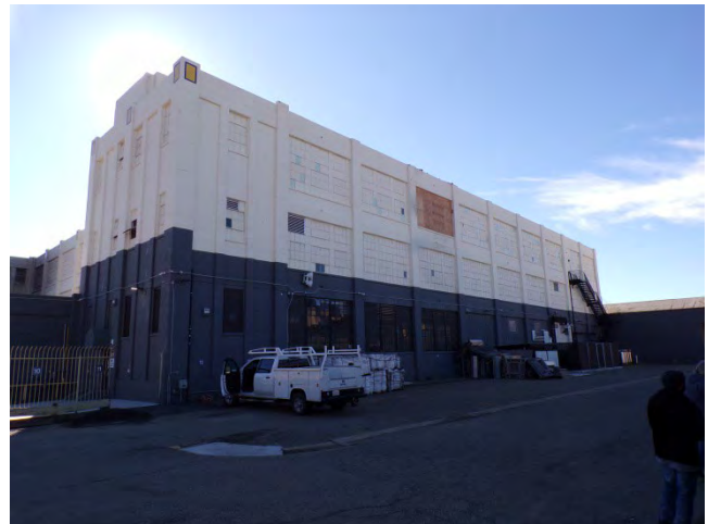
4. Bldg 5601E: North elevation.
