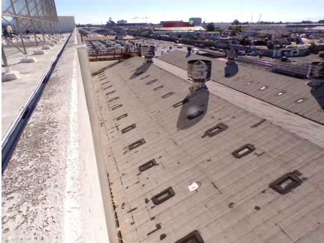
61. Bldg 5601W: The ribbed steel roof panels appear to have had a spray-on coating applied.
