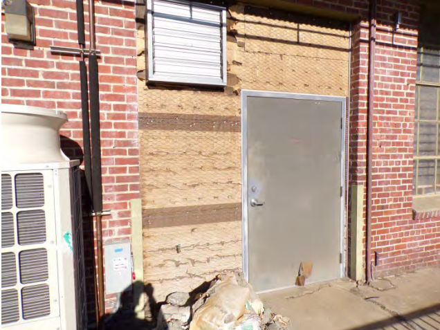
25. Bldg 5733E: Plywood has been installed in various locations along the south elevation.
