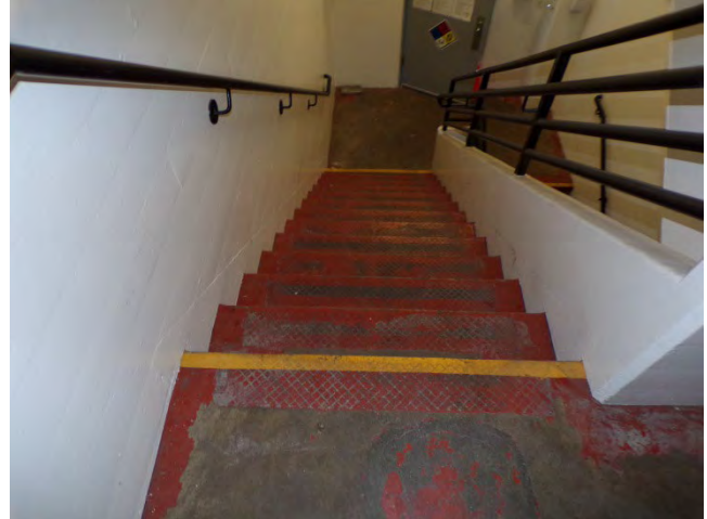
92. Space 5601E: Interior finishes in stairwells.
