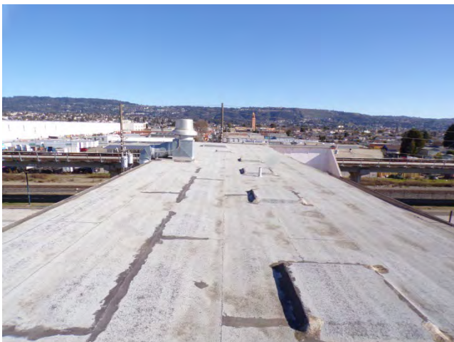
65. Bldg 5733E: The BUR roofing system on the second story portion of the building, looking east.
