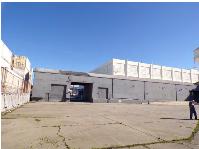
5. Bldg 5601W: West elevation. Bldg 5601E (white building) in background.
