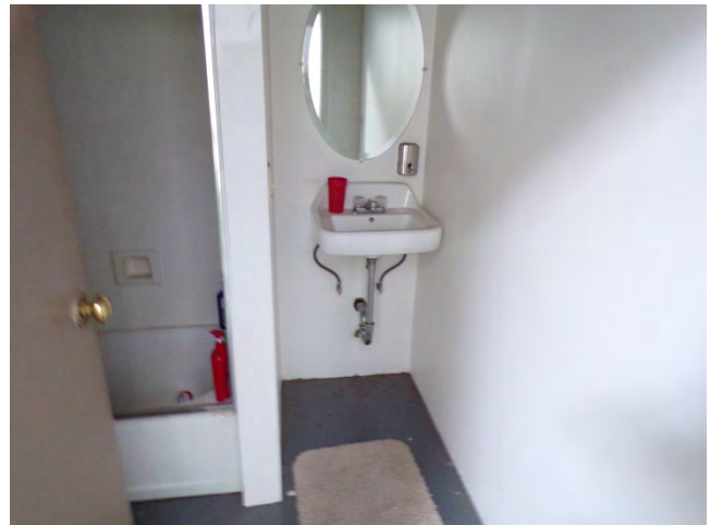
106. Bldg 5733E: Interior finishes and fixtures in apartment bathrooms.
