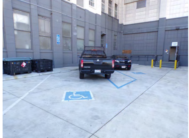
8. Bldg 5601E: New Accessible parking stalls along east elevation.
