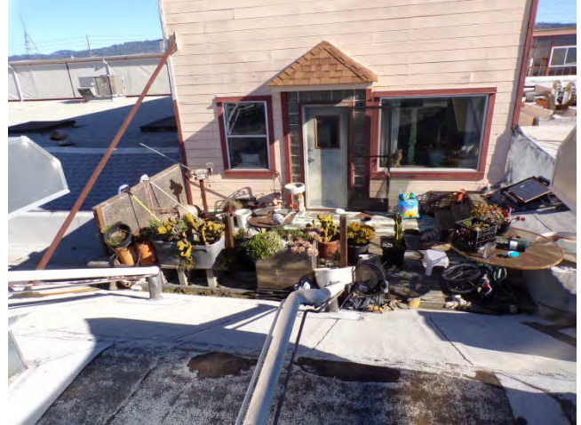
74. Bldg 5733E: A wood-framed roof terrace is installed on the west end of the two-story portion of this building.
