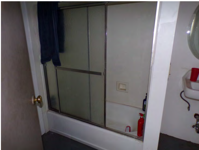
105. Bldg 5733E: Interior finishes and fixtures in apartment bathrooms.
