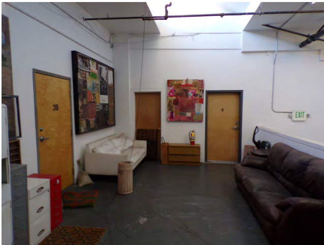
99. Bldg 5733E: Interior finishes and fixtures in common area of apartment portion of building.
