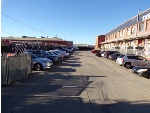
43. Bldg 5733E: Concrete-paved parking area on east side of site.
