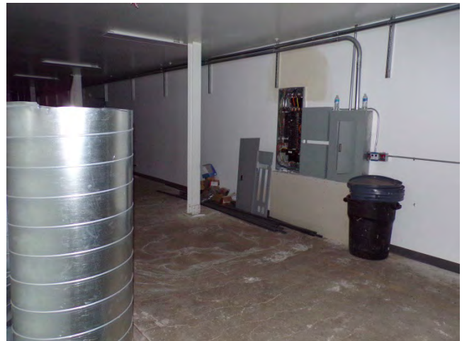
94. Bldg 5601W: Interior finishes, fixtures and equipment in circulation area of plant cultivation rooms.
