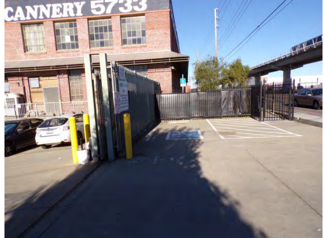
44. Bldg 5733E: One Van Accessible parking stall is provided at this building.
