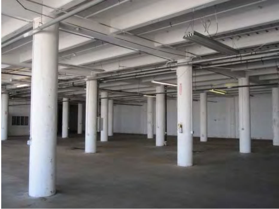
5. The reinforced concrete slabs, joists, beams and supporting columns in the main portion of the building.
