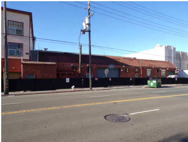
21. Bldg 5733E: East elevation, north portion.
