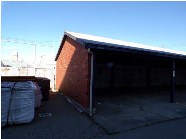
17. Bldg 5601E: Carport along north property line.
