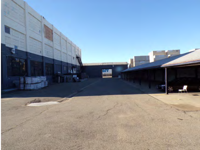
37. Bldg 5601E: Asphalt parking area on north side of building.
