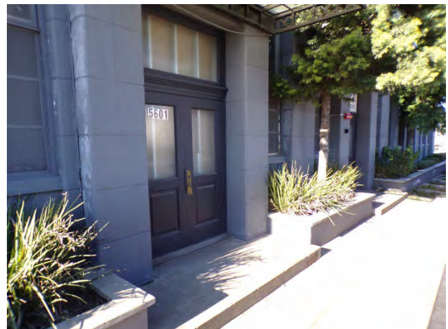
36. Bldg 5601E: Landscaping along east elevation.
