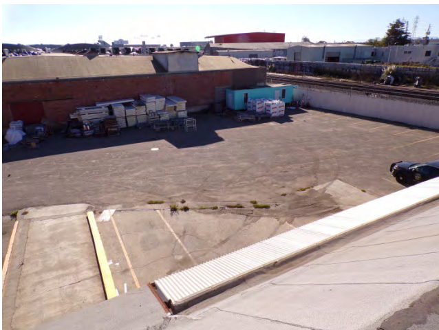
47. Bldg 5733W: Concrete and asphalt paving are provided on the south side of this building.
