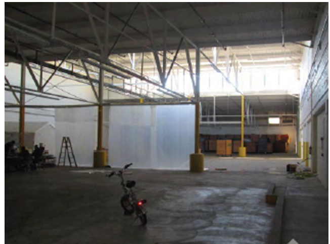
112. Bldg 5733W: Interior finishes and fixtures in warehouse areas. (Photo from 2017 PCA.)
