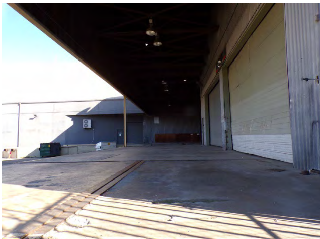
11. Bldg 5601W: Concrete loading apron on north elevation.
