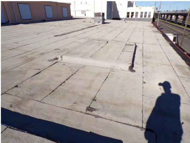
63. Bldg 5733E: The BUR roofing system on the east side of the building, looking north.
