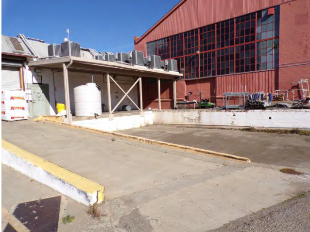
31. Bldg 5733W: Loading area with concrete truck ramp in foreground.
