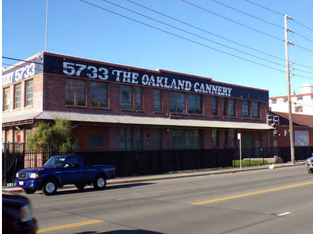
19. Bldg 5733E: East elevation, south portion.
