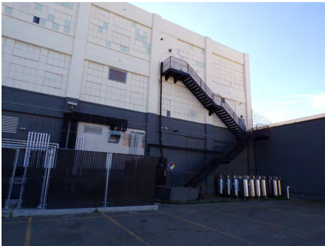
9. Bldg 5601E: Exterior stairs on north elevation.
