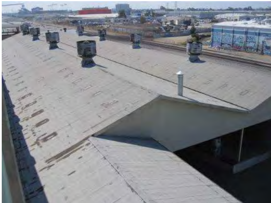
4. The single-story steel framed warehouse portion of the building.
