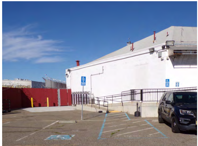
28. Bldg 5733W: Chamfered corner at southwest corner of building.
