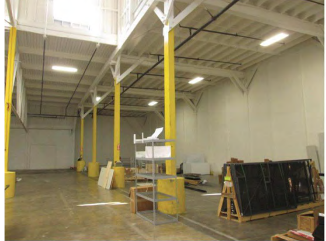
110. Bldg 5733E: Interior finishes and fixtures in warehouse areas. (Photo from 2017 PCA.)
