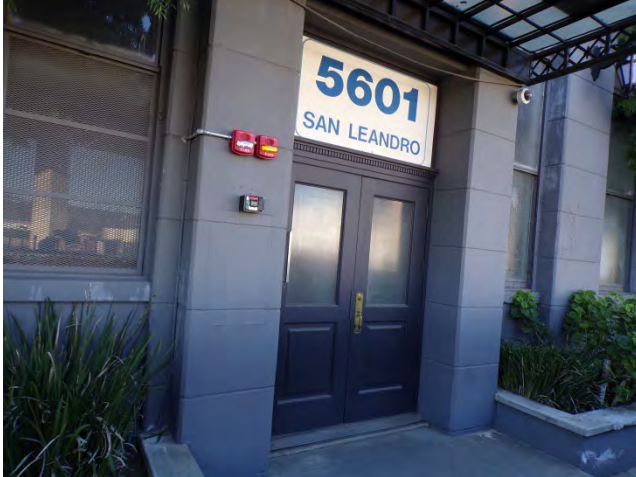
7. Bldg 5601E: Original primary pedestrian entrance along San Leandro Street.
