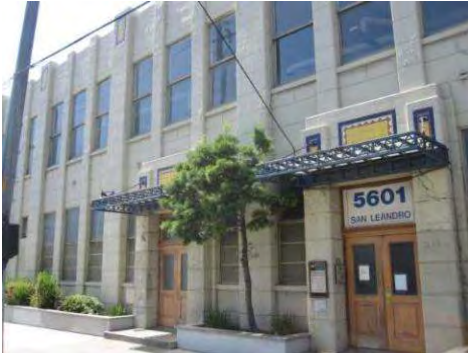
1. The single, two- and three-story, 5601 San Leandro Street, front elevation.
