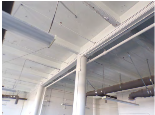
88. Bldg 5601E: Interior finishes and fixtures in office area.
