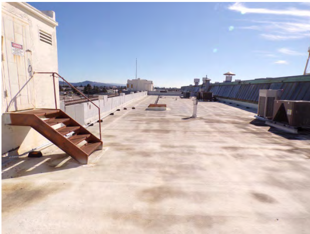
51. Bldg 5601E: The BUR roofing system on the east side of the building, looking south.
