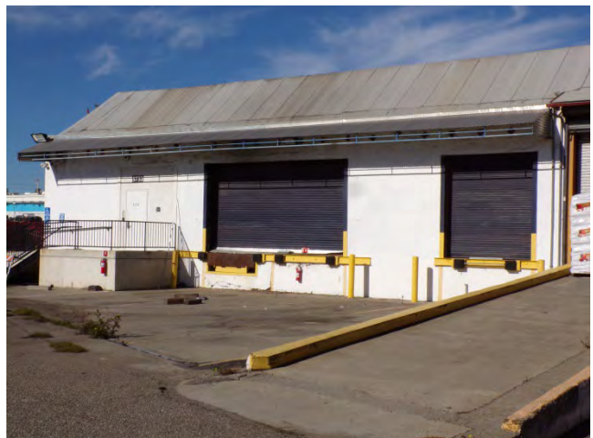
30. Bldg 5733W: Raised loading docks along south elevation.
