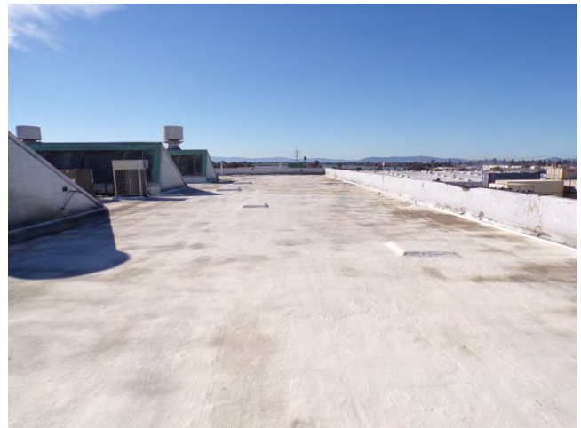
52. Bldg 5601E: The BUR roofing system on the north side of the building, looking west.
