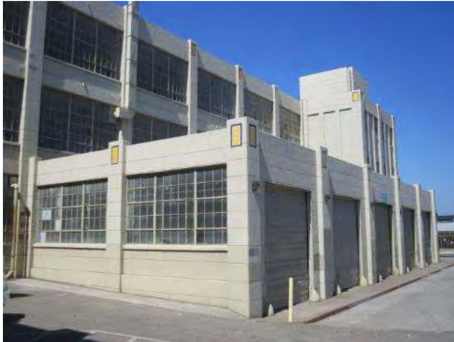
3. The single- and three-story reinforced concrete frame main portion of the building, partial front elevation.
