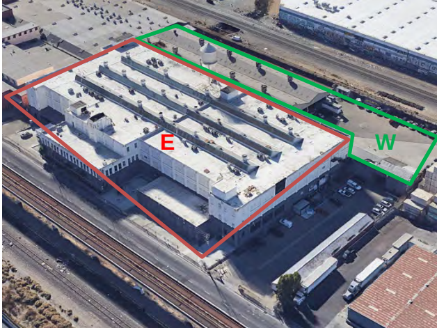
1. Bldg 5601E at bottom of photo (white building); Bldg 5601W at center top of photo with double gable roof.
