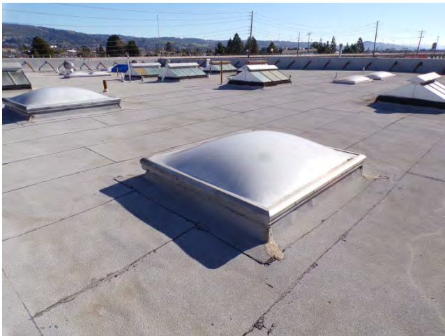
69. Bldg 5733E: Numerous skylights are installed.
