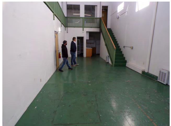
102. Bldg 5733E: Interior finishes and fixtures in apartments.
