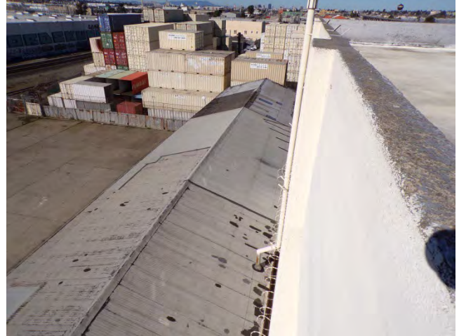
62. Bldg 5601W: The ribbed steel roof panels appear to have had a spray-on coating applied.
