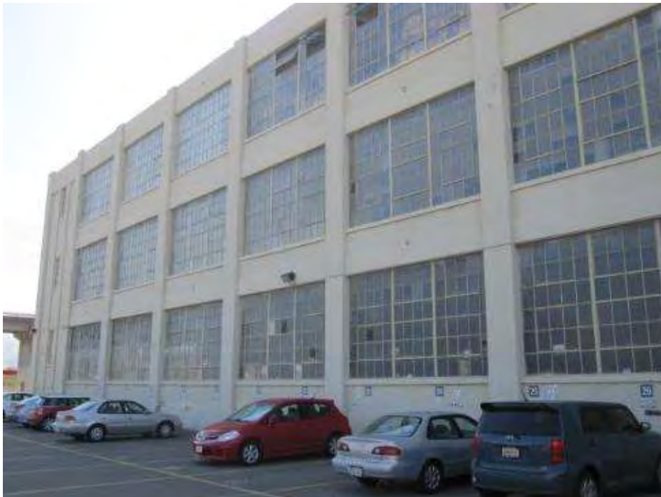
2. The three-story reinforced concrete frame, side elevation.
