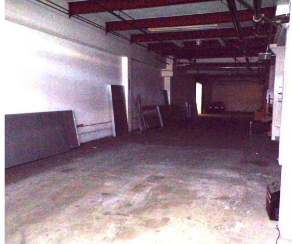
104. Bldg 5733E: Interior finishes and fixtures in parking garage.
