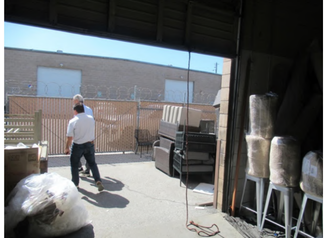
38. The roll-up door at Suite 444 is operational.
