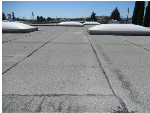
16. Looking south on the roof.
