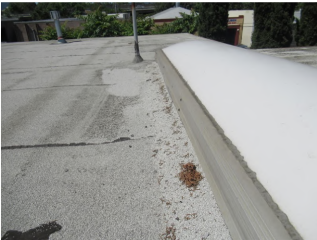
15. Looking west from the roof hatch. The age of the roofing system is unknown. Domed skylight at right.
