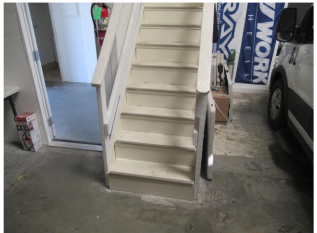
48. The stairs to the mezzanine in Suite 1720.
