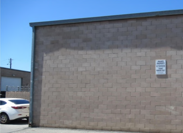
19. The roof drains to gutters along the east and west sides. Downspouts at the building's four corners convey drained water from roof to grade.
