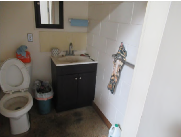
41. Fixtures and finishes in the Suite 460 restroom.
