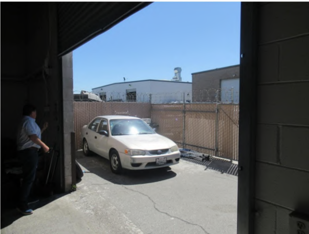
51. The roll-up door at Suite 1720 is operational.
