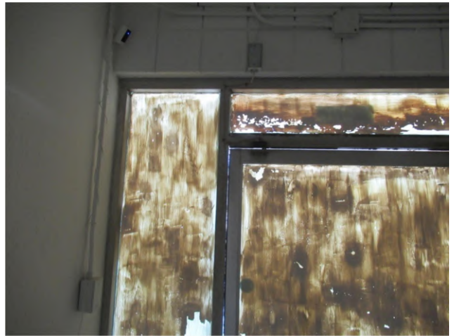
46. The interior side of the entrance glass at Suite 1720 is painted.
