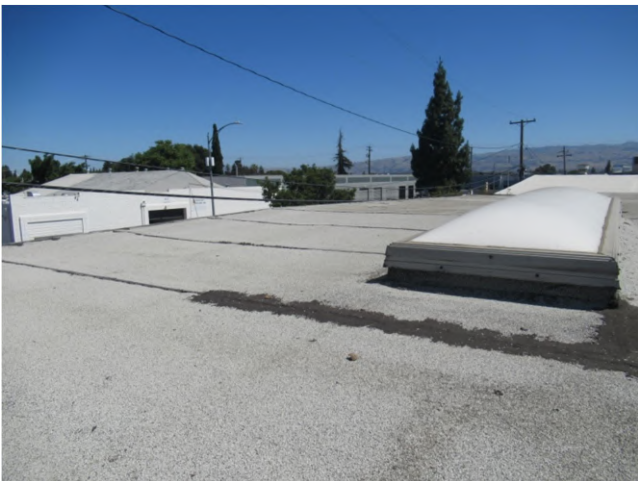
17. Looking northeast on the roof.
