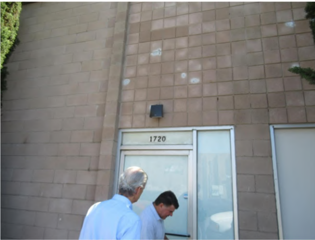
45. The entrance to Suite 1720 has two separated storefront panels.
