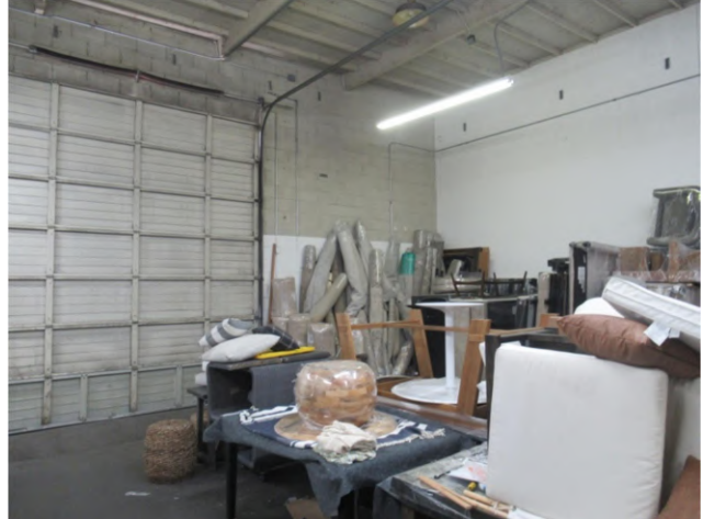
32. First floor interior finishes in Suite 444.
