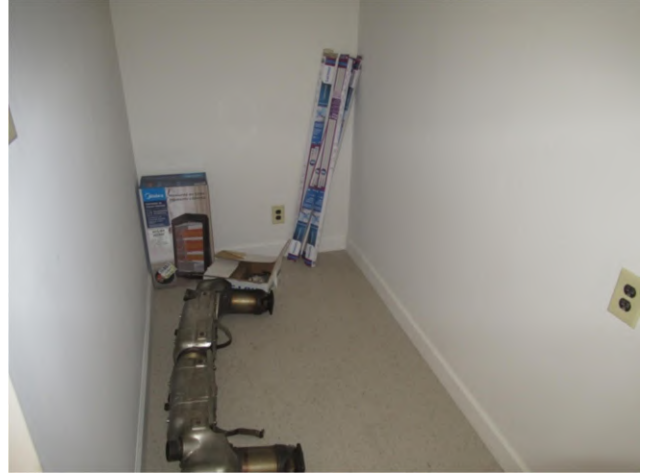
50. Interior finishes on the mezzanine in Suite 1720.
