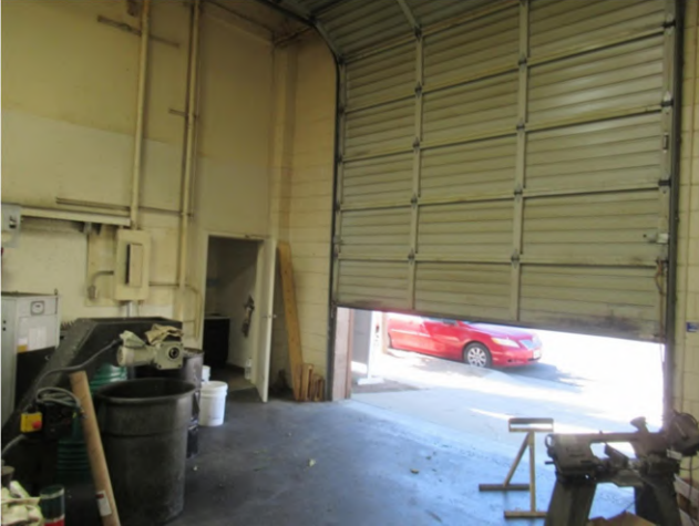
43. The roll-up door at Suite 460 is operational.
