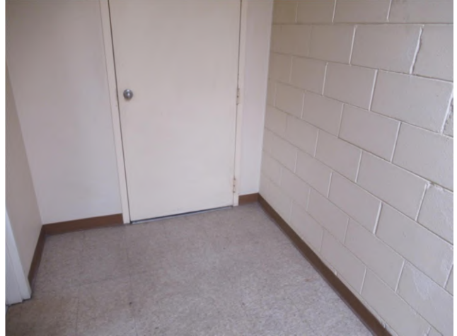
44. Interior finishes on the mezzanine in Suite 460.
