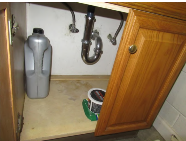
29. The only observed supply pipes were the flexible connections under the sinks; and the only waste pipes observed were the restroom sink drains.
