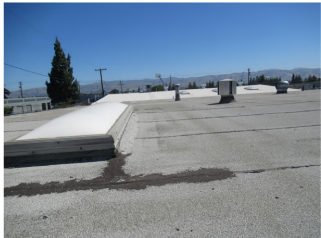
18. Looking east on the roof. A domed skylight and several roof vents are in view. No other HVAC equipment is installed on the roof.
