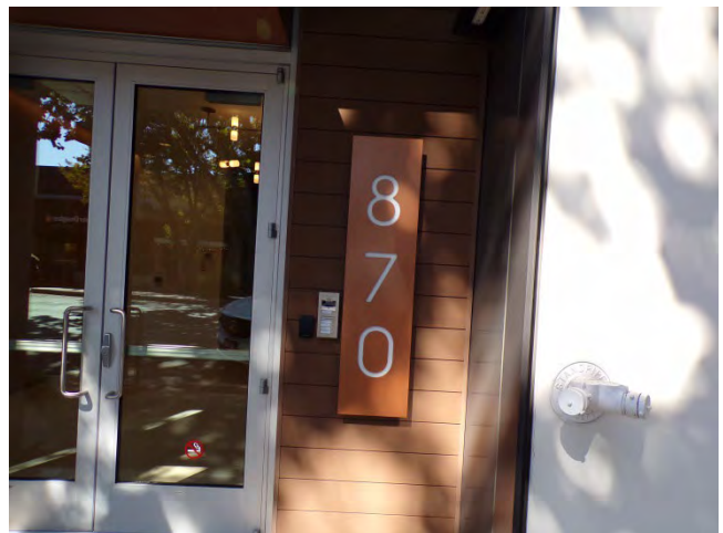
6. Primary address signage at northeast corner of building. FDC shown at right.
