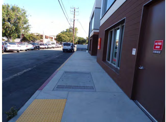
8. View along west elevation walkway, looking north. The large vault is for the PG&E transformer.
