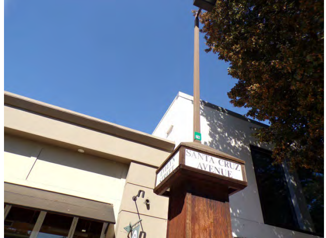
2. Portion of south elevation (white CMU wall) at center of photo above adjacent building.
