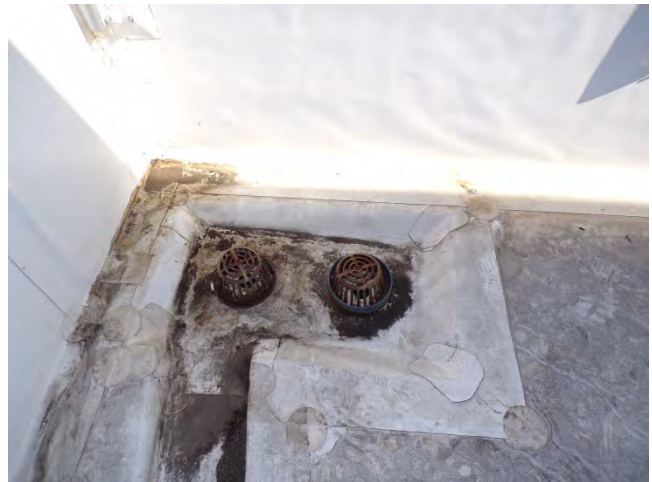
22. Roof and overflow drain combinations are located near the four corners of the building.
