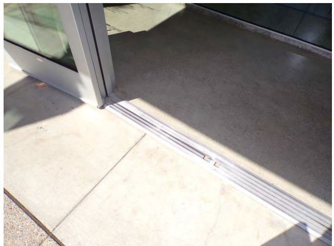
12. Threshold plate and new concrete pour at main entrance along Santa Cruz Avenue into first floor tenant space.
