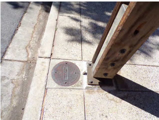
11. Various vaults are located in the sidewalk along Santa Cruz Avenue. A sewer clean-out vault is shown.
