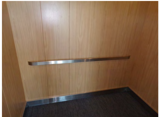
70. A handrail is installed on the back wall of the elevator cab.
