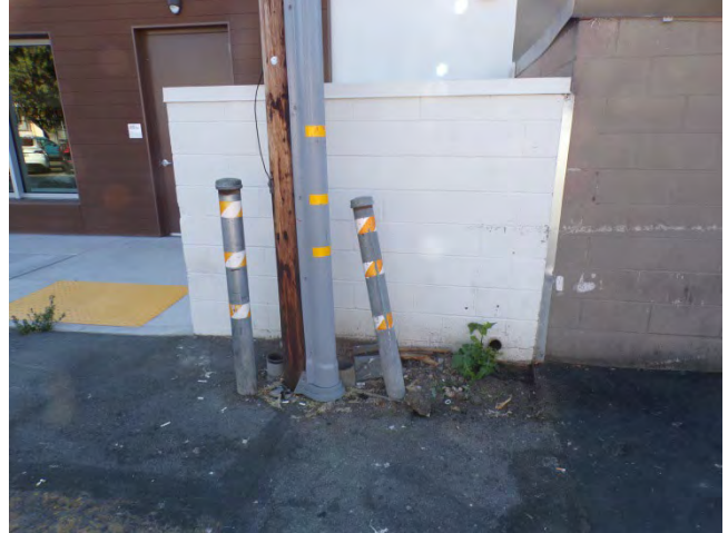
14. The bollards in the parking lot are presumed to be the responsibility of the City. The CMU enclosure behind the bollards contains the gas meter for the subject property.
