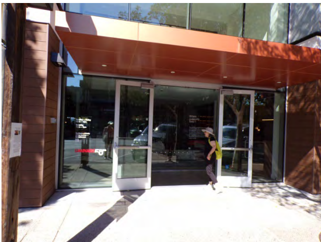
5. Clear anodized aluminum storefront window and door assemblies are installed along the Santa Cruz Avenue elevation (shown) and on the west elevation.
