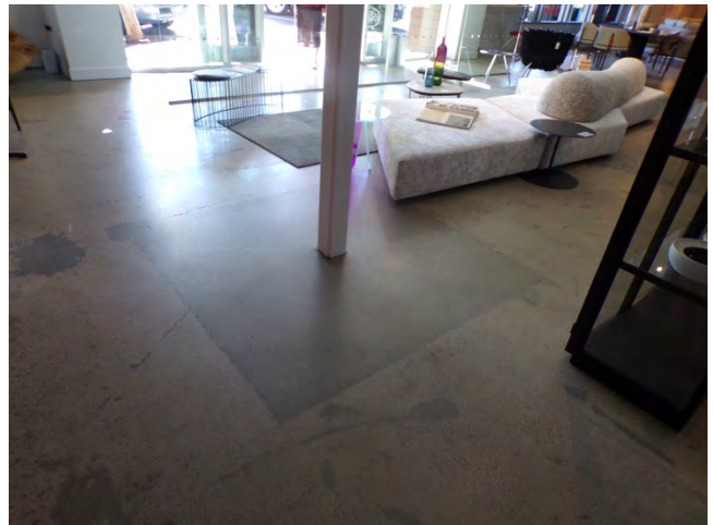
28. First floor: Interior finishes in showroom area. The outline of the enlarged column footing can be seen.
