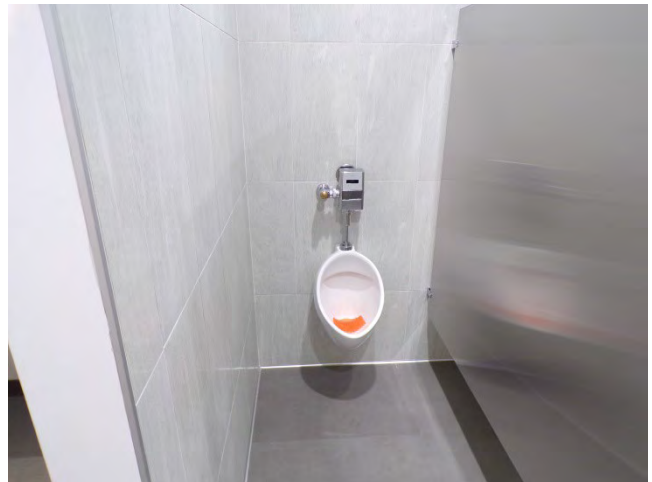
46. First floor: Interior finishes and fixtures in restrooms.
