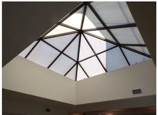
36. Suite 201: Interior finishes, skylight and fixtures.
