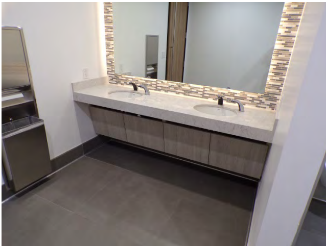
45. First floor: Interior finishes and fixtures in restrooms.
