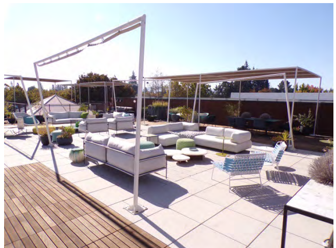
18. Most of the roof is covered with a pedestal flooring system upon which outdoor furniture is displayed.
