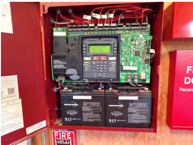
77. The FACP is a FireLite model ES-200, installed in 2022.
