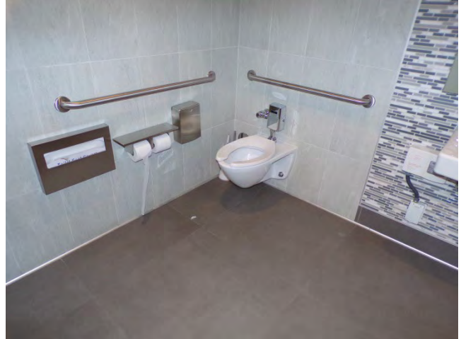
50. Second floor: Interior finishes and fixtures in restrooms.
