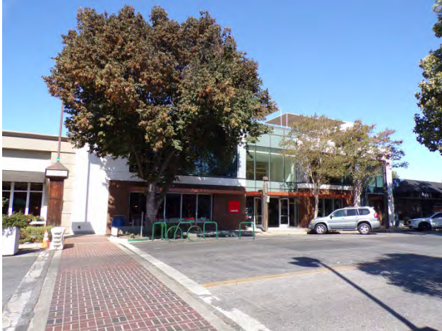
1. East elevation along Santa Cruz Avenue.
