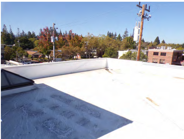
17. The PVC roofing system should be cleaned as part of routine maintenance.
