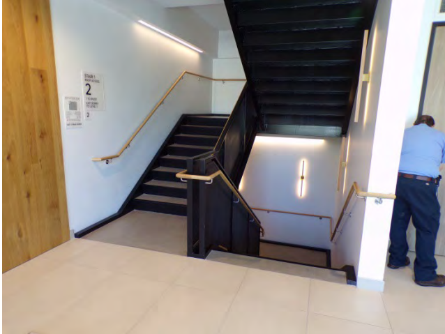
43. Two sets of interior stairs are provided.
