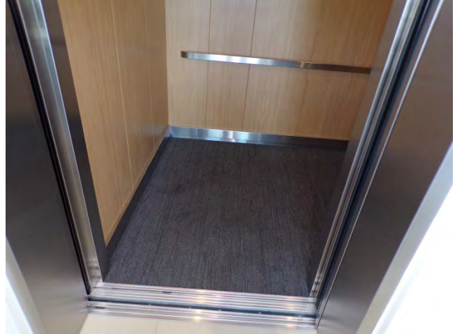
68. Interior finishes in elevator.
