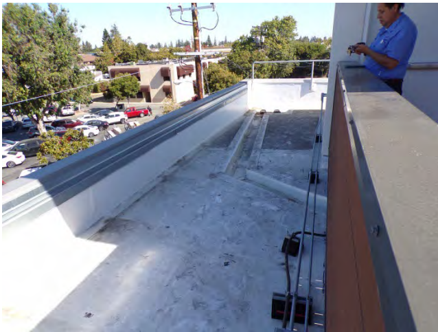
15. The PVC roofing system was installed in November and December of 2020.
