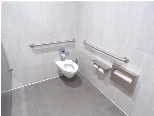
47. First floor: Interior finishes and fixtures in restrooms.
