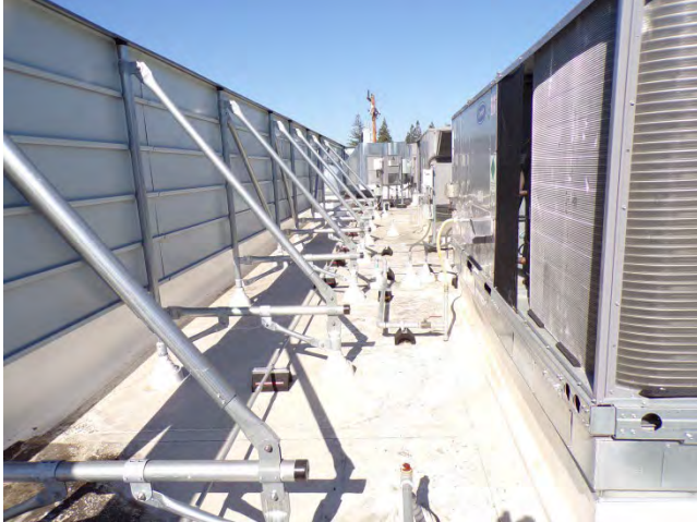
19. The inner face of the mechanical equipment roof screens is shown at left.
