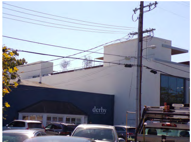
4. North elevation (white CMU wall) above adjacent building.
