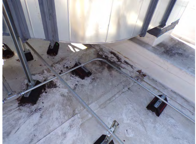
20. The roofing system should be inspected and cleaned as part of routine maintenance.
