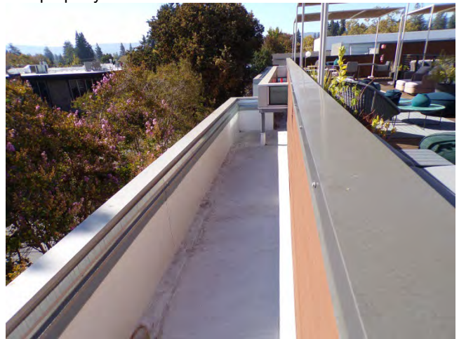
16. The PVC roofing system appeared in "Good" condition.
