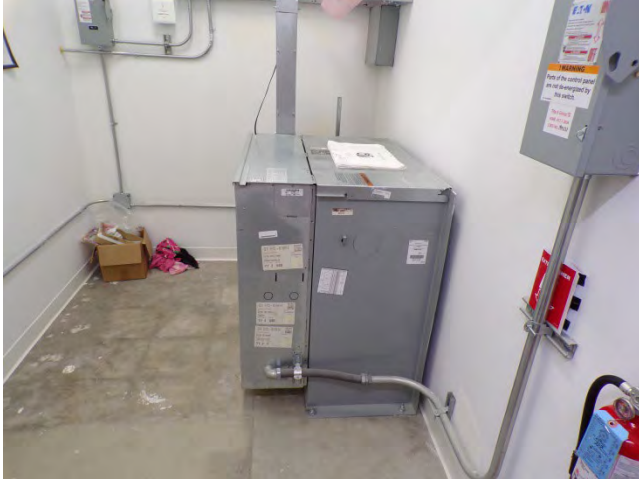
73. The elevator hydraulic load test was last conducted on January 22, 2024.
