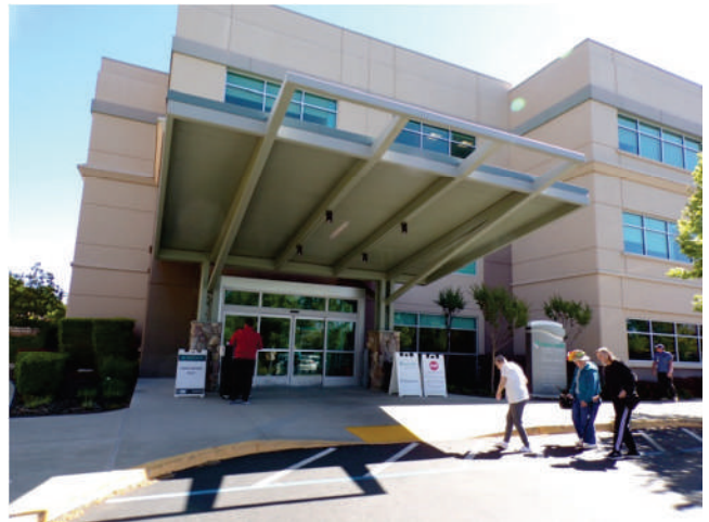
12. MOB 8: Primary pedestrian entrance at northwest corner of building.
