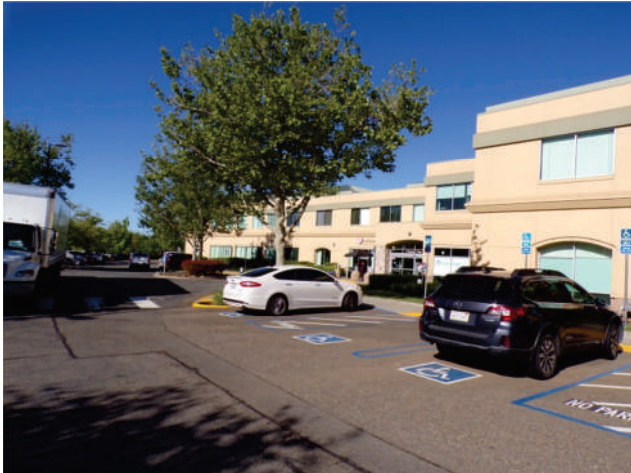
1. MOB 2: West portion of south elevation facing Medical Plaza Drive. Accessible parking also shown.
