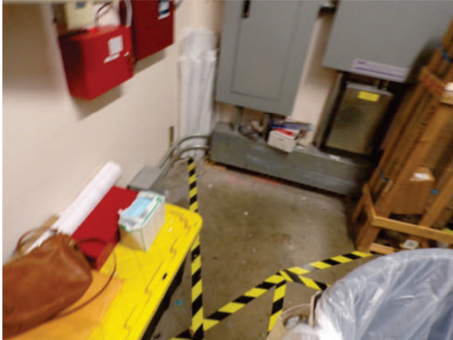
109. MOB 2: Interior finishes and fixtures in service rooms.
