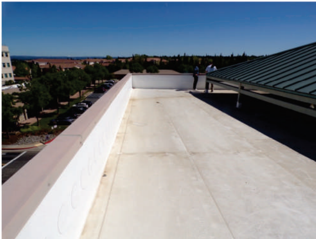
63. MOB 8: The TPO roofing system was installed in 2016 at the time of original construction.
