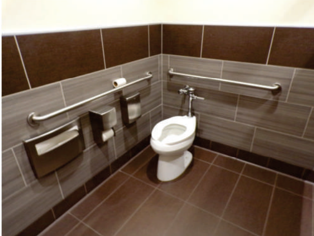
103. MOB 8: Interior finishes and fixtures in restrooms.
