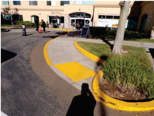
39. MOB 2: Concrete site walkways appeared in generally "Good" condition. Truncated domes are located in required locations.
