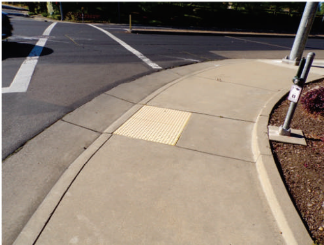
45. MOB 2: Truncated domes are located in required locations.
