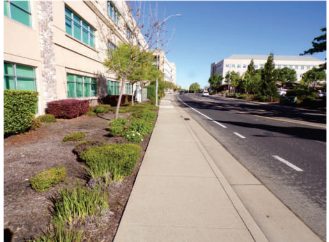
44. MOB 8: Concrete public sidewalk along Medical Plaza Drive.
