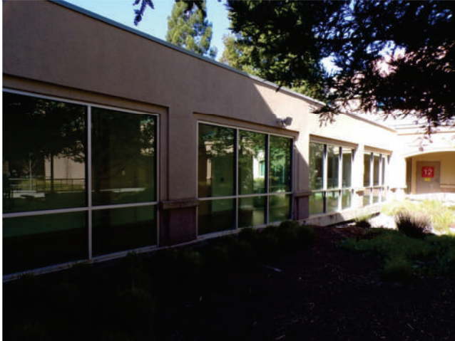
7. One-story connector between hospital in background at right and MOB 2 (out of shot to left).
