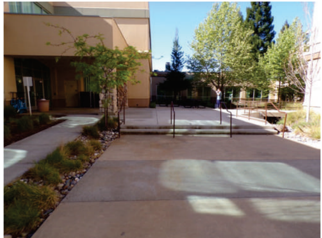
18. MOB 2: The concrete stairs along the north elevation. In background, one-story connector between hospital (at right) and MOB 2 (at left).
