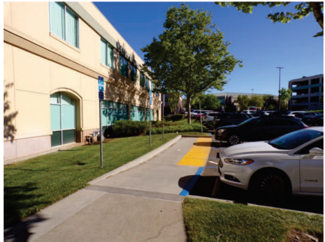
40. MOB 2: Concrete site walkways appeared in generally "Good" condition. Truncated domes are located in required locations.
