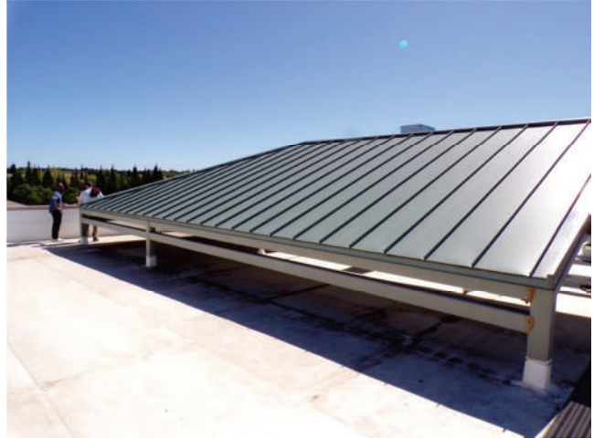
68. MOB 8: The mansards were directly observable from adjacent flat roof areas on this building.
