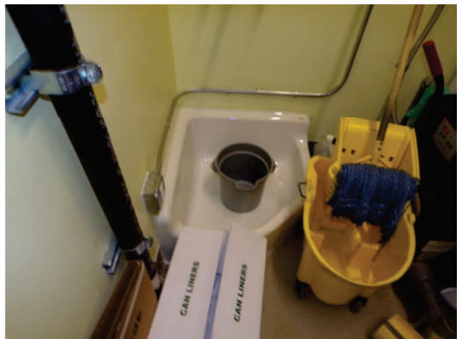
114. MOB 8: Interior finishes and fixtures in service rooms.
