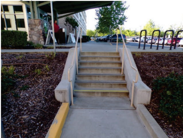
17. MOB 8: The concrete stairs near the primary pedestrian entrance (in background at left).
