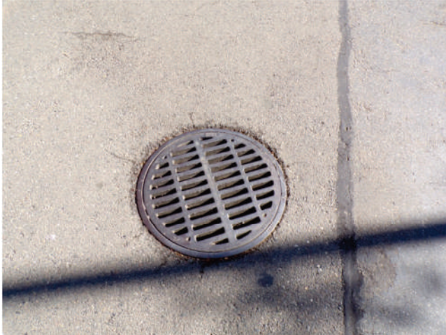
25. MOB 2: Drain inlets are located in several locations in the parking lot.
