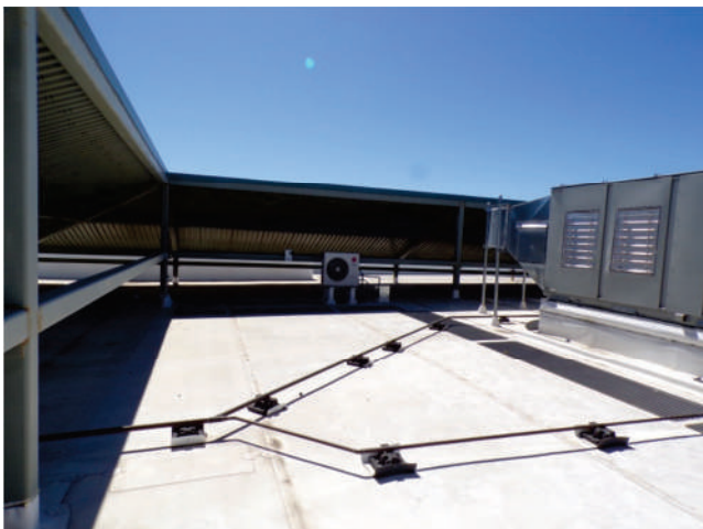
65. MOB 8: The TPO and metal roofing systems both appeared in generally "Good" condition.
