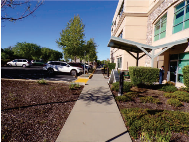
13. MOB 8: Site walkway along east elevation. Canopy at secondary entrance at right.
