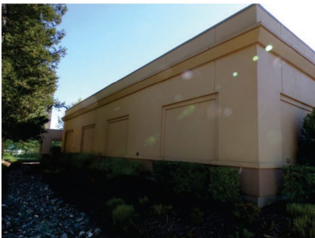
5. MOB 2: North elevation on west side of building at one-story segment. This one-story building segment contains radiation equipment.
