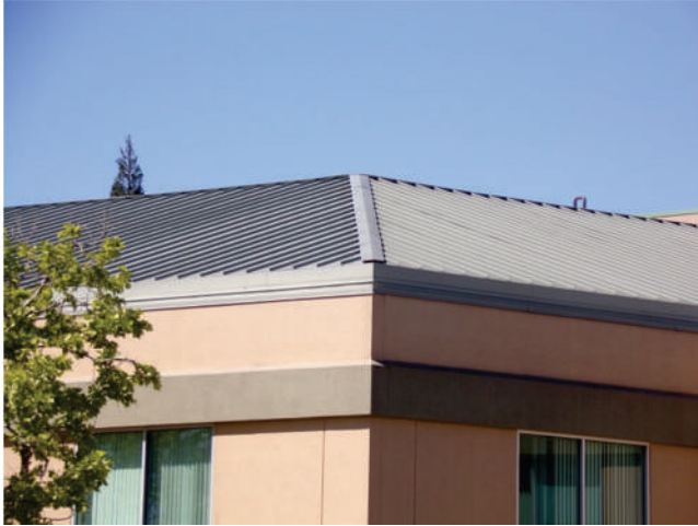
61. MOB 2: The pitched roof mansards on this building could only be observed from grade.
