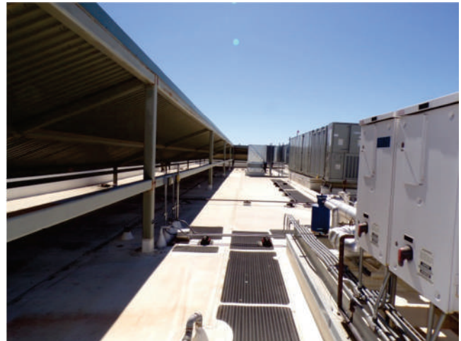
64. MOB 8: The TPO roofing system appeared in generally "Good" condition.
