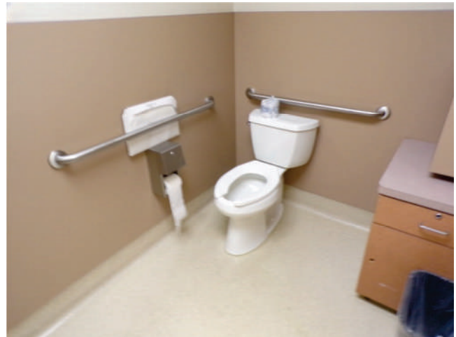
100. MOB 2: Interior finishes and fixtures in older restrooms.
