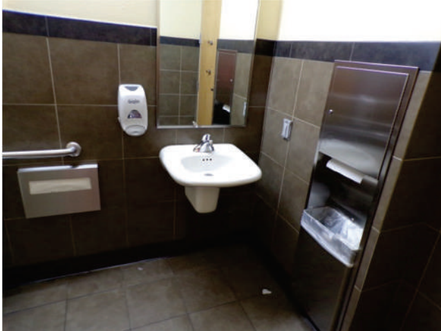
97. MOB 2: Interior finishes and fixtures in remodeled restrooms.
