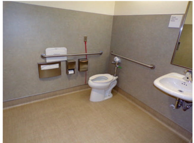
106. MOB 8: Interior finishes and fixtures in patient area restrooms.
