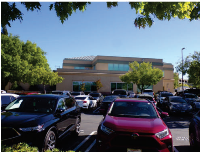
3. MOB 2: West elevation and parking area on west side of building.
