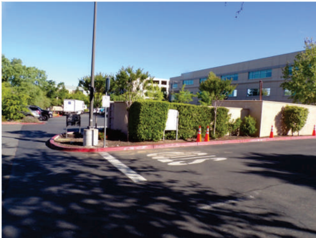
15. Freestanding enclosures for trash (left) and generator (right) near MOB 8 (in background at right).
