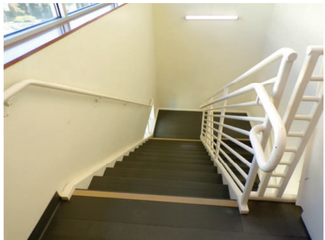
96. MOB 8: Interior finishes and fixtures in fire stairs.
