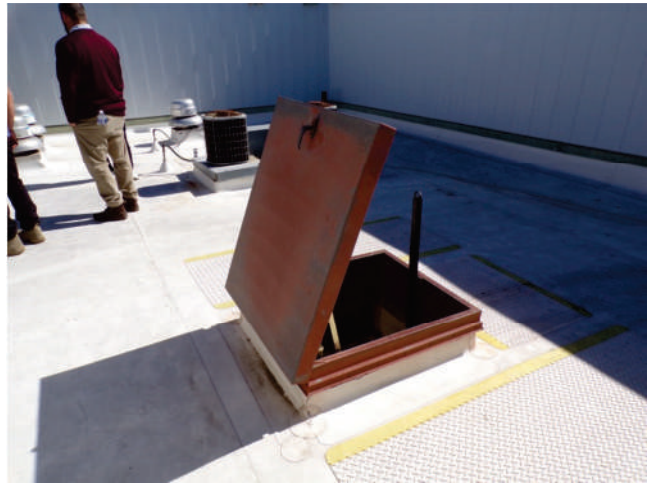
58. MOB 2, north wing: A separate roof hatch provides access to the flat roof area of this wing.
