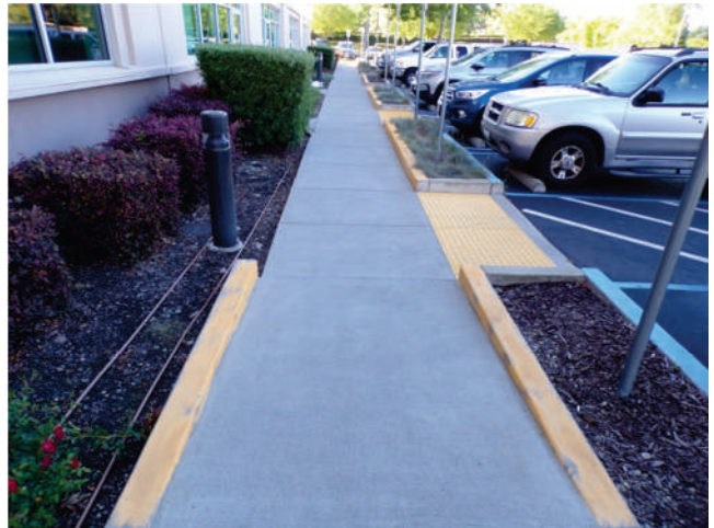
46. MOB 2: Concrete site walkways appeared in generally "Good" condition. Truncated domes are located in required locations.
