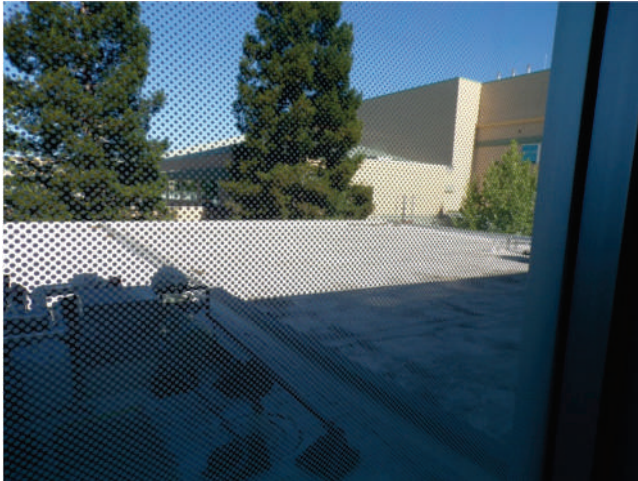
55. MOB 2, south wing: Direct physical access was not possible on the secondary flat roof areas of this building.
