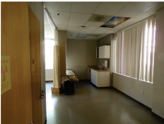
77. MOB 2: Interior finishes and fixtures in open office areas.
