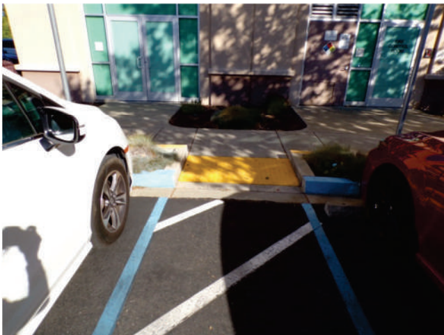
47. MOB 2: Truncated domes are located in required locations.
