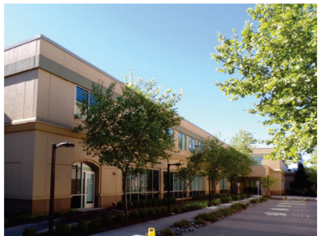
6. MOB 8: North elevation on east side of building.
