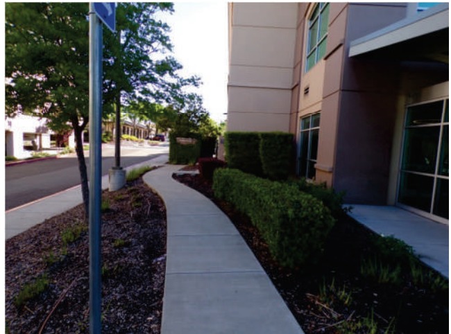
16. MOB 8: The concrete ramp near the primary pedestrian entrance.
