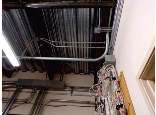
110. MOB 2: Interior finishes and fixtures in service rooms.
