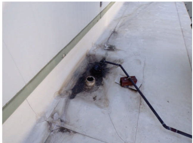
60. MOB 2, north wing: Roof and overflow drains are located in shallow sumps. Accumulation of grime in sumps is typical.
