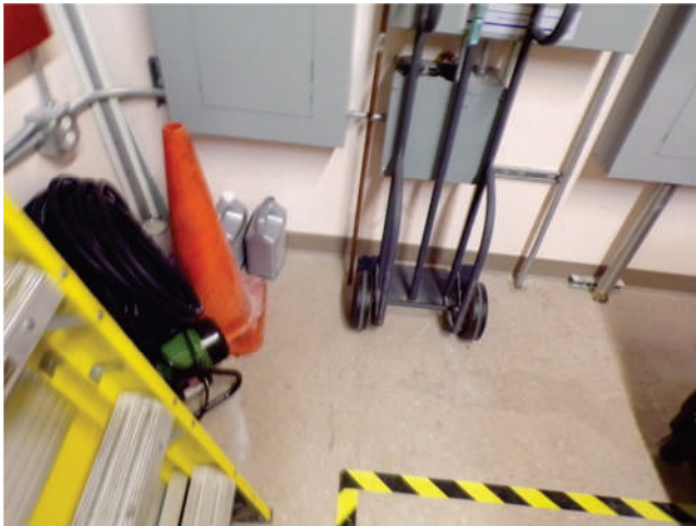
111. MOB 2: Interior finishes and equipment in service rooms.
