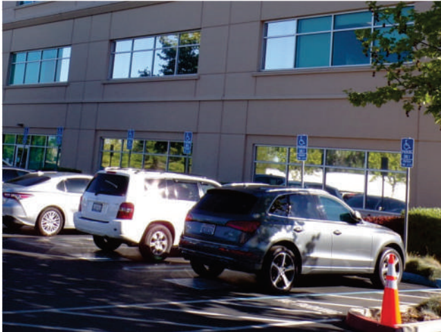
115. MOB 8: Sixteen Accessible parking stalls are provided at this building.
