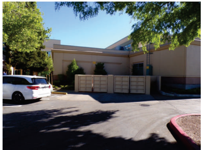
4. MOB 2: West elevation at trash enclosure.
