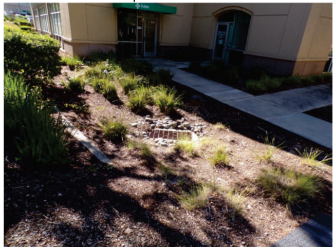
42. MOB 2: Drain inlets are also located in landscaped areas.
