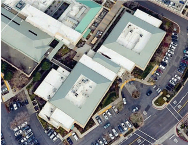
49. MOB 2 has a complex roofing configuration.
