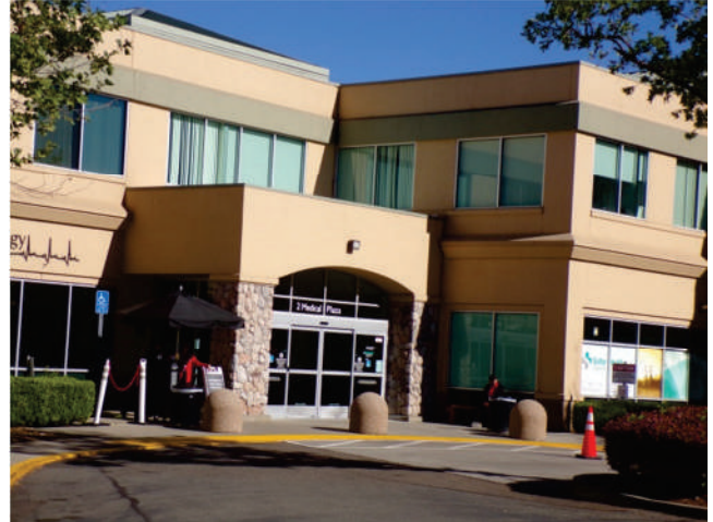
8. MOB 8: Primary pedestrian entrance on south elevation.
