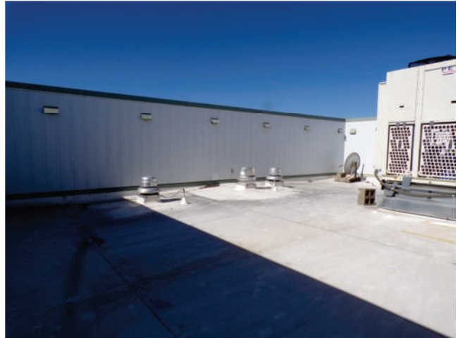
56. MOB 2, north wing: The TPO roofing system was installed in 2018.
