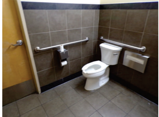
98. MOB 2: Interior finishes and fixtures in remodeled restrooms.
