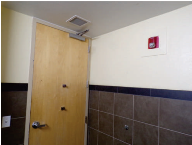
99. MOB 2: Interior finishes and fixtures in remodeled restrooms. Horn/strobe alarm devices are installed in these newer restrooms.
