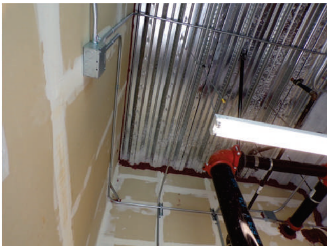
113. MOB 8: Interior finishes and fixtures in service rooms.
