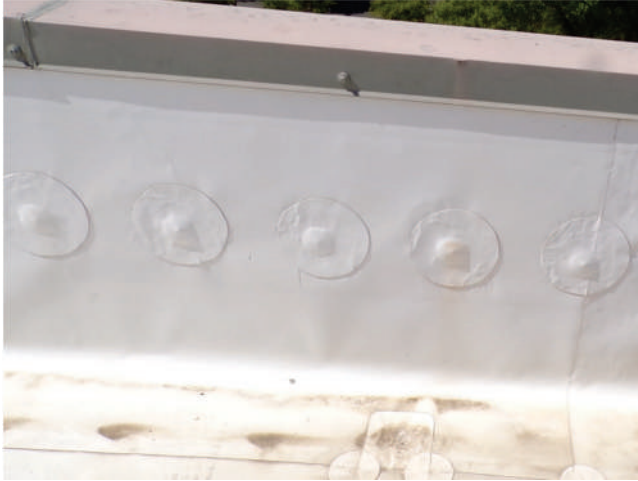
67. MOB 8: The TPO membrane turns up at the parapets and terminates under the parapet cap.
