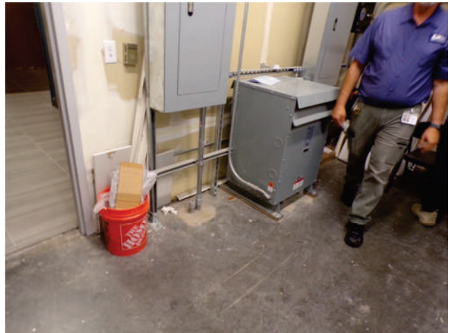
112. MOB 8: Interior finishes and equipment in service rooms.
