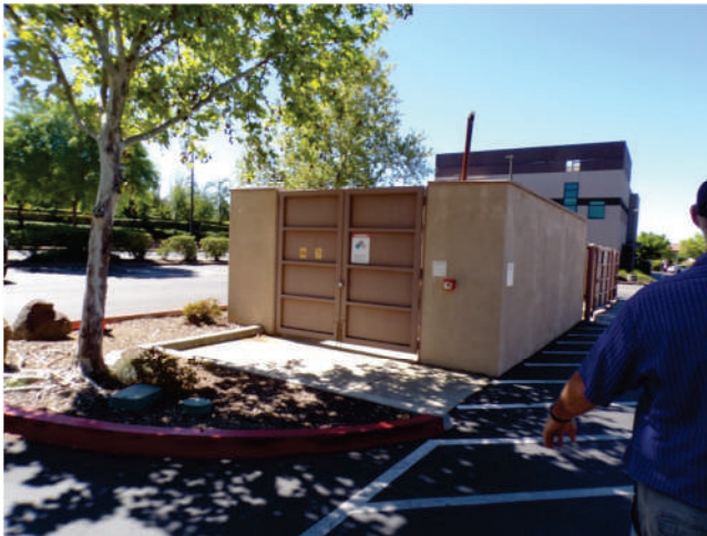
33. MOB 8: CMU generator enclosure.
