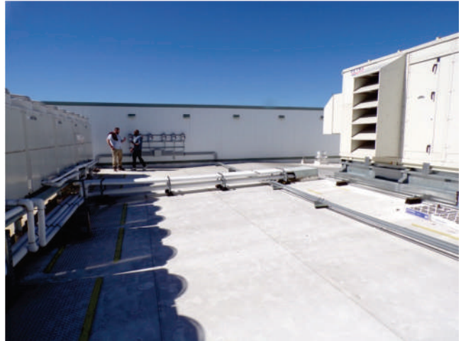
50. MOB 2, south wing: The TPO roofing system was installed in 2018.
