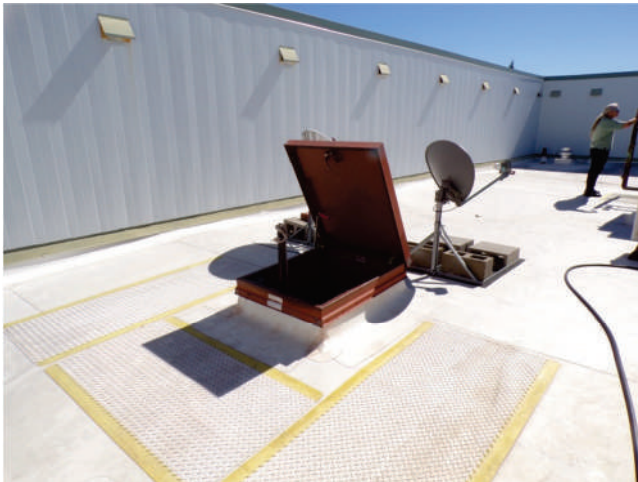
51. MOB 2, south wing: A roof hatch provides access to the flat roof equipment well of this wing.
