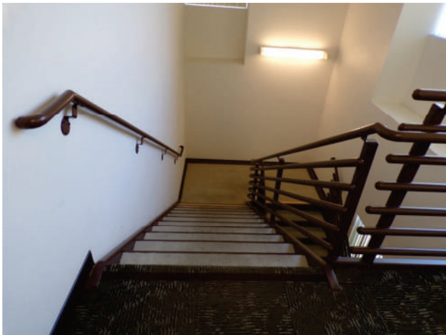
83. MOB 2: Interior finishes and fixtures in fire stairs.
