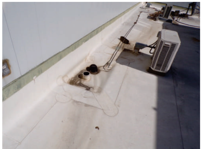
54. MOB 2, south wing: Roof and overflow drains are located in shallow sumps.
