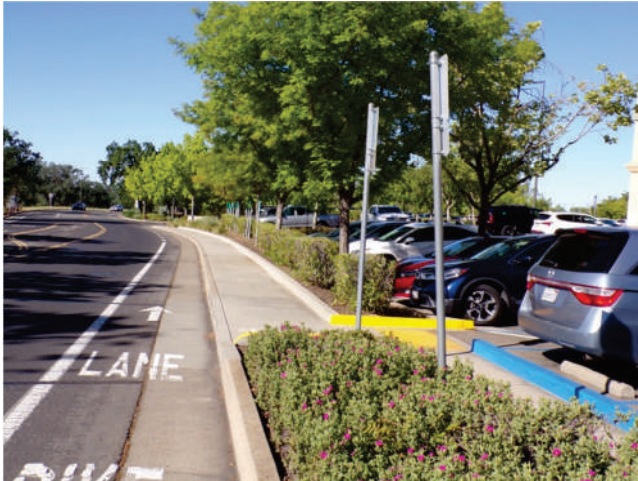
37. MOB 2: Concrete public sidewalk along southwest quadrant of site.
