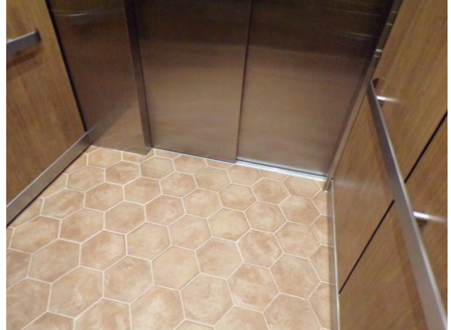
86. Main Bldg: Interior finishes and handrails in freight elevators.
