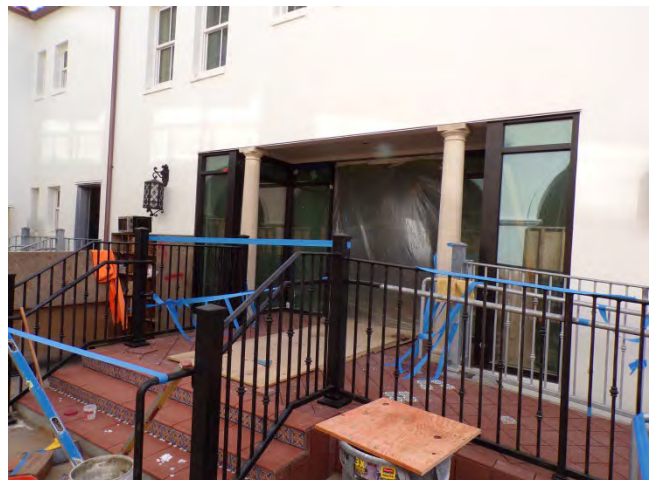
12. Tower Bldg: Primary pedestrian entrance.
