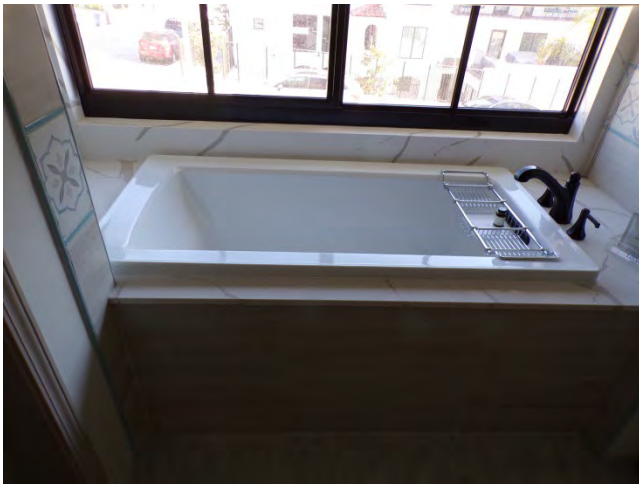
39. Main Bldg: Interior finishes and fixtures in guestroom bathrooms.
