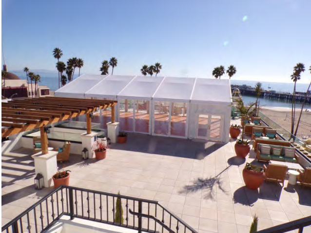
97. Main Bldg: The tent structure is a temporary installation, only used in cold weather months.
