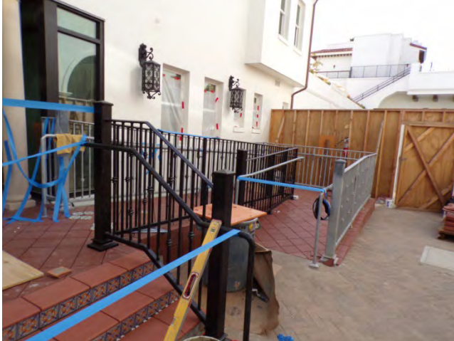
13. Tower Bldg: Wheelchair ramp along north elevation.
