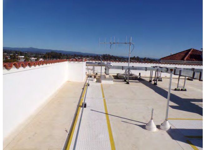
14. Main Bldg: The TPO roofing system is date stamped February 2024.
