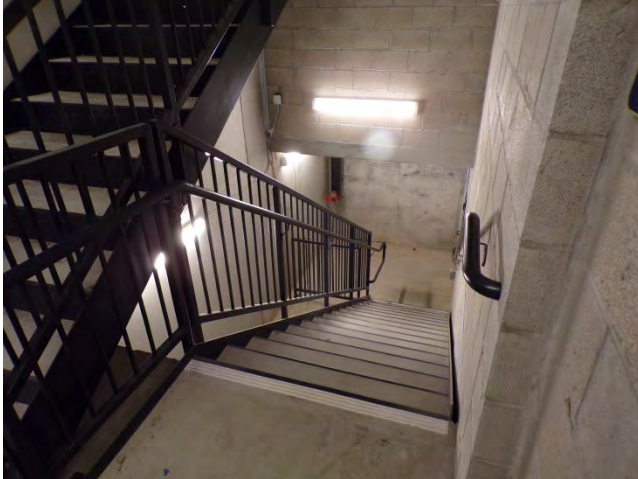
43. Main Bldg: Numerous sets of interior stairs are installed.
