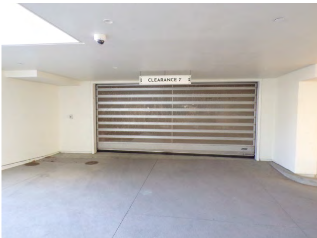
53. Main Bldg: Vehicular entrance to the parking garage for basement and first floor levels. This entrance is located near the southwest corner of the building.
