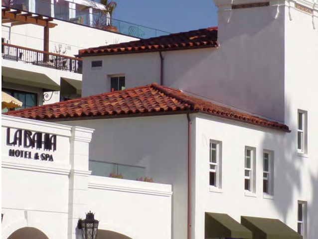
19. Tower Bldg: The red barrel tile roofing system was reportedly installed in August 2025.
