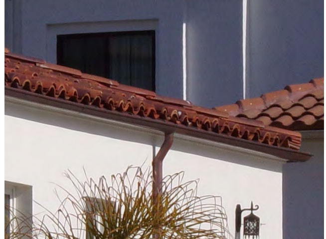
20. Tower Bldg: Gutters and downspouts provide roof drainage.
