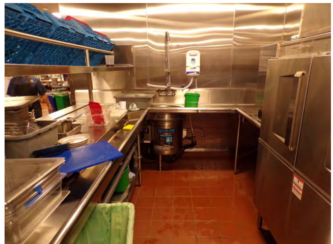
30. Main Bldg: Interior finishes and fixtures in kitchens.
