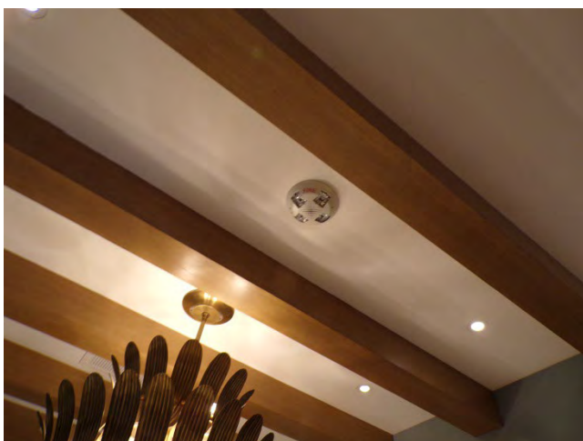
77. Horn/strobe alarm device placements appeared compliant with current Accessibility codes.
