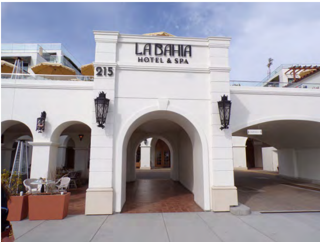
9. Primary pedestrian entrance along Beach Street.
