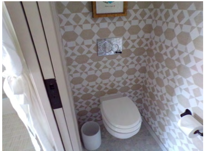
40. Main Bldg: Interior finishes and fixtures in guestroom bathrooms.
