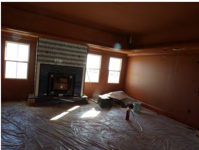
47. Tower Bldg: Interior finishes and fixtures.
