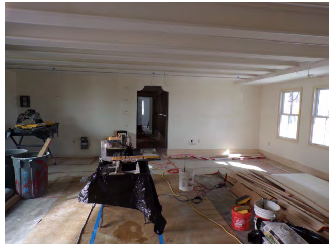
46. Tower Bldg: Interior finishes and fixtures.
