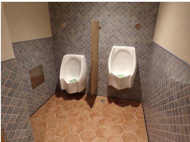
89. Main Bldg: Interior finishes and fixtures in restrooms. Waterless urinal are installed.
