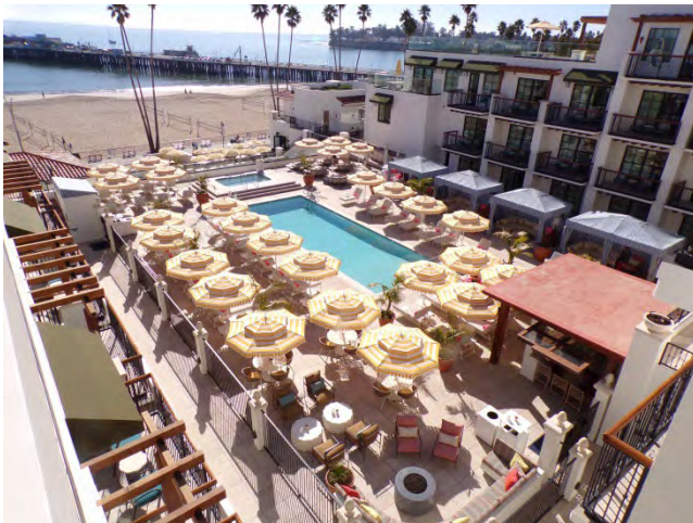
93. Main Bldg: The swimming pool is at third floor level.
