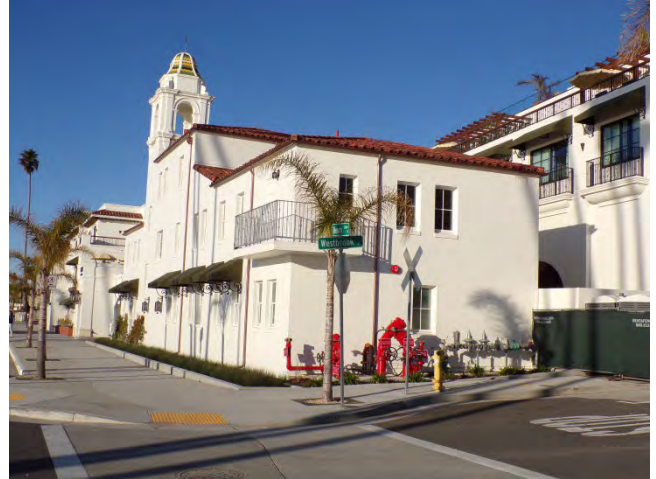
8. Tower Bldg: East elevation at center of shot.
