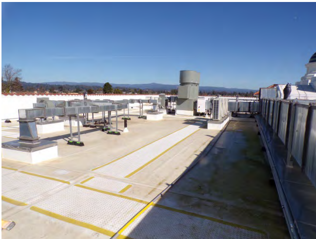
15. Main Bldg: The TPO roofing system is date stamped February 2024.
