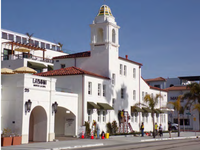
7. Tower Bldg: South elevation at center of shot.
