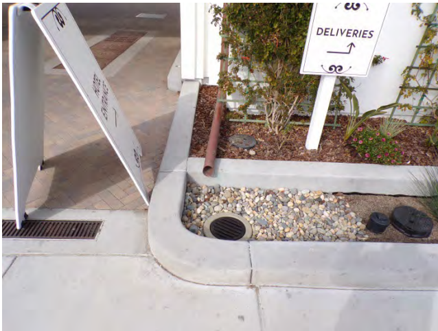
21. Tower Bldg: Downspouts discharge at slightly above grade to nearby drain inlets.
