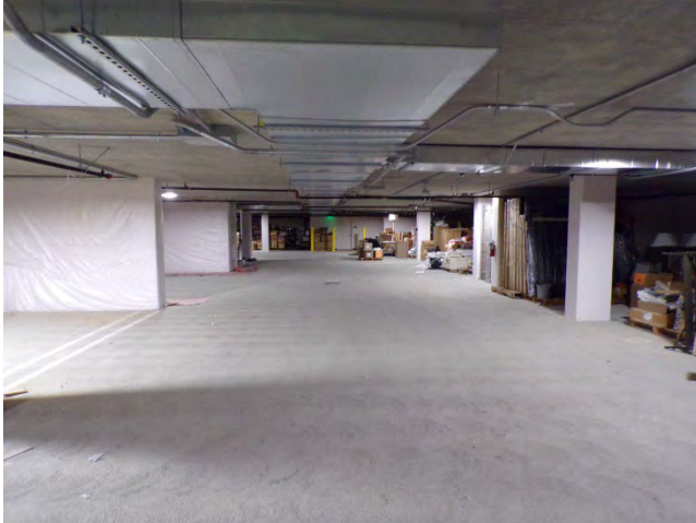
49. Main Bldg: The parking garage is located on the basement level (shown) and on the first and second floors.
