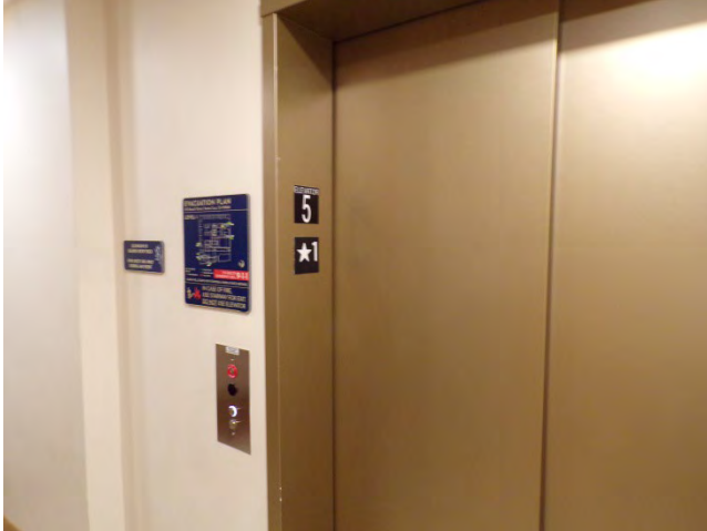
85. Main Bldg: Two Otis freight elevators are installed.
