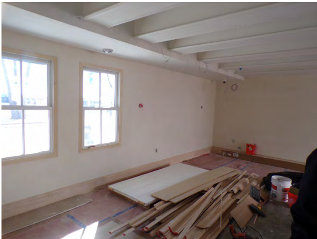
45. Tower Bldg: Interior finishes and fixtures. Construction was underway at the time of our site visit.
