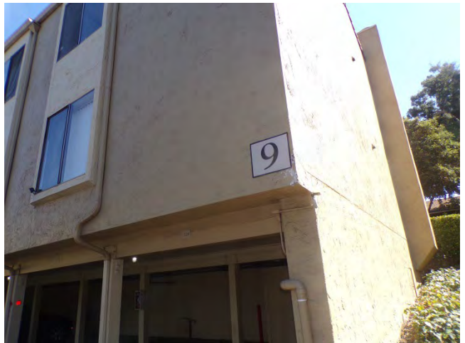
10. Bldg 9: North elevation. Buildings also carry identification signs mounted on an exterior wall.
