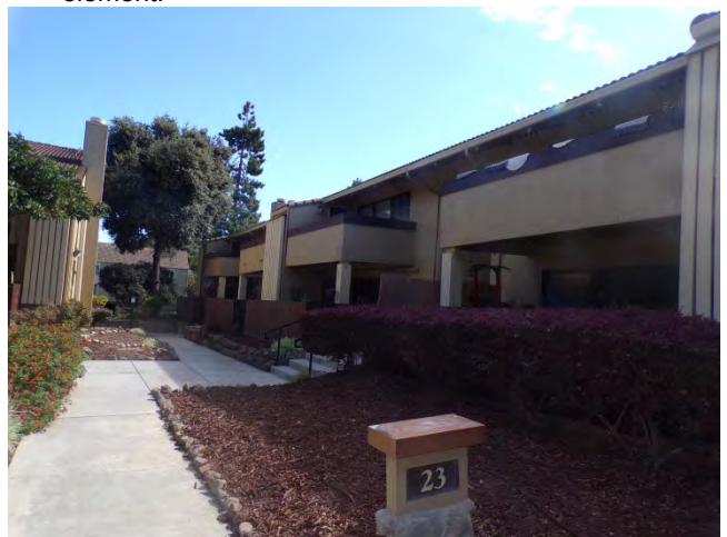
24. Bldg 23: East elevation. Original design stucco and wood balcony railings are still installed on this building.
