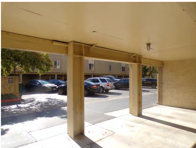
35. Bldg 34: Two welded steel moment frame braces are installed on each building with tuck-under parking.
