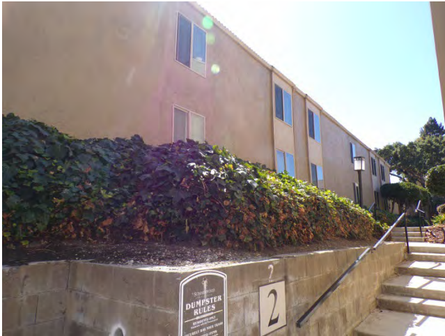
3. Bldg 2: North elevation. This is one of 12 buildings without tuck-under parking.
