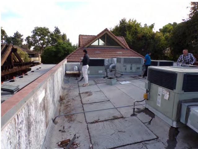
47. Clubhouse: The BUR roofing system was reported to have been installed between 2007 and 2011.
