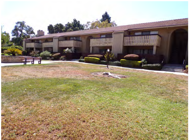
6. Bldg 5: Partial view of east elevation. Some landscaping elements are in a degraded condition. Dead grass and tree stump shown.
