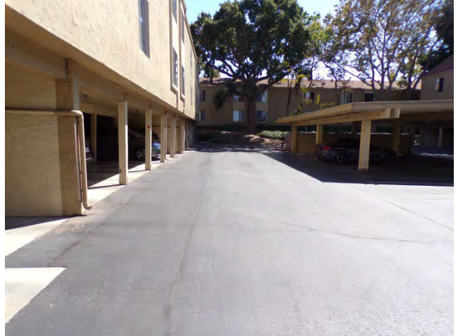
92. The asphalt paving appeared in generally "Good" condition, though it is not without deficiencies.
