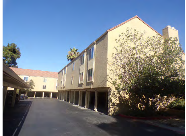
38. Bldg 37: West elevation and asphalt-paved parking area.
