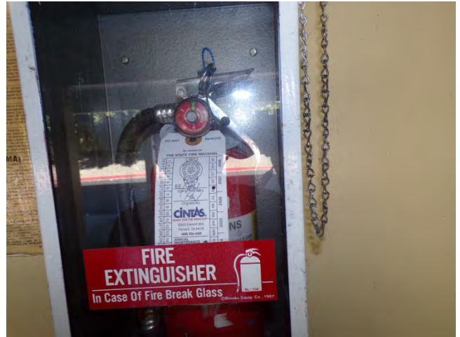
112. All observed fire extinguishers had current inspection tags.
