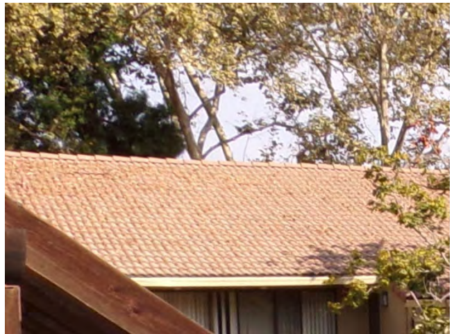
46. Red concrete barrel tile roofs were installed on all buildings between 2007 and 2011.
