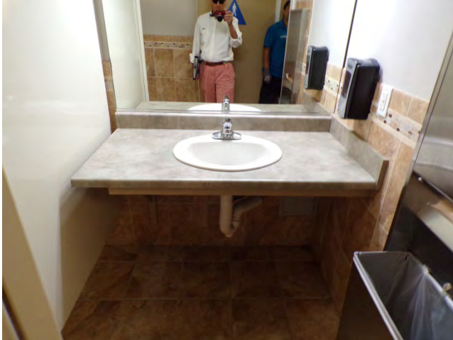
73. Clubhouse: Interior finishes and fixtures in restroom.
