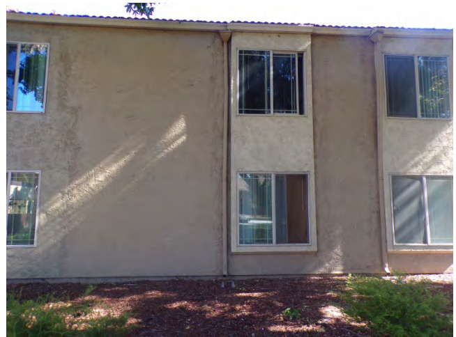
34. Bldg 33: North elevation. New plastic frame windows were installed in this building—and others—in 2014.
