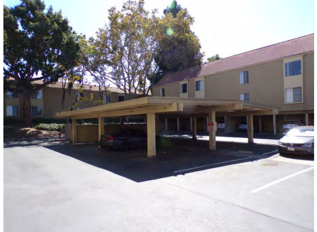
44. Six wood-framed carports are provided.
