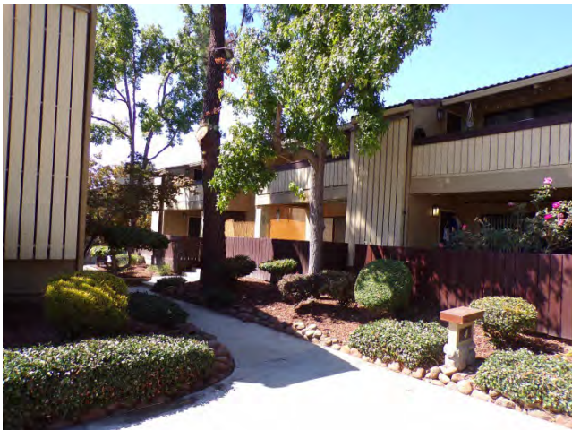
5. Bldg 4: Partial view of south elevation. Landscaping is attractive and appeared in generally "Good" condition.
