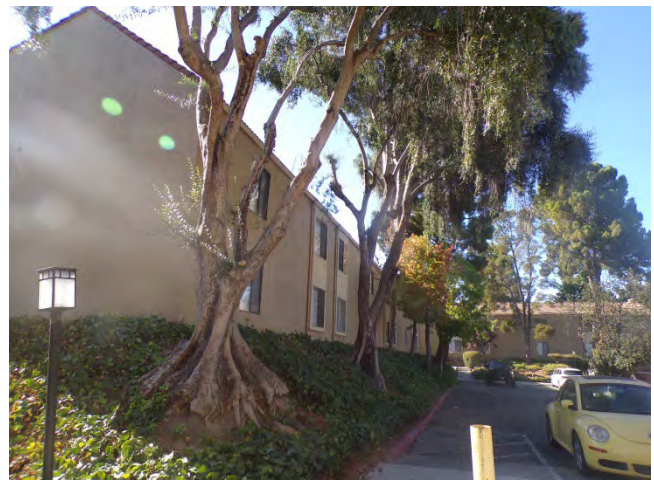
42. Bldg 41: East elevation. A sense of the slopes at the site and the changes in elevation can be gained from this photo.
