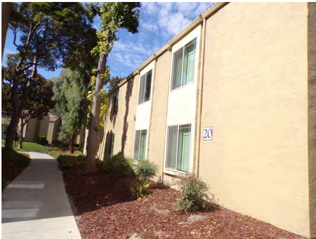
21. Bldg 20: This building is one of 12 without tuck-under parking.
