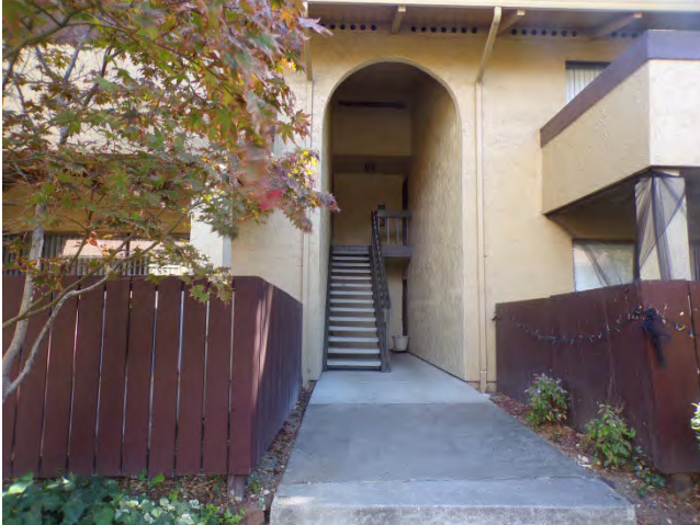
13. Bldg 12: North elevation. AllWest considers the open-air stairs at the residential buildings to be exterior stairs.
