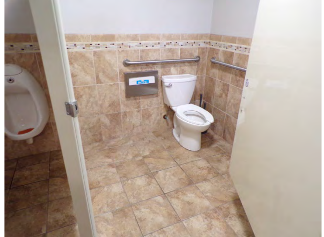
74. Clubhouse: Interior finishes and fixtures in restroom.
