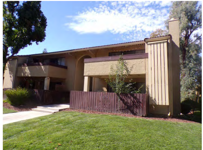
16. Bldg 15: South elevation. The primarily stucco and wood trim balcony railing on both the long and short sides of the balcony is the original design.
