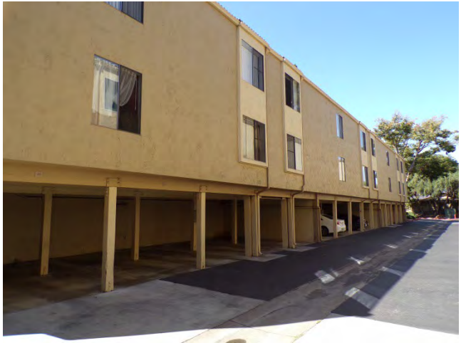
4. Bldg 3: East elevation. Tuck-under parking is provided in 28 buildings.
