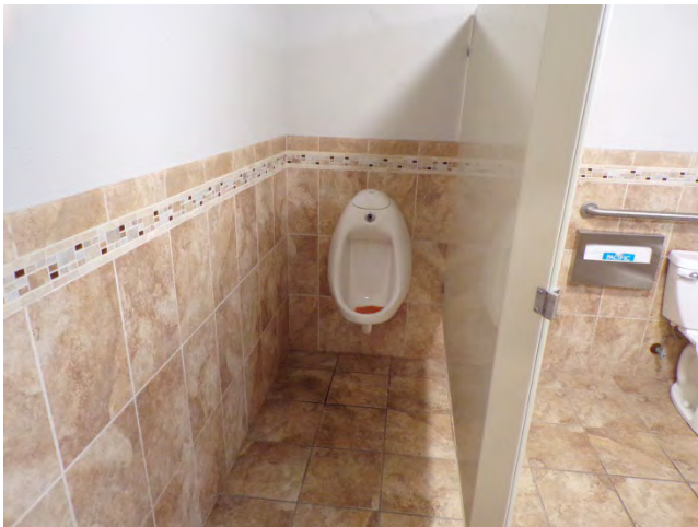
75. Clubhouse: Interior finishes and fixtures in restroom.
