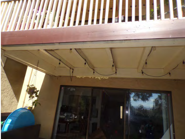
19. Bldg 18: The original balcony design incorporated a concrete balcony deck.
