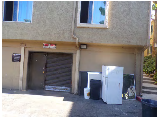
28. Bldg 27: The maintenance office is located in this building behind the roll-up door.
