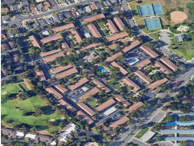
1. The subject property contains forty residential buildings and two non-residential buildings.
