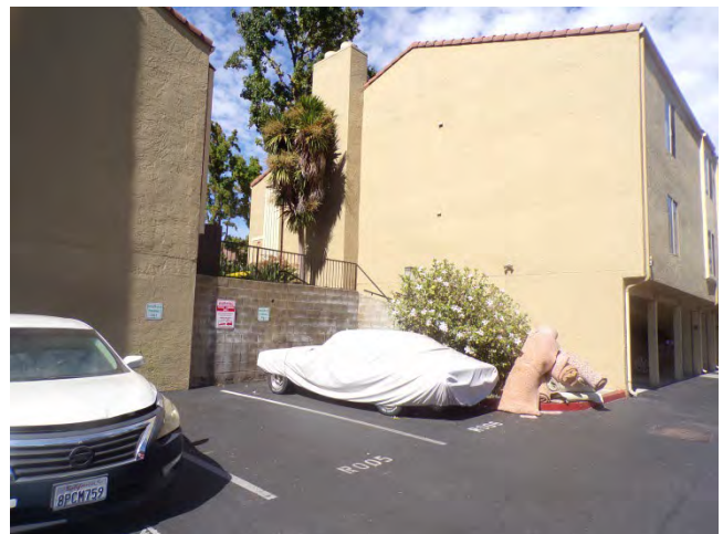
18. Bldg 17: South elevation. A sense of the slopes at the site and the changes in elevation is discernable in this photo.
