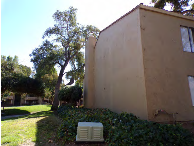
7. Bldg 6: East elevation. Short elevations on the residential buildings have no windows.
