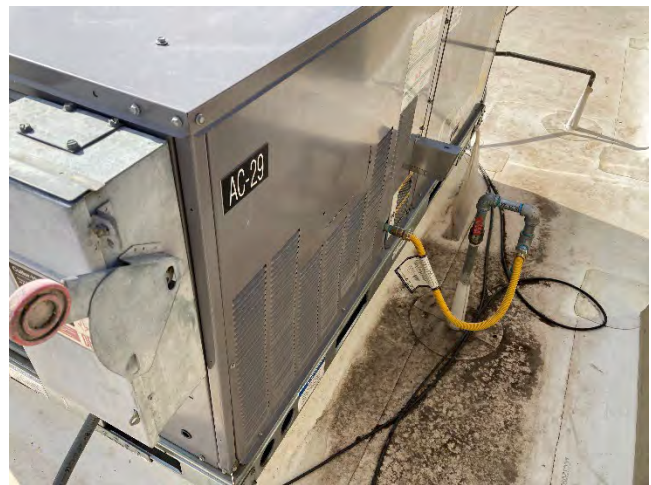
M-4. Main Bldg: Air conditioner with flexible natural gas connection.
