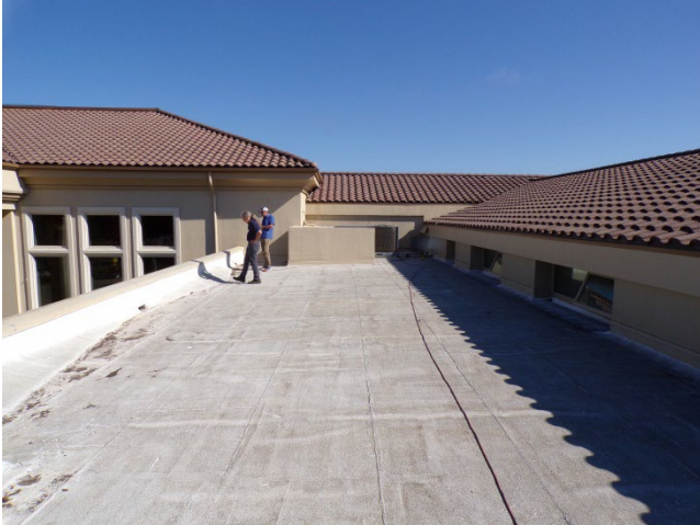
37. Main Bldg: Southeast wing BUR roof. This is the only BUR roofing system remaining on Main Bldg. Concrete barrel tiles shown on adjacent pitched roof areas.
