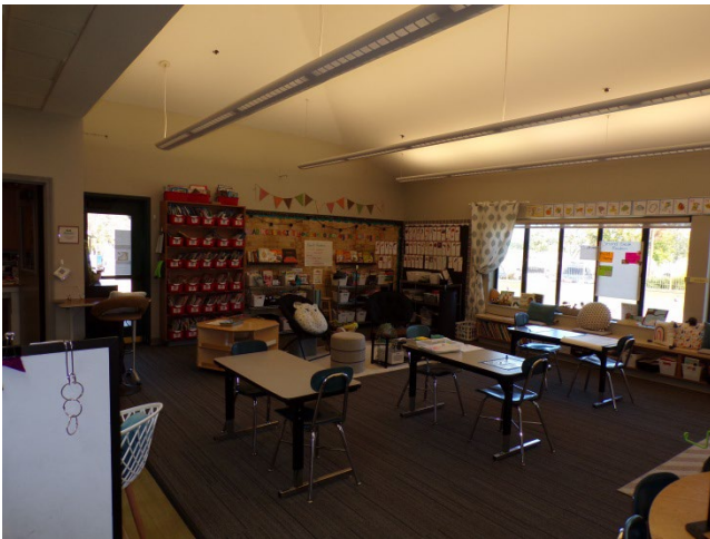
51. Main Bldg: Typical classroom.
