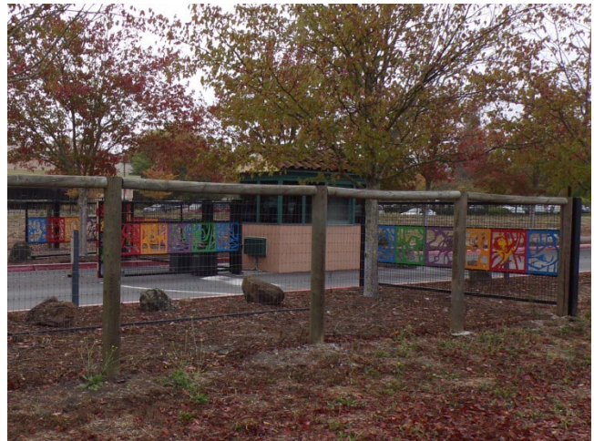
16. Guard building along entrance drive.
