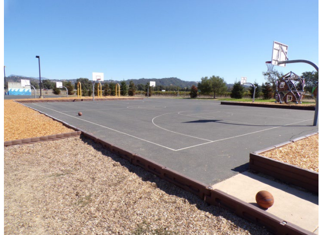
20. Asphalt-paved play area to east of Gym.
