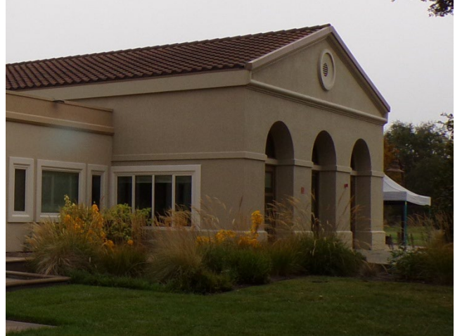
2. Main Bldg: Library wing at southeast corner of building.
