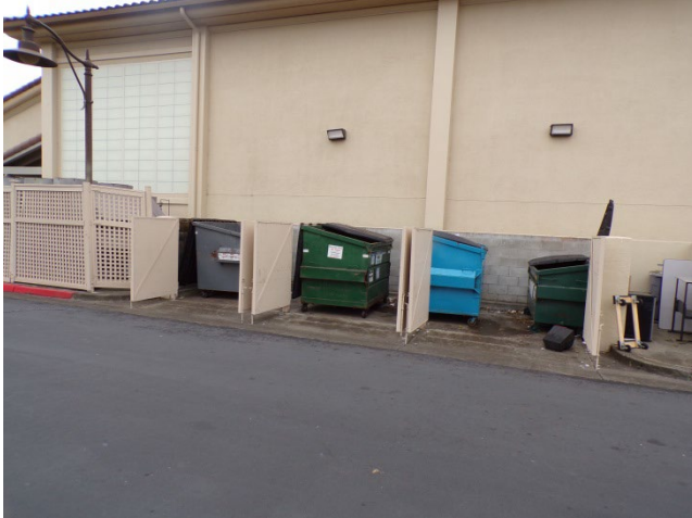
25. Dumpster enclosure at rear of Gym.
