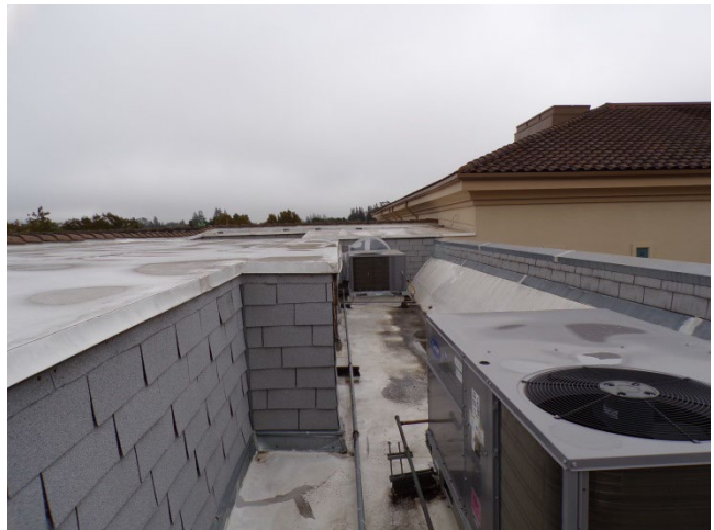
34. Main Bldg: Northwest wing TPO roof looking east-southeast.
