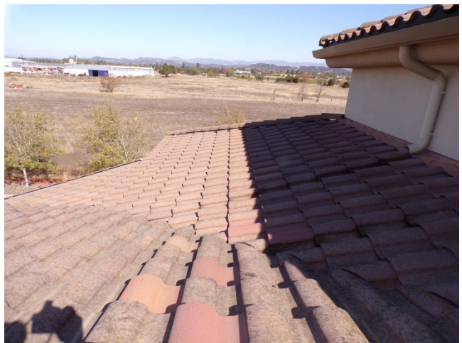
42. Gym: Concrete barrel tile roofing systems.
