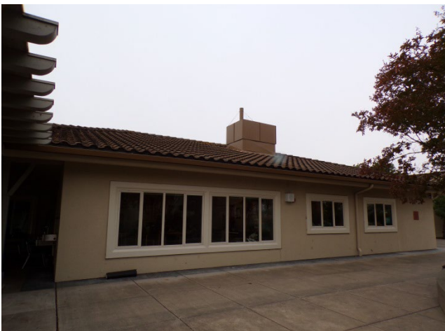
5. Main Bldg: Portion of north elevation at northeast corner of building.
