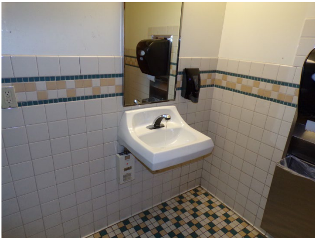
63. Gym: Typical restroom finishes.
