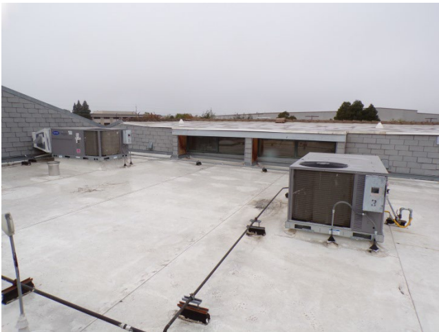
33. Main Bldg: Northwest wing TPO roof, looking northwest.
