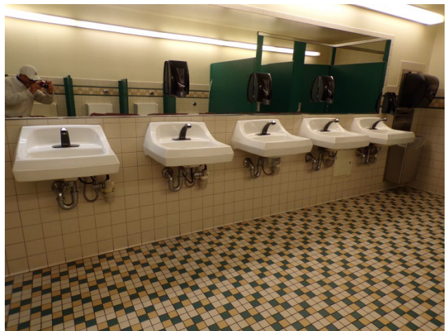
72. Typical sink and accessories generally meet Accessibility requirements, though many sinks lack drain pipe insulation; Main Bldg restroom shown.
