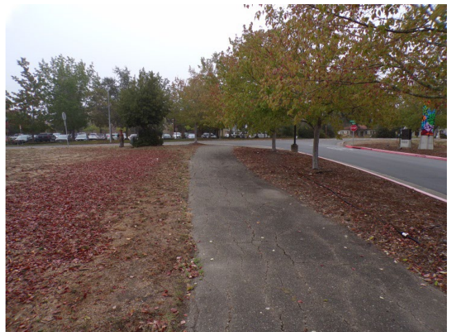
24. Asphalt pedestrian path along entrance drive, looking south.
