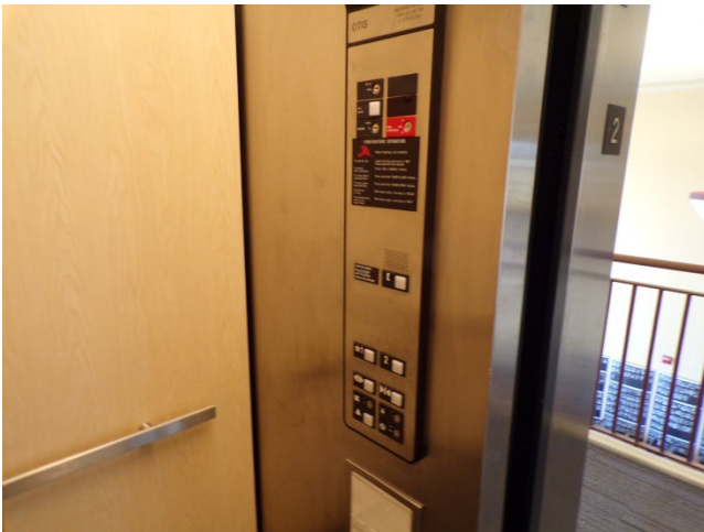
69. Gym: The elevator generally appears to meet Accessibility requirements.
