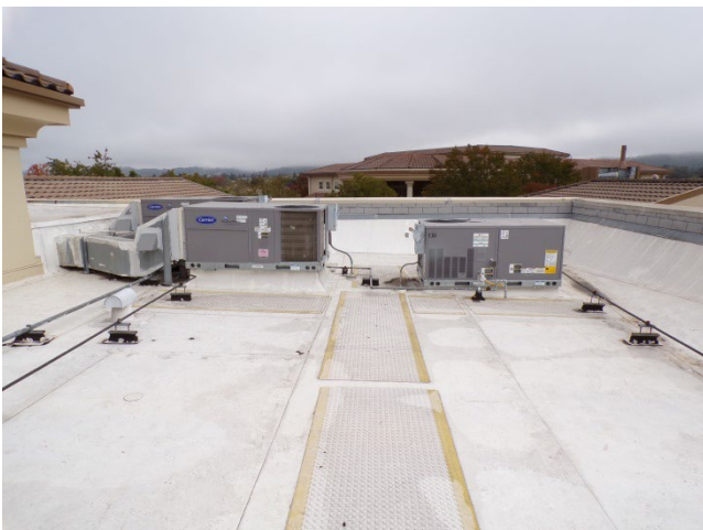
35. Main Bldg: Northeast wing TPO roof looking northeast.
