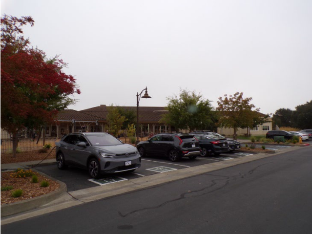
79. Four EV charging stalls are provided on the west side of the Main Bldg.
