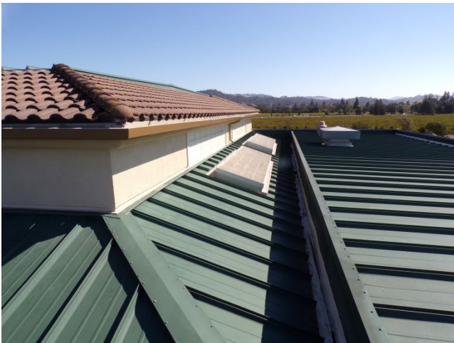
39. Gym: Standing seam metal roof with raised basketball court roof to left, looking south. Clerestory windows with translucent fiberglass panels shown.
