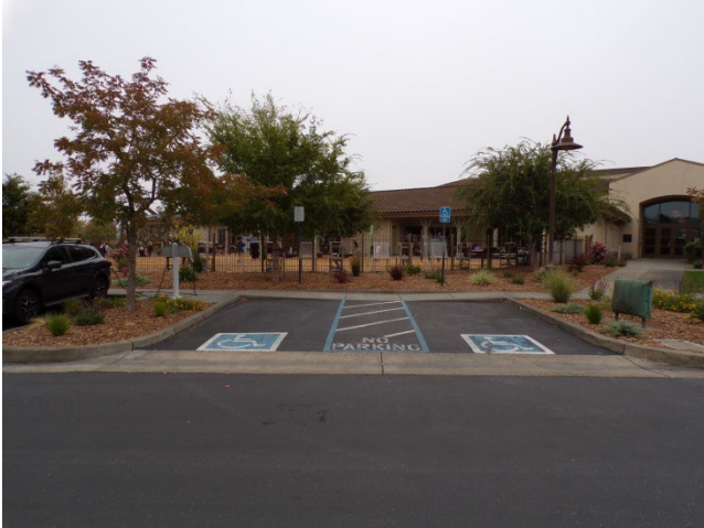
67. Accessible parking lacking correct signage; the fine amount sign is absent. Signage is typically in a degraded condition.
