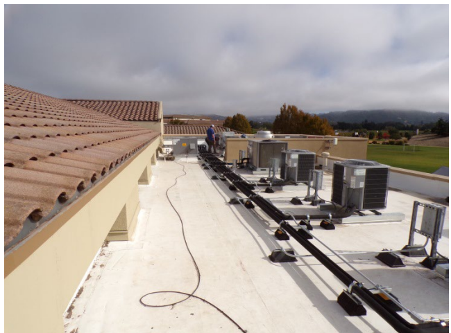
36. Main Bldg: Southeast TPO roof looking northeast.
