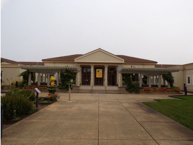
1. Main Bldg: Main entrance, terraces and stairs along south elevation.
