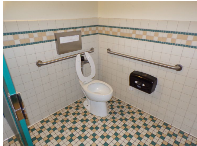
64. Gym: Typical restroom finishes.
