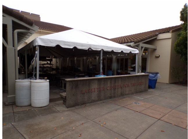
4. Main Bldg: Along north elevation. Signage for Lasseter Center for the Arts and temporary events tent shown.
