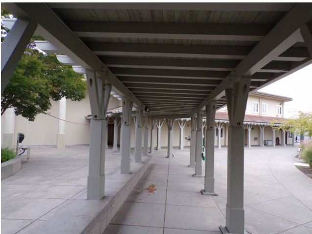
11. Covered walk connecting Main Bldg to the Gym, in background.
