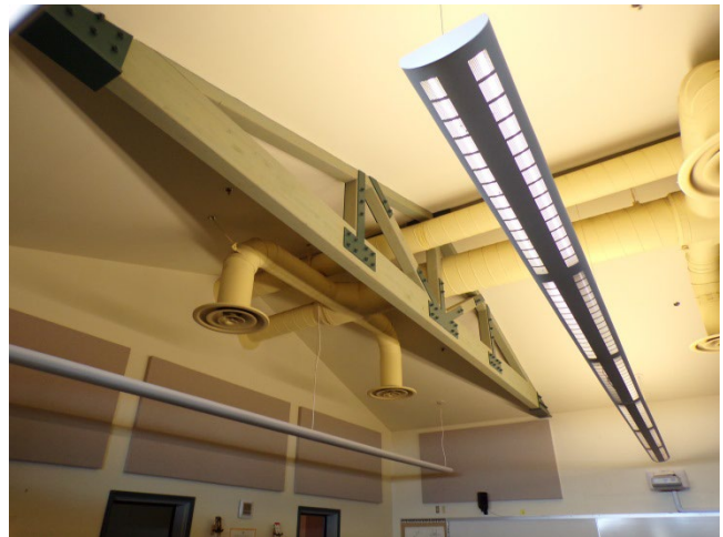
52. Main Bldg: Music classroom with exposed wood truss roof structure.
