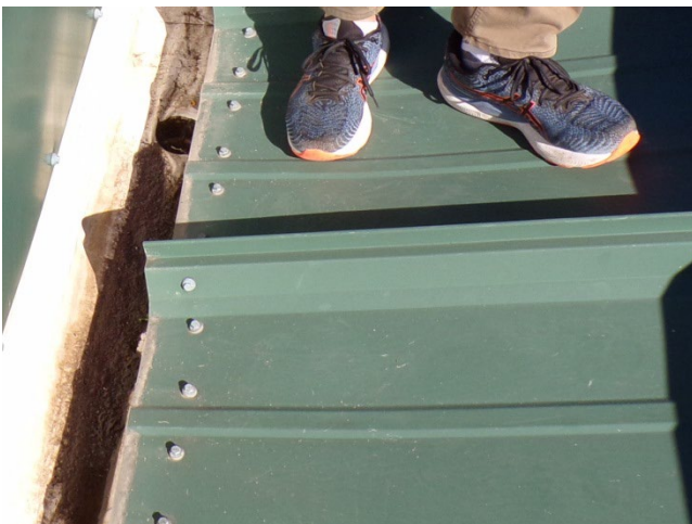
41. Gym standing seam metal roof showing TPO lined interior gutter, at left.
