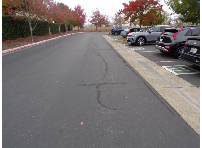
80. Minor repairs to asphalt paving can be anticipated during the reserve term.
