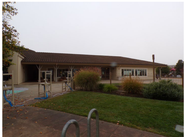
6. Main Bldg: Portion of north elevation at northwest corner of building.
