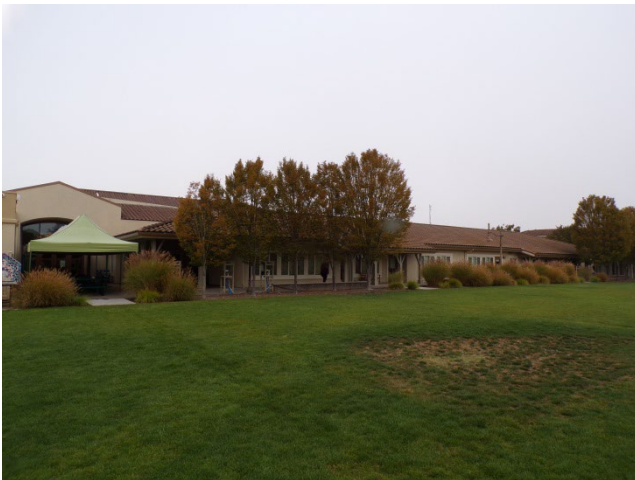
3. Main Bldg: East elevation.
