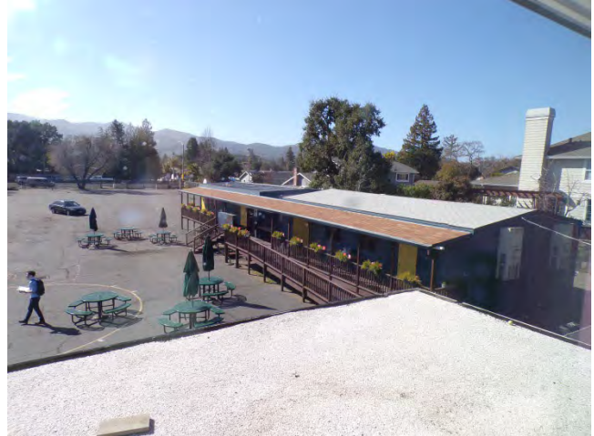
14. Mod Bldg N has an asphalt composite roofing system. Mod Bldg S has a ribbed steel panel roofing system.
