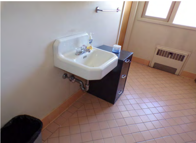
87. Rectory: Finishes and fixtures in restroom.
