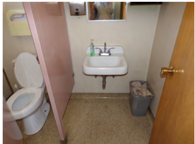
72. Church: Finishes and fixtures in older restroom.
