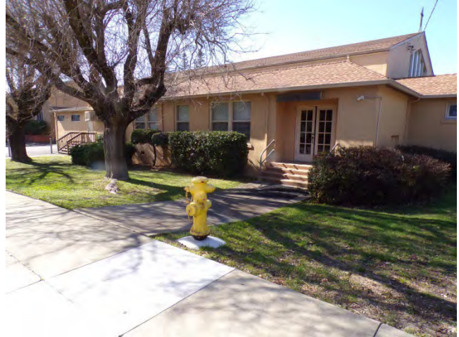
8. Hall Bldg: East elevation along Grant Avenue.
