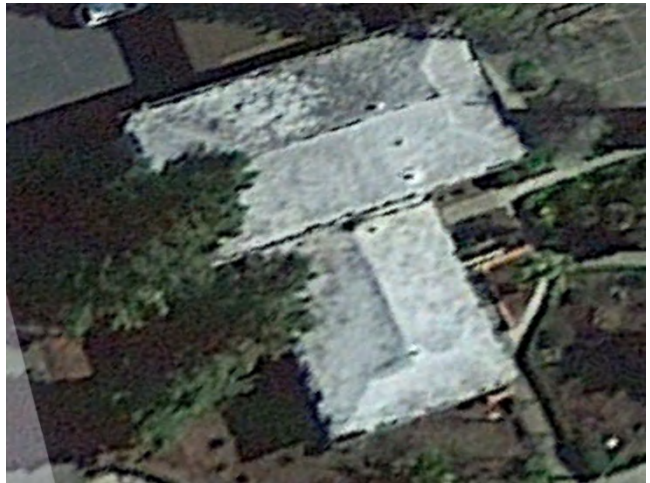
34. Rectory: A modified bitumen roofing system with white gravel ballast is installed.
