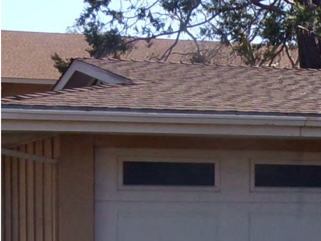
37. Garage: An asphalt composite roofing system is installed.
