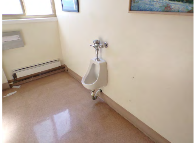
86. Rectory: Finishes and fixtures in restroom.
