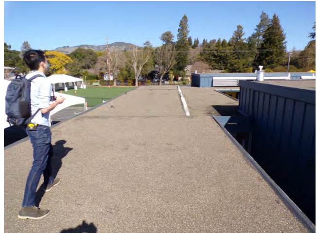
40. School: A modified bitumen roofing system with pea gravel ballast is installed.
