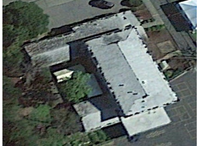
38. Convent: A modified bitumen roofing system with white gravel ballast is installed.
