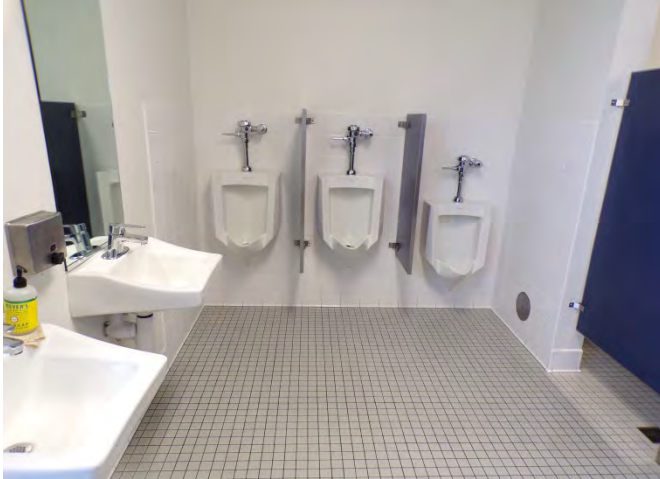
79. Hall Bldg: Finishes and fixtures in remodeled restroom.
