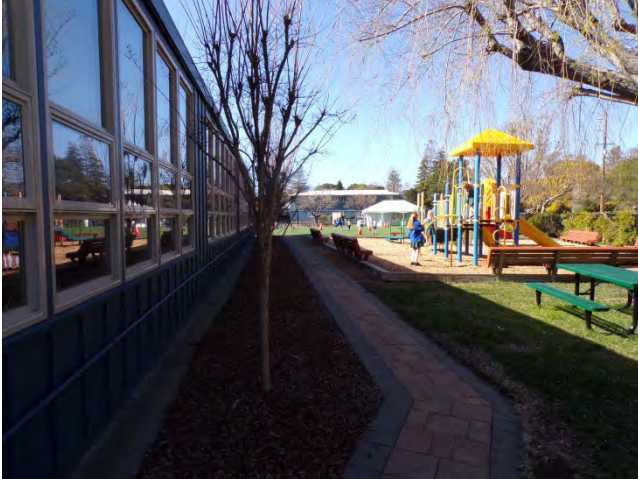
25. Playground equipment is installed along the north elevation of the School.
