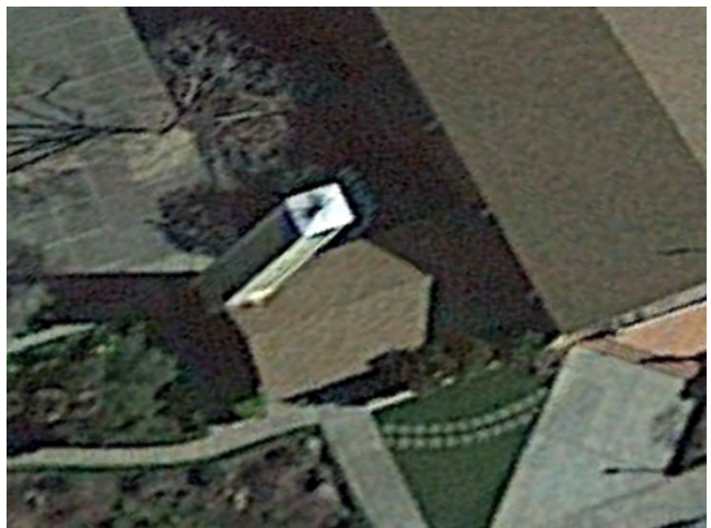
36. Bell Tower: The roofing system was not visible from grade. An unknown type of roofing system is installed.
