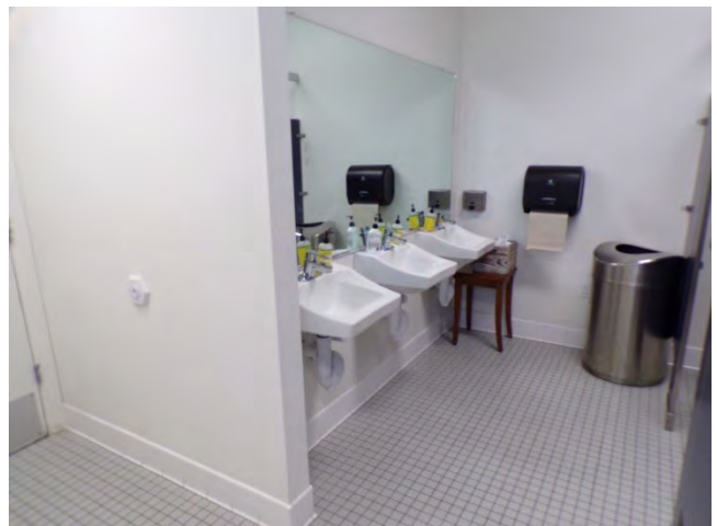
78. Hall Bldg: Finishes and fixtures in remodeled restroom.
