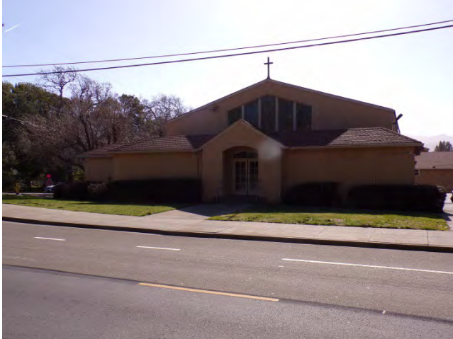
7. Hall Bldg: North elevation along Virginia Avenue.
