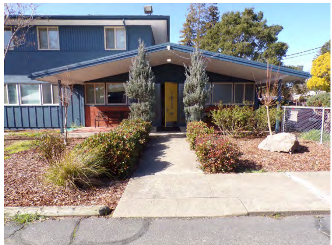
12. Convent: The primary entrance is on the east elevation.
