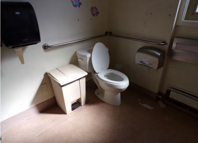
85. Rectory: Finishes and fixtures in restroom.
