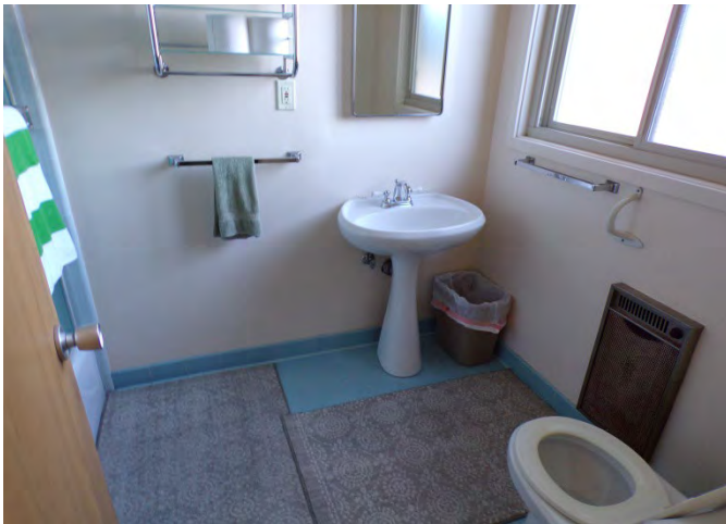
75. Rectory: Finishes and fixtures in residential unit bathroom.
