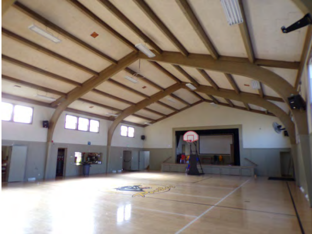
55. Hall Bldg: Interior finishes and fixtures in basketball court.
