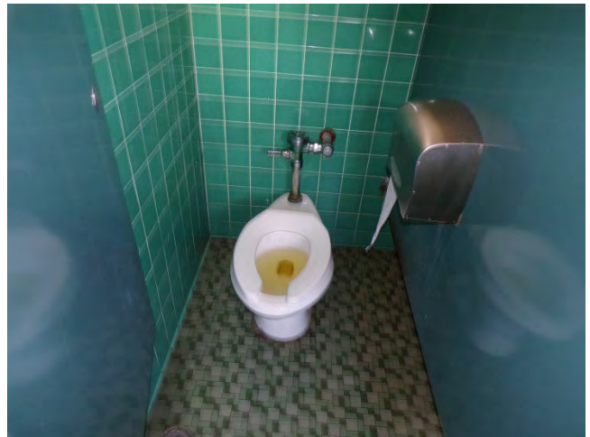
82. School: Finishes and fixtures in children's restroom.
