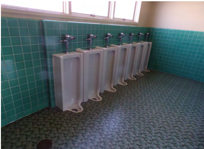
81. School: Finishes and fixtures in children's restroom.
