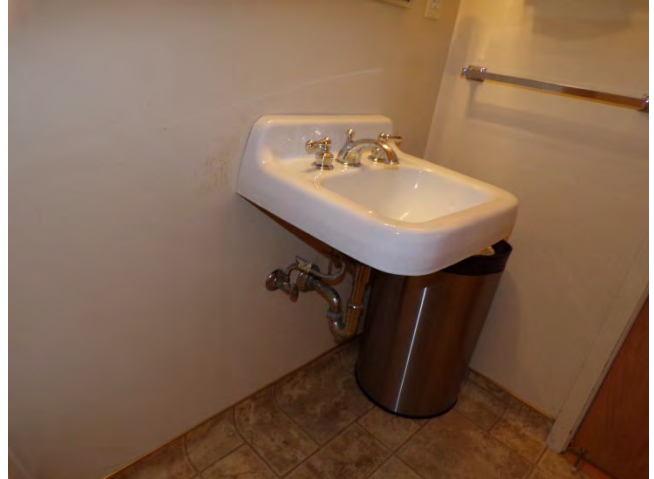
74. Rectory: Finishes and fixtures in office area restroom.
