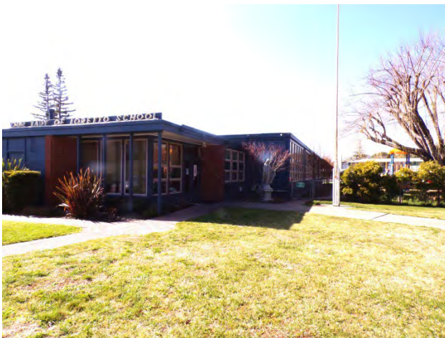
9. School: Primary entrance at center of photo. North elevation at right-center.
