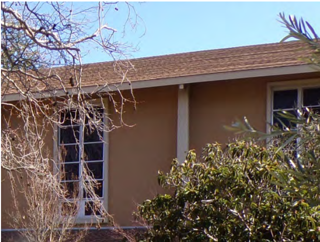
33. Church: An asphalt composite roofing system is installed.
