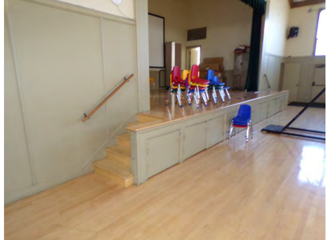
56. Hall Bldg: Interior finishes and fixtures at stage area.
