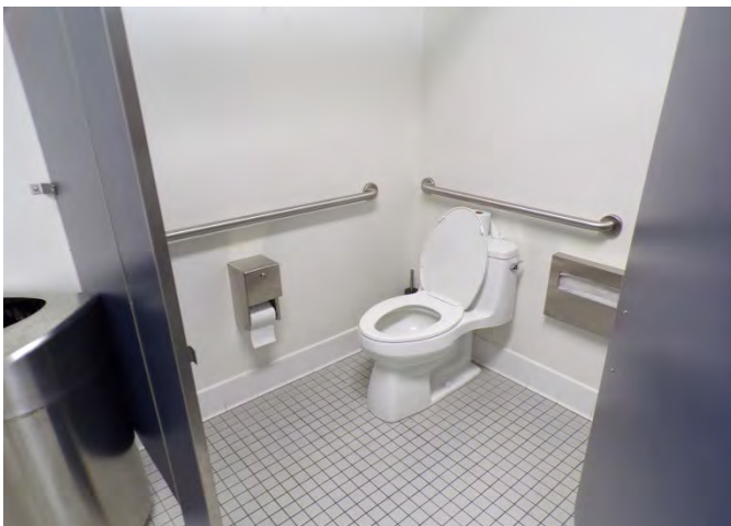
77. Hall Bldg: Finishes and fixtures in remodeled restroom.
