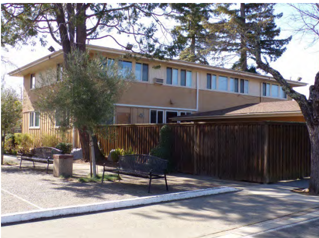
5. Rectory: Portion of west elevation at center; north elevation at far left. The roof of the Garage is at right.
