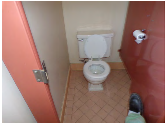
88. Rectory: Finishes and fixtures in restroom.
