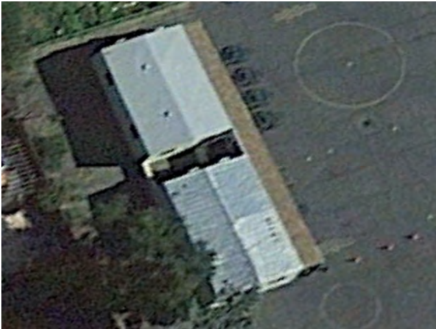
39. Mod Bldg N (at top) has an asphalt composite roofing system. Mod Bldg S (at bottom) has a ribbed steel panel roofing system.
