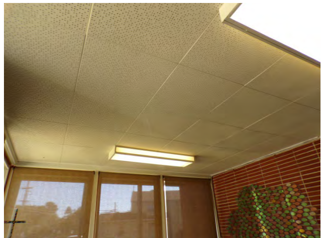
60. School: Interior finishes and fixtures in office area. Adhesive-applied acoustic ceiling tiles shown.
