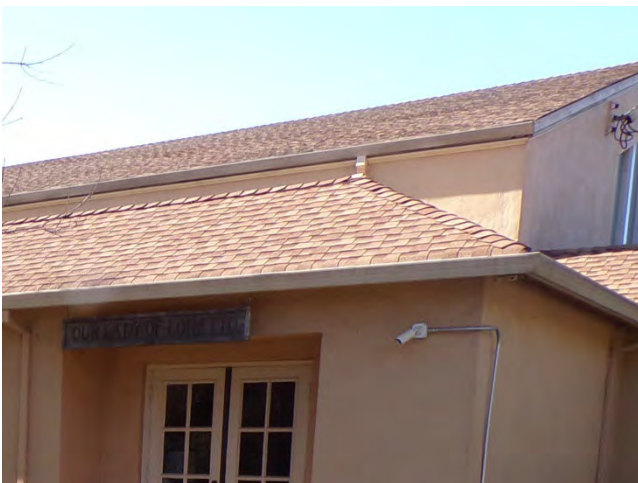
35. Hall Bldg: An asphalt composite roofing system is installed.
