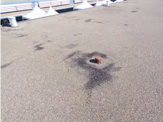
43. School: Atrium grated roof drains are installed.
