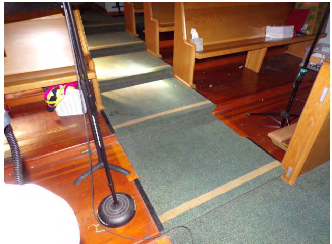
48. Church: Interior finishes and fixtures in choir loft
