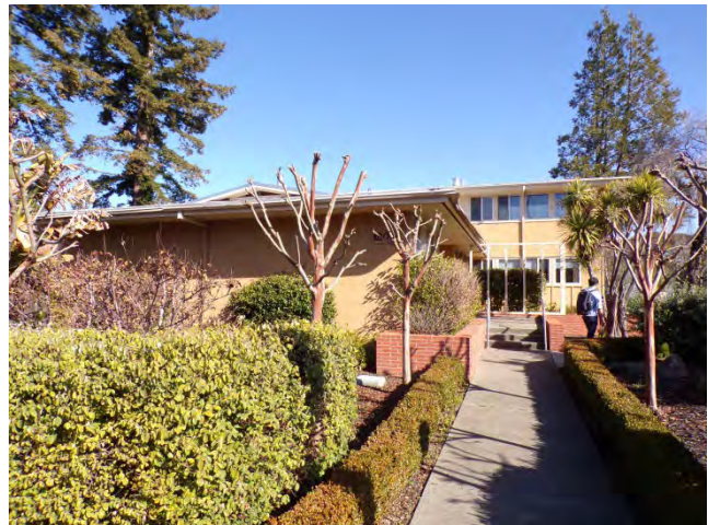
4. Rectory: South elevation.
