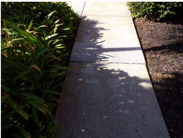
23. Evidence of concrete grinding was observed.
