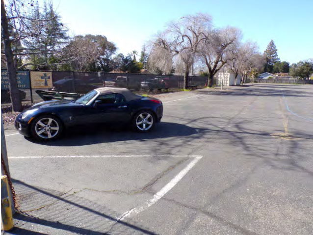
31. Parking stall striping is in an overall degraded condition.
