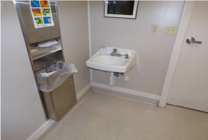
25. Interior finishes and fixtures in Accessible restroom.
