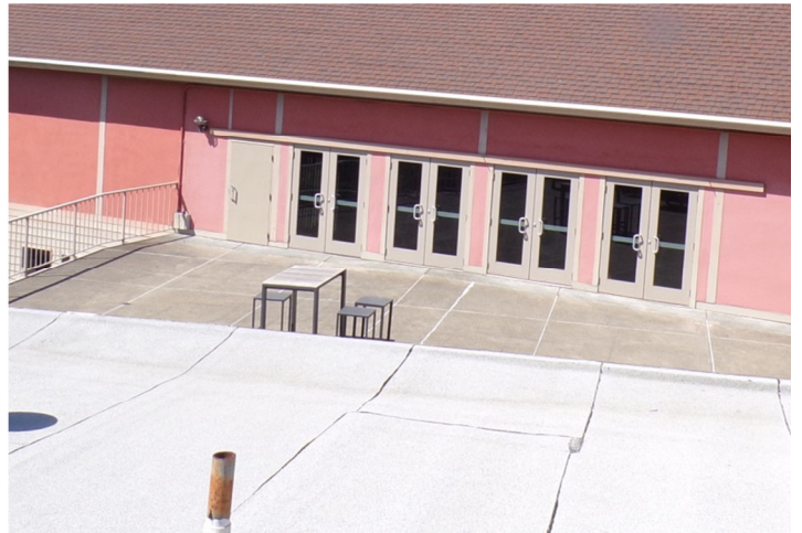
52. A concrete deck is provided on east side of the Sanctuary.
