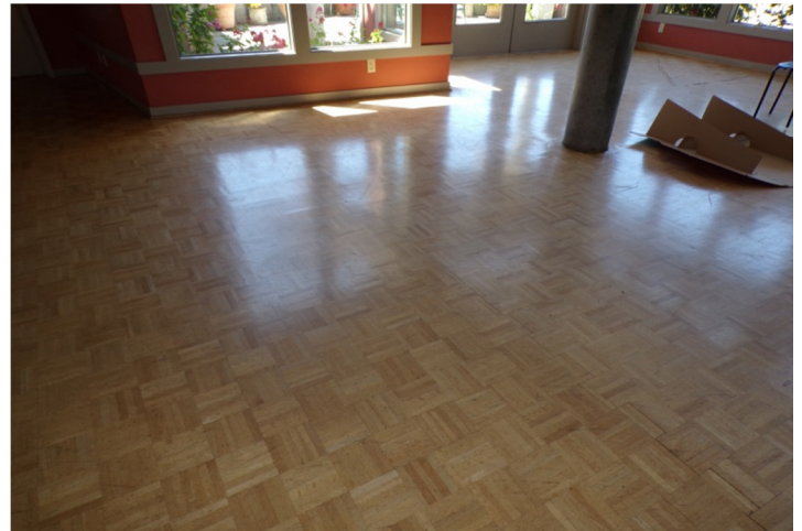
28. Interior finishes on main level with parquet wood flooring shown.
