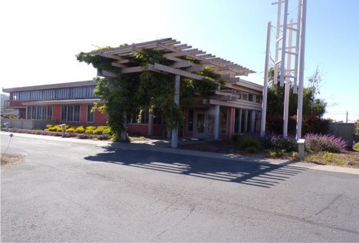
1. North elevation and main entrance, looking southeast.
