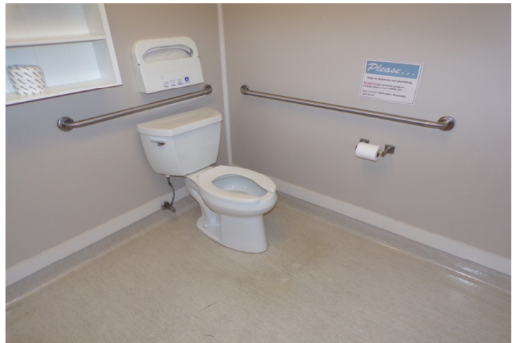
24. Interior finishes and fixtures in Accessible restroom.
