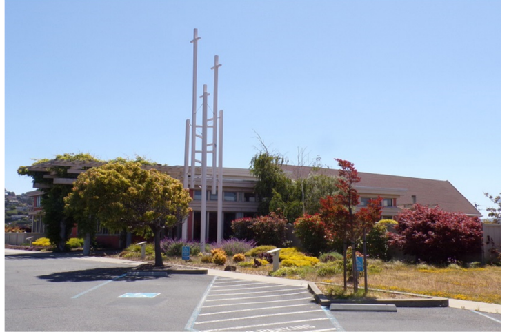
2. North portion of west elevation, looking east.
