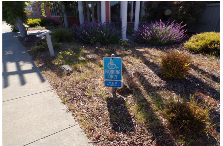
64. Accessible parking signage no longer complies with current Accessibility codes.
