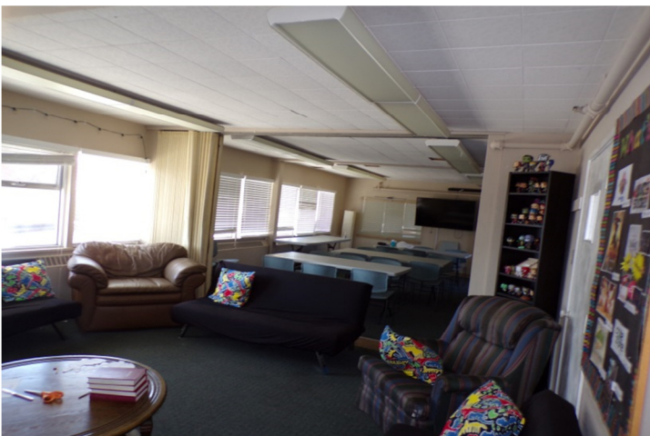
29. Typical interior finishes and fixtures in upper level classroom.
