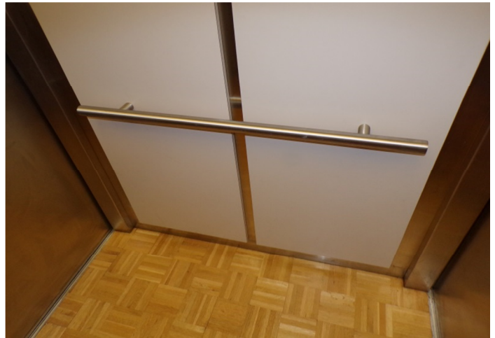
82. Interior finishes in the elevator cab with grab bar shown.
