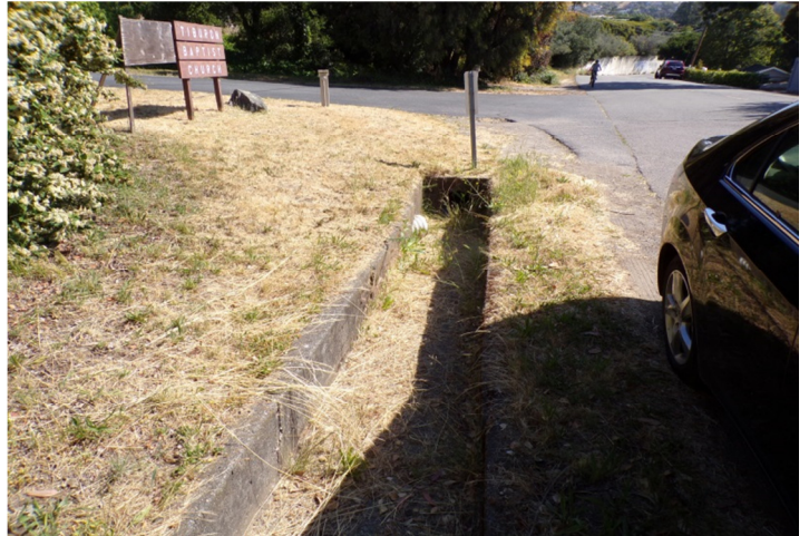
14. Typical untended landscaping along Greenwood Beach Road at south side of site with concrete swale shown. East site entrance in background.
