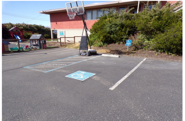
10. Single Accessible parking stall along east elevation.
