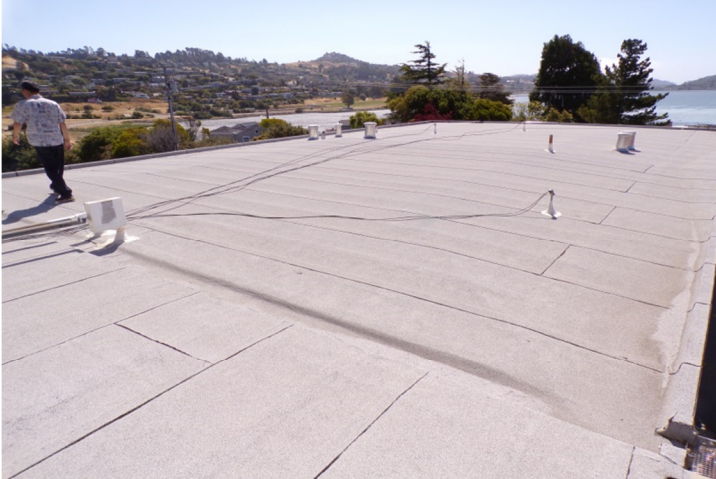
37. Roof above main floor level, looking south toward southeast corner of the building.
