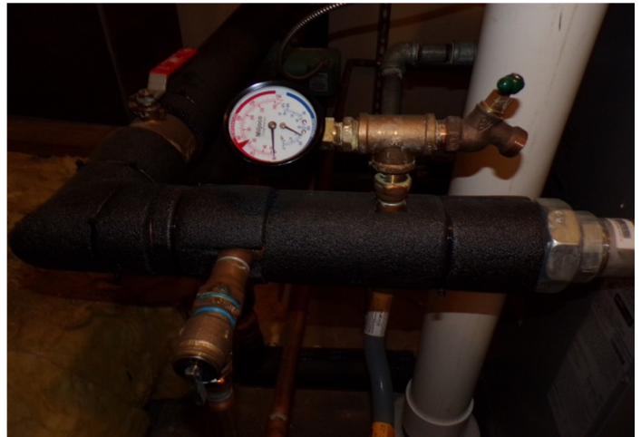
88. The boiler is fitted with a rigid gas line connection.
