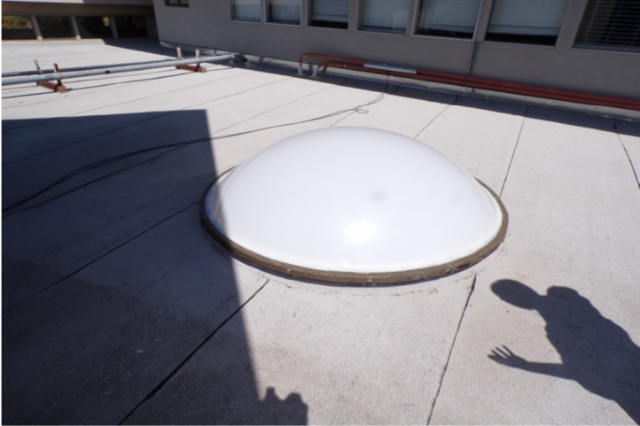
43. In September 2017, a new circular domed skylight was installed on the roof above the main floor.
