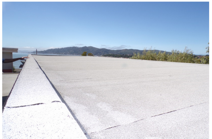
42. Roof above main floor level with new BUR system, looking south-southwest.
