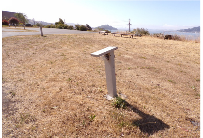
92. Some wooden pedestals for exterior lighting are out-of-plumb.
