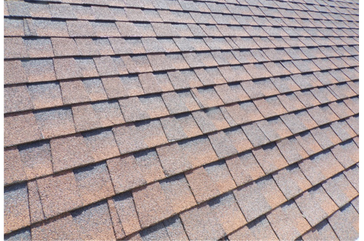
50. The shingles above the Sanctuary are in better condition than those on the lower-sloped pitched roofs.
