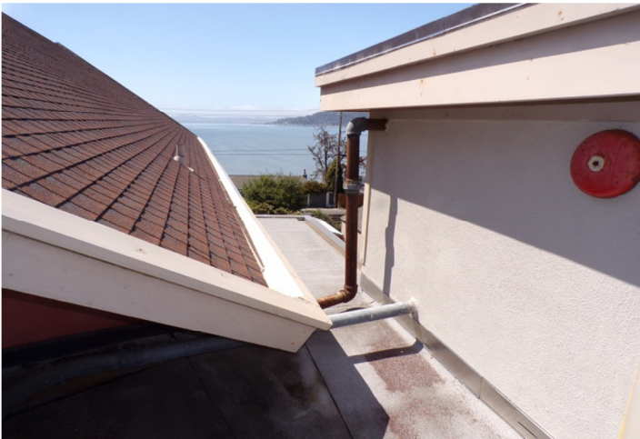
51. The asphalt composite shingles above the Sanctuary may have an EUL which extends beyond the 10-year term of analysis.
