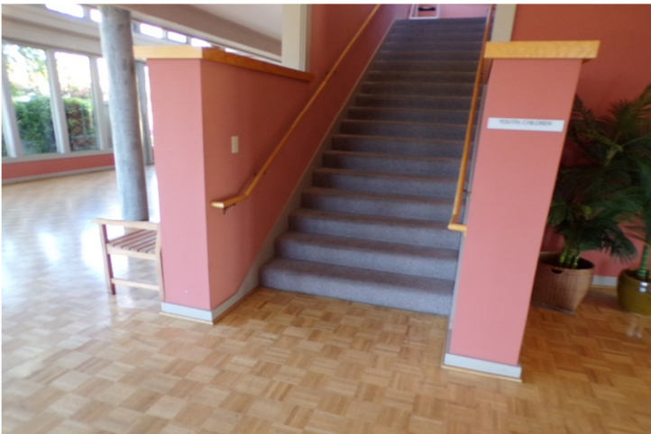
23. Interior finishes at the stairs adjacent to entrance foyer.
