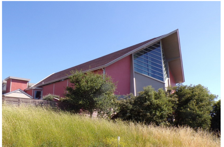
4. South elevation at Sanctuary (at right), looking northeast. South portion of west elevation at left.
