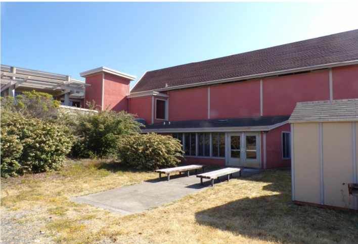
3. South portion of west elevation, looking northeast.
