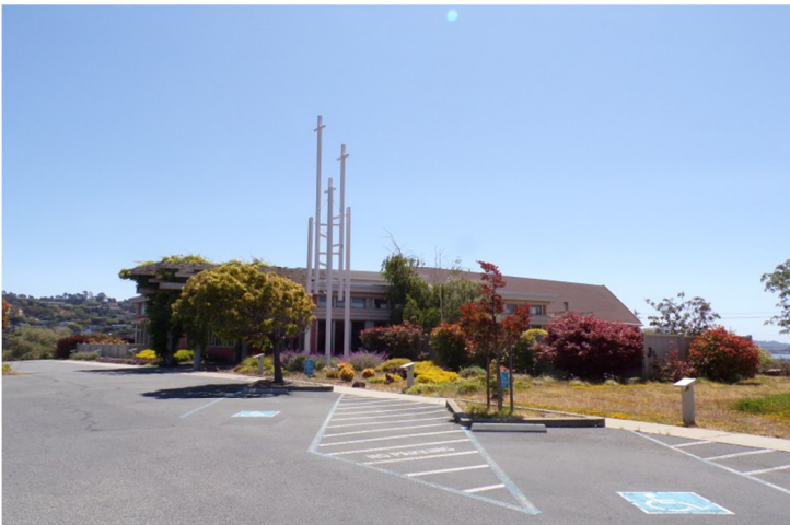
65. Truncated domes are not installed in any required location at the subject property.
