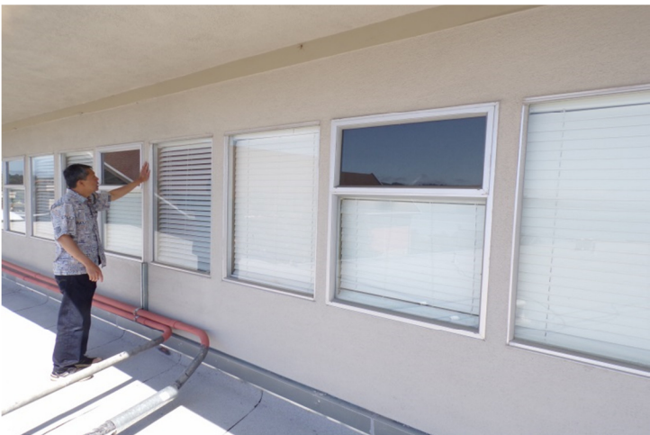
59. Some exterior elements on the upper level were relatively recently repainted (2020 reported).
