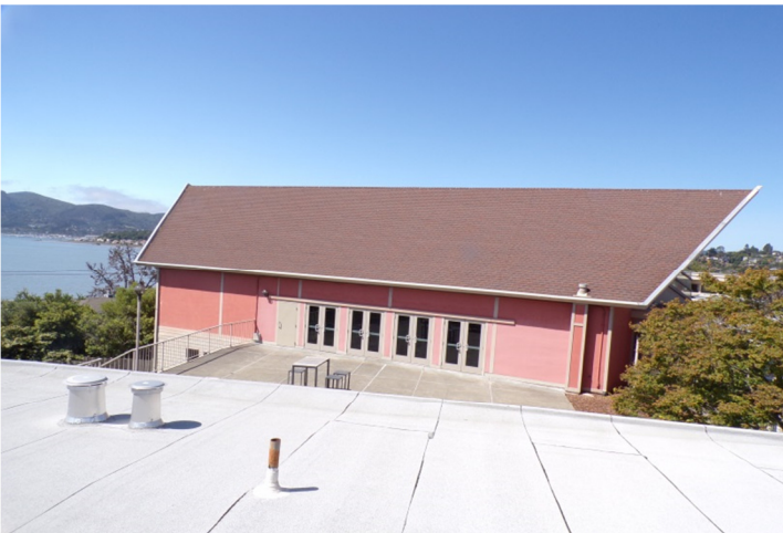
5. East elevation of the Sanctuary, looking west-southwest.
