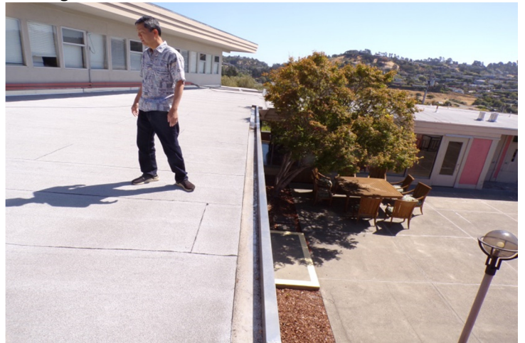
40. Roof above main floor level, looking east. New flashings were installed along with the BUR systems.
