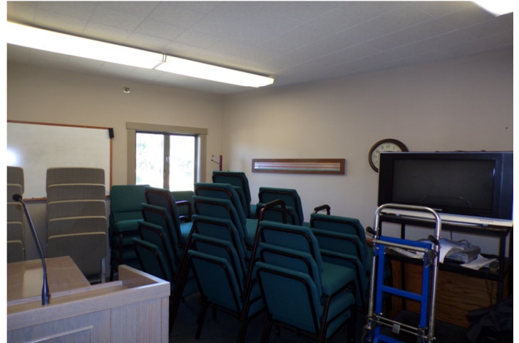
26. Typical interior finishes and fixtures in classroom.
