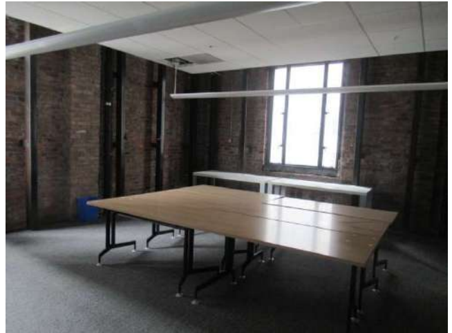
28. Typical seismic bracing at the exterior brick walls.
