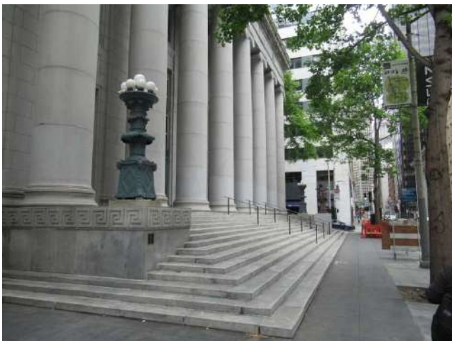
5. Grand staircase serving the Sansome Street entrance.
