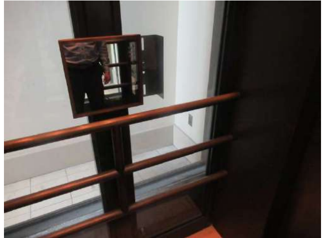
56. Elevator is provided with transparent cab walls.
