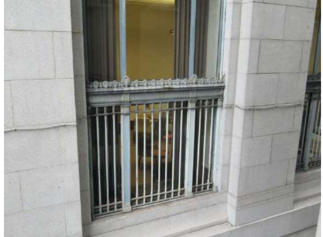
20. Typical window at the first floor with vertical bars at the bottom.
