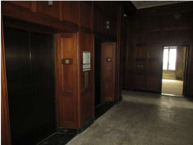
51. Historical interiors at the second floor elevator lobby.
