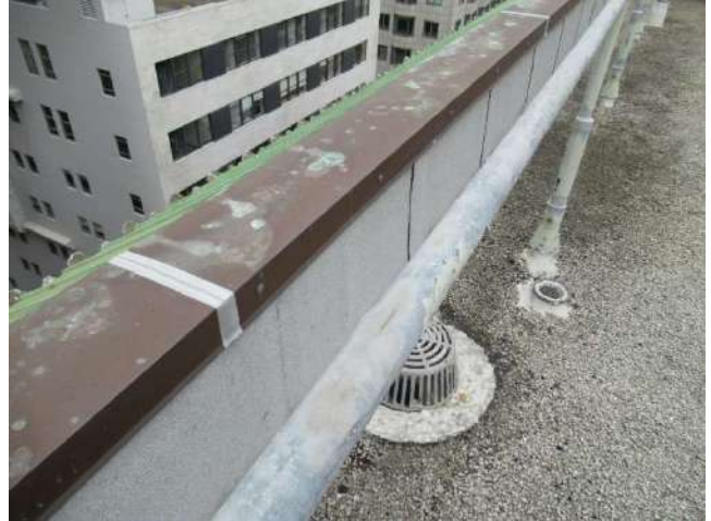
14. Typical roof drain configuration.
