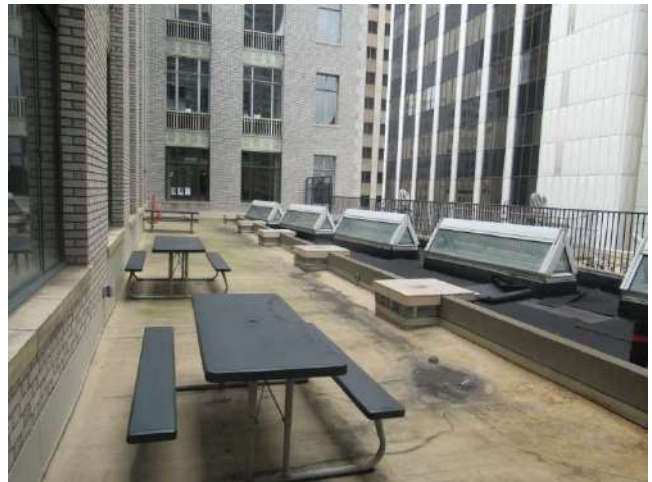
10. Fourth floor terrace is constructed with a cast-in-place concrete slab over a waterproof membrane. The row of triangular skylights was apparently installed after 2019.
