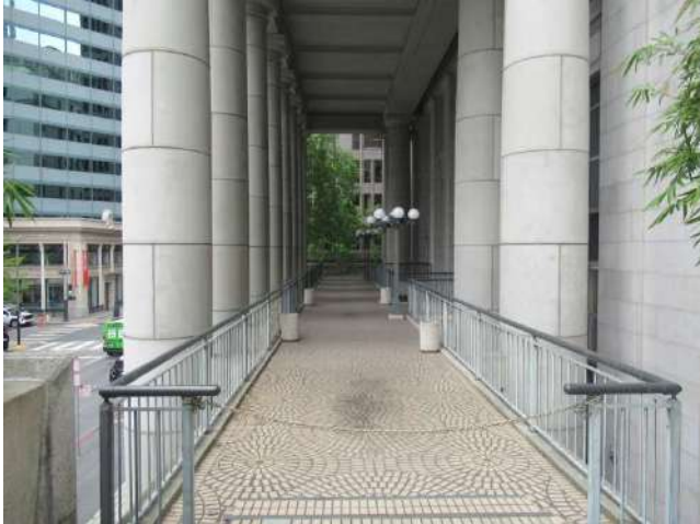
7. Balcony from elevated walkway above the Battery Street entrance.
