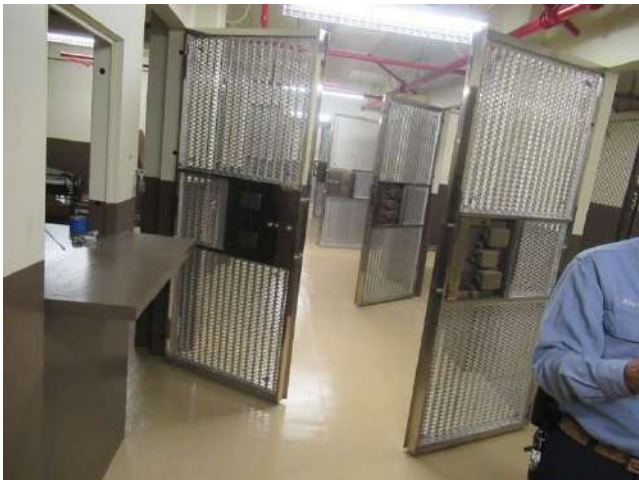
53. Vault space at basement level.
