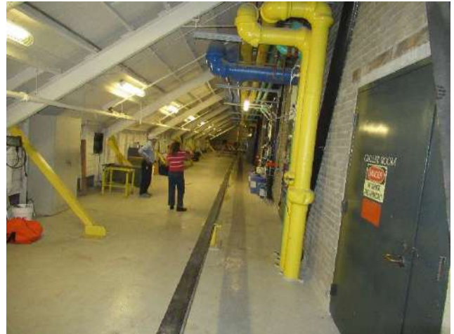
76. In the interior spaces beneath the copper roof areas, the steel rail running through the center of the shot is used for window washing equipment anchoring.
