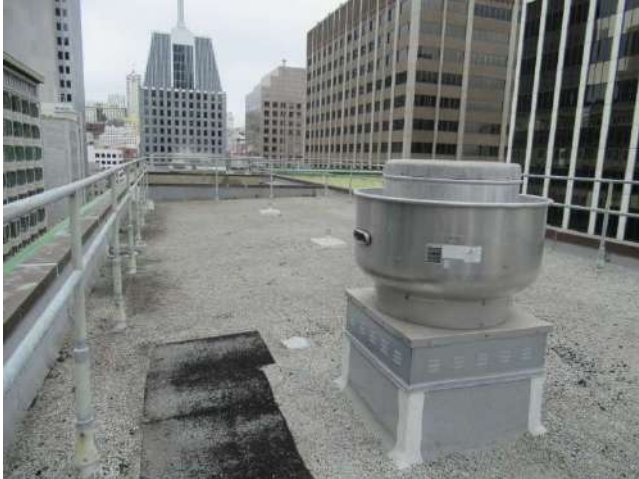
13. Built-up roofing system at top roof.
