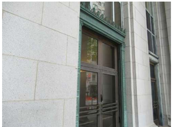
24. Copper and bronze entrance along Sansome Street.
