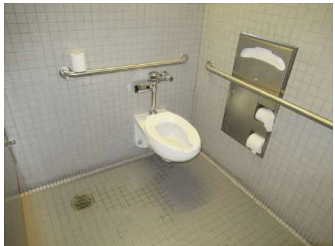
42. Typical Accessible restroom stall.
