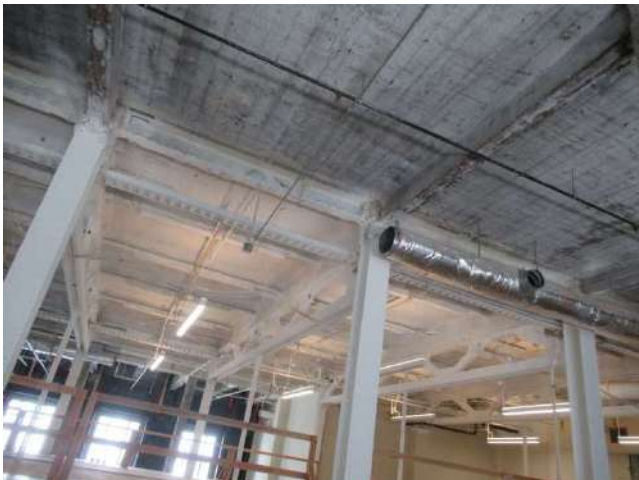
29. Steel trusses above the banking hall roof support the floors above.
