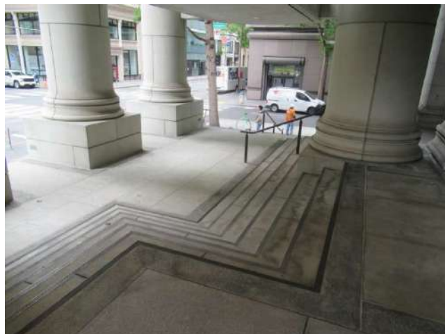
6. Staircase serving the Battery Street entrance.
