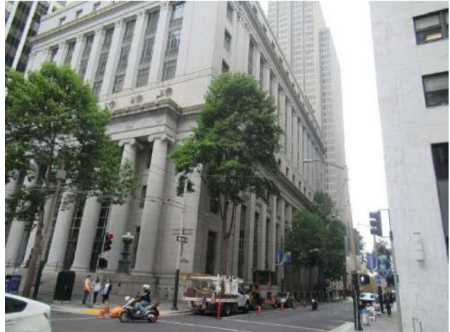
2. South elevation facing Sacramento Street, at right.
