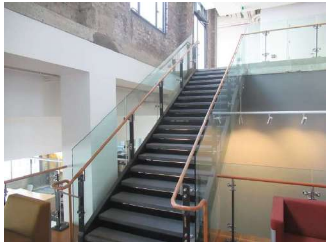
40. Stairs connecting levels six and seven.
