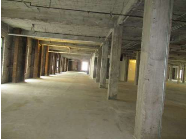
25. All partition walls on the third floor have been removed.
