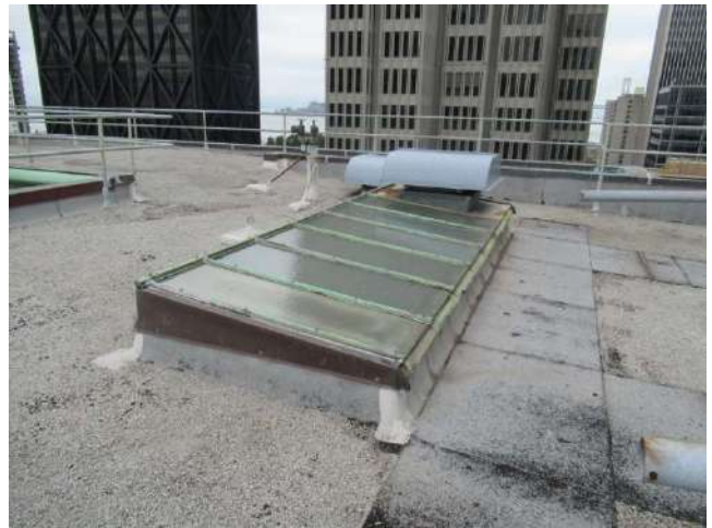
16. Typical roof-mounted skylight.
