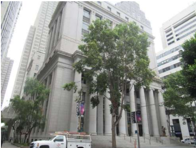
3. West elevation facing Sansome Street.
