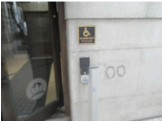
59. Accessible entrance at Commercial Street is provided with an intercom and power door assist equipment. The vertical bar door assist has been installed since 2019, as required by code.
