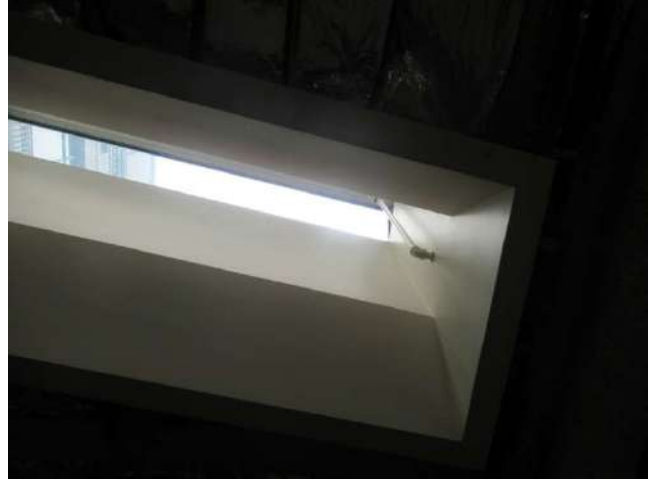
26. Looking up into one of the five skylights that illuminate the third floor.
