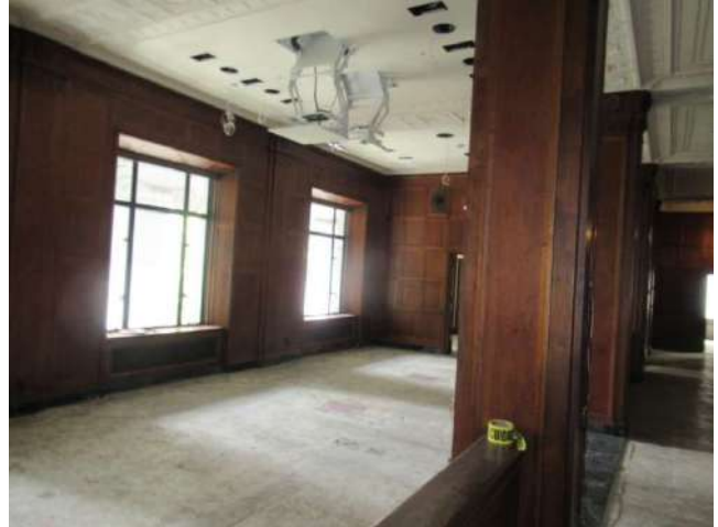
50. Historical interiors at a second floor conference room.
