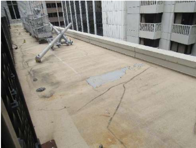
75. Swing stage, booms, and window washing equipment attachment points on 4 th floor roof.
