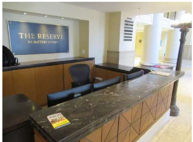
60. The main lobby reception desk includes a lower surface at Accessible height.
