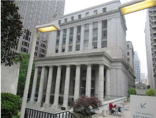
1. East elevation facing Battery Street.
