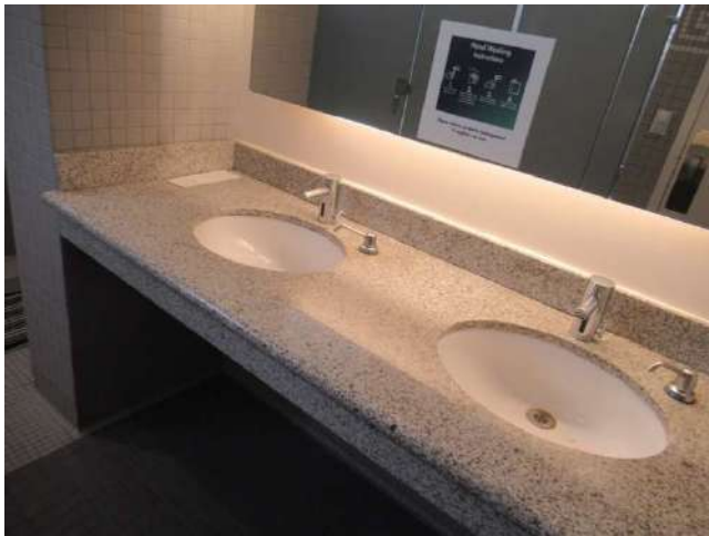
45. Restroom adjacent to locker room.
