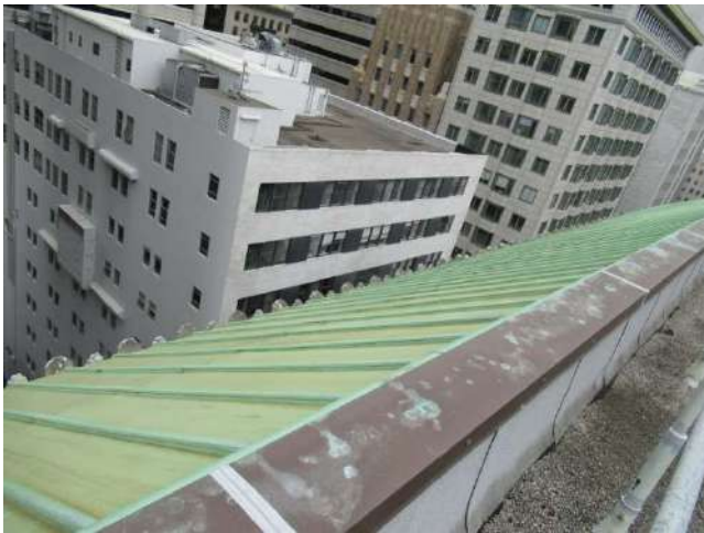
15. Sloped copper roofing systems are provided.
